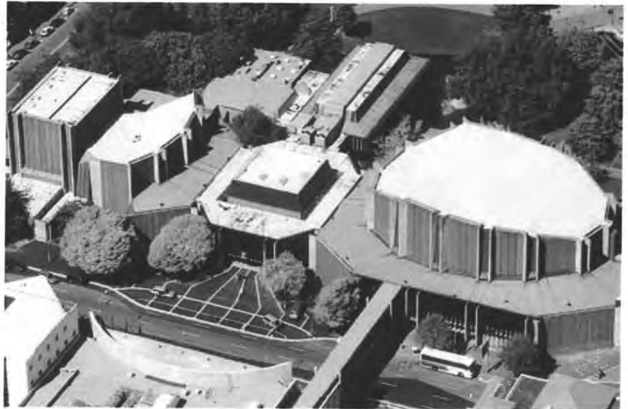
Current View of Christchurch Town Hall. 1 mm Butynol® Roof Membrane laid 1972.
