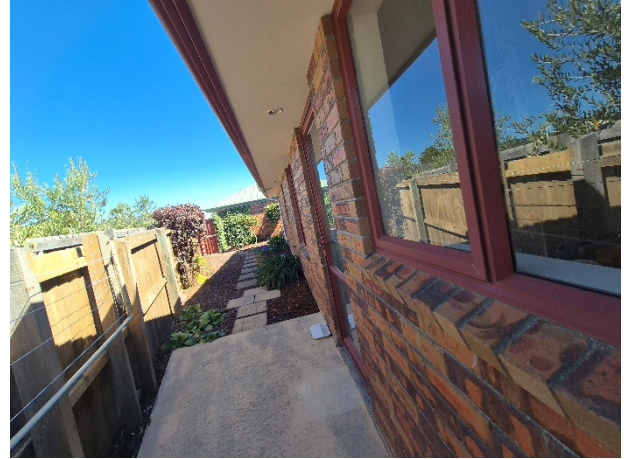
Photo 2. View of exterior.
