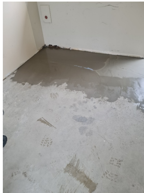
Photo 6. View of floor levelling compound (Received pics)
