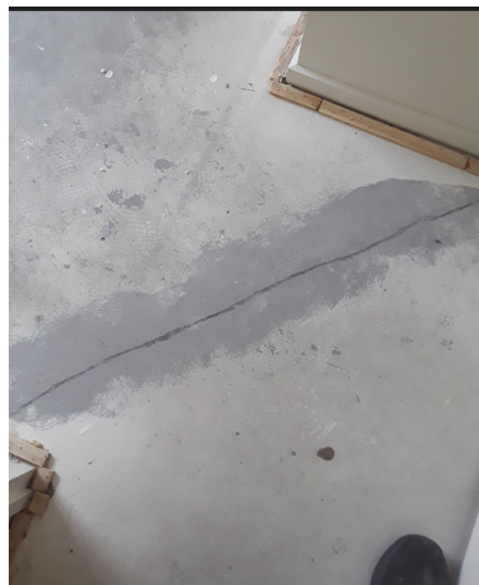
Concrete slab crack repairs 2( received)
