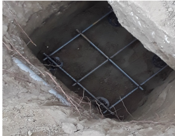
Photo 4. View of pre-pour underpinning-pad hole (Received pics)
