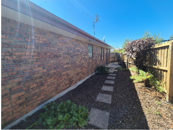
Photo 1. View of exterior.
