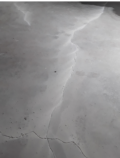
Concrete slab crack repairs 1( received)
