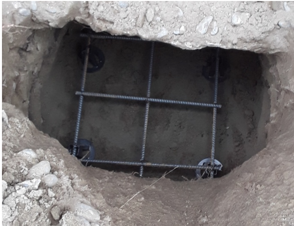
Photo 3. View of pre-pour underpinning-pad holes (Received pics)
