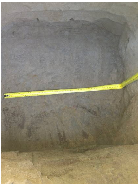
Photo 5. View of pre-pour underpinning-pad holes (Received pics).
