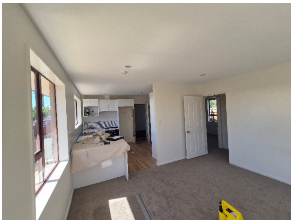
Photo 7. View of internal linings.
