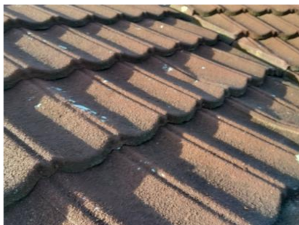
Roof – general view. Patches of coating missing
