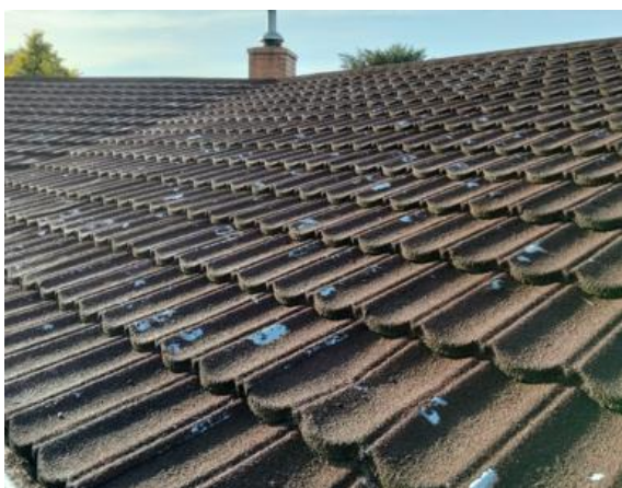
Roof – general view. Patches of coating missing
