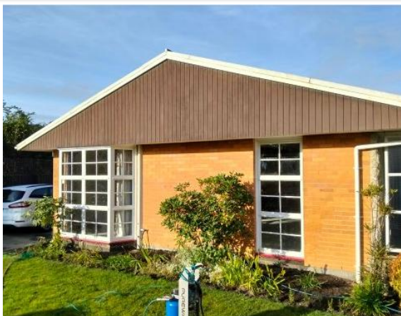
Cladding and windows – general view
