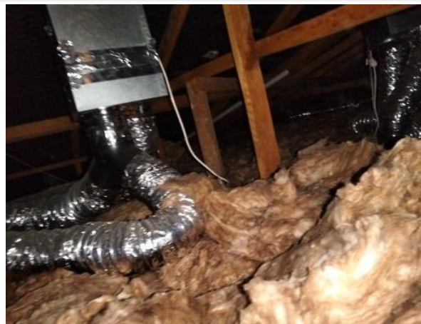
Roof space is well insulated, batts are approx. 200mm thick
