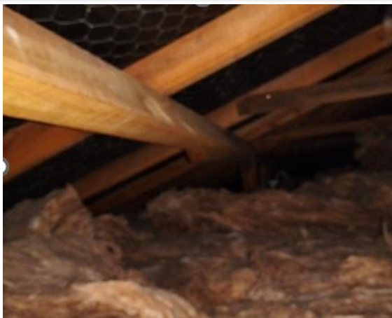
Roof space is well insulated, batts are approx. 200mm thick
