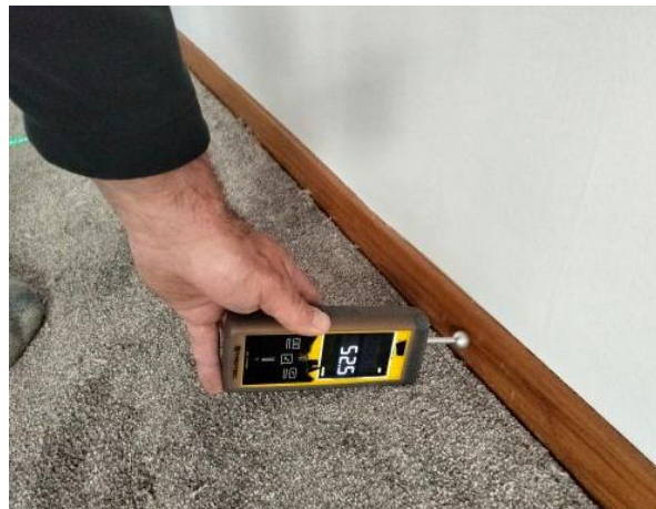
One moisture reading – slightly elevated, lounge
