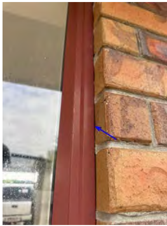
Example - where gap sealing could be carried out around joinery where it meets the cladding to improve it.
