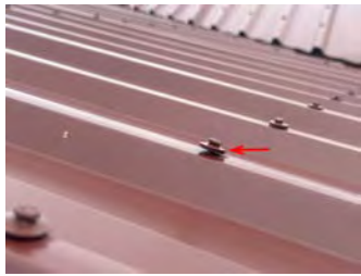
Example - popped roofing nail.
