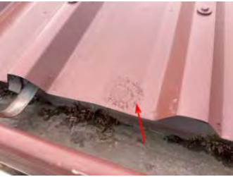
Example - there are some patches in places where the paint has been applied over residual lichen on the cladding or damaged undercoat. This may eventually cause some minor flaking in some isolated spots.
