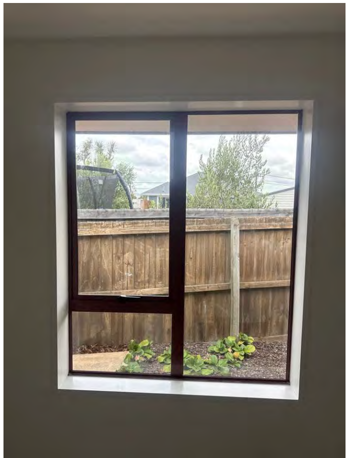
Ease window a touch so it doesn't grab the frame.
