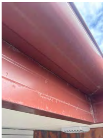
Example - typical light corrosion to fascia's throughout
