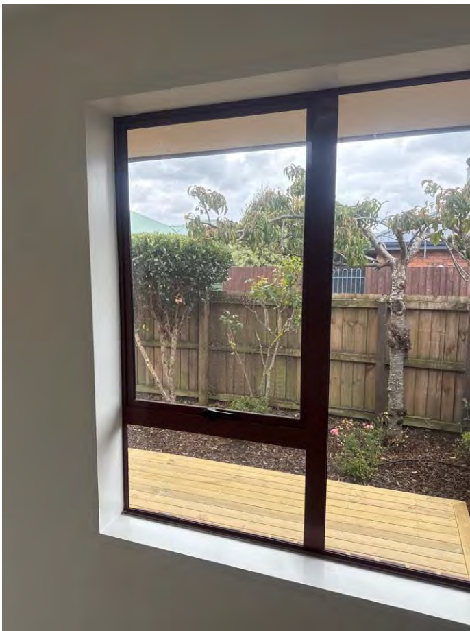
Ease window a touch so it doesn't catch the frame.
