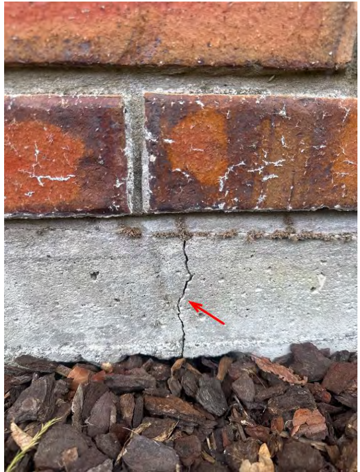
Minor crack.
