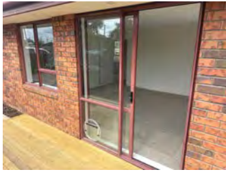
Example - where gap sealing could be carried out around joinery where it meets the cladding to improve it.
