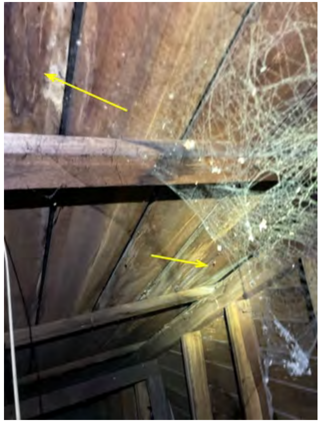
Historical signs of moisture marks on sarking. Likely from previously popped roof fixings.
