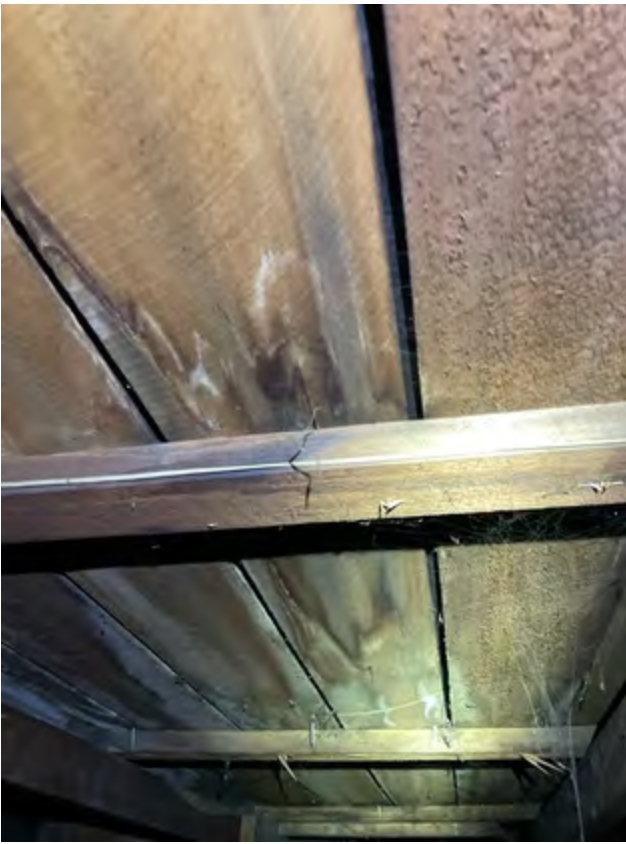
Historical signs of moisture marks on sarking. Likely from previously popped roof fixings.
