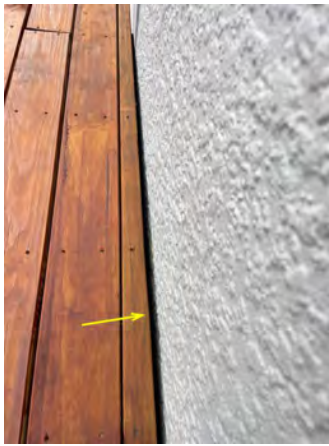
Good drainage gaps between the deck and the dwelling.
