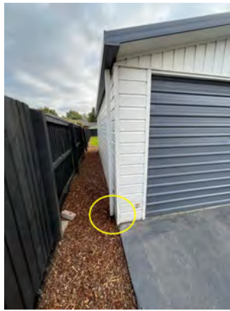
No stormwater risers noted.
