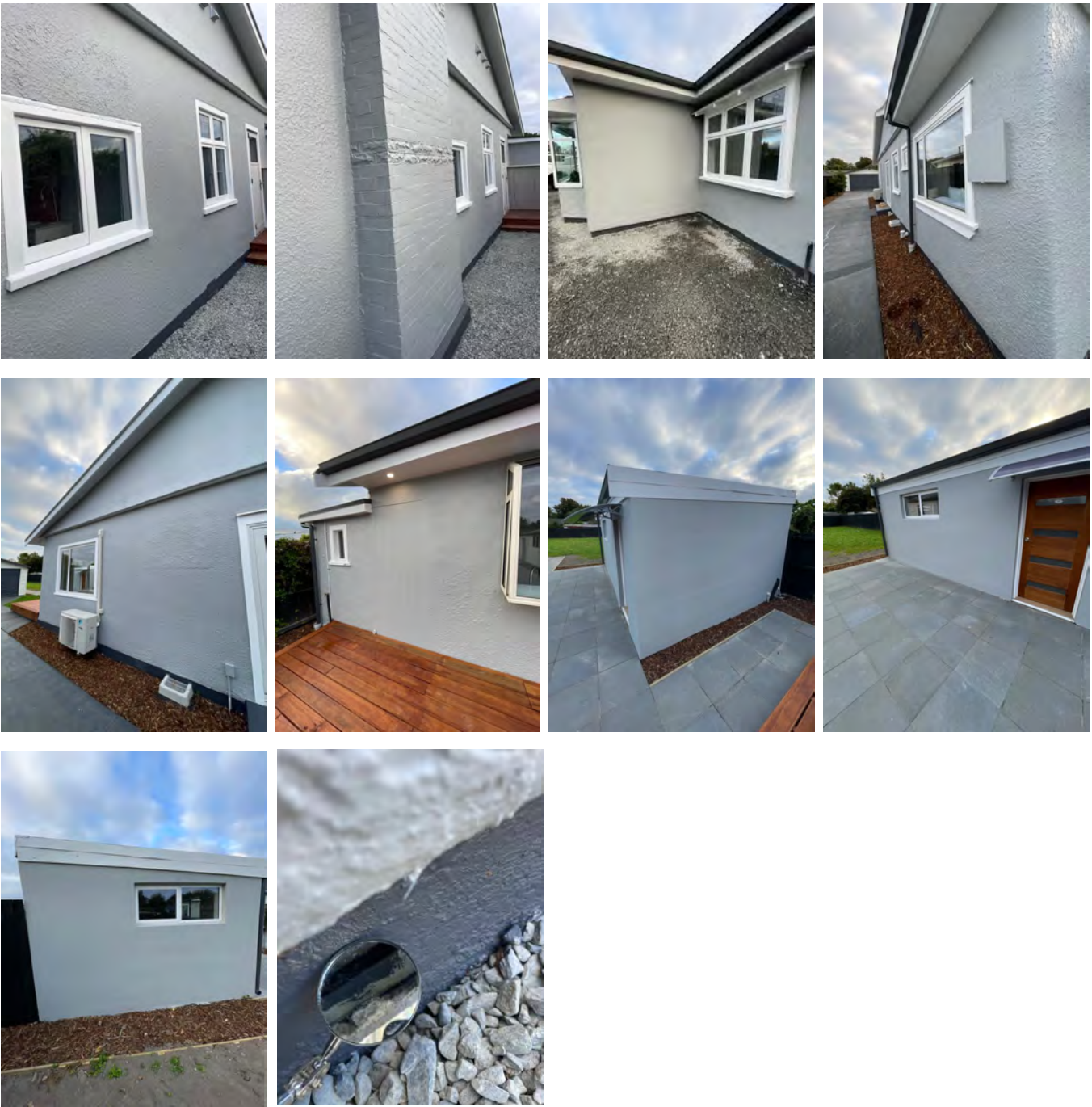
Example of what looks to be stucco over a timber weatherboard cladding system on south end of the main dwelling.
