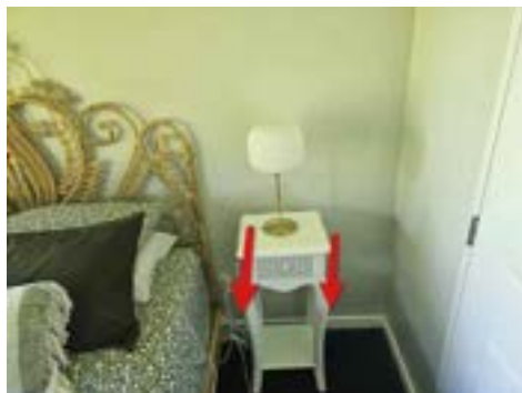
Corner Bedroom - 78.3% Elevated reading due to concrete nib wall
