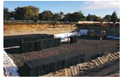
Fig. 4 Preassembled modules can be placed in the excavation or installation can be sped up by assembling the modules in the excavation.
