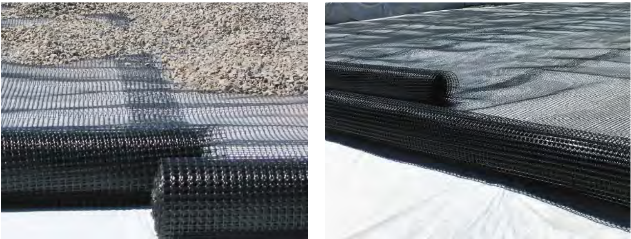
Fig. 24 Overlap geogrid 300mm or as required by plans.
