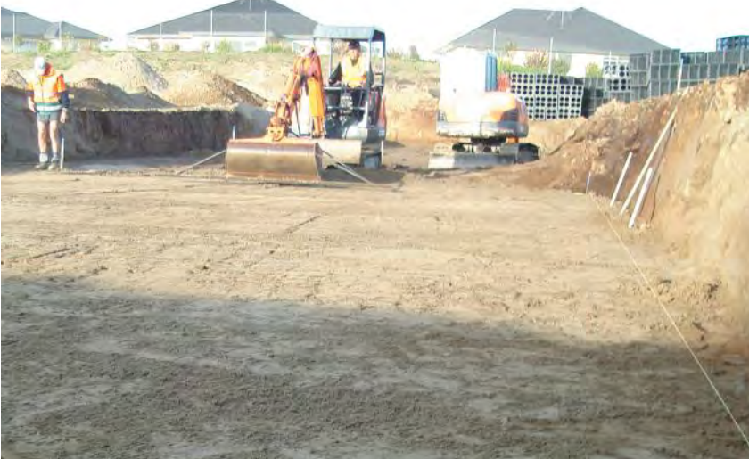
Fig. 5 Base must be smooth to ensure modules fit together without gaps.
