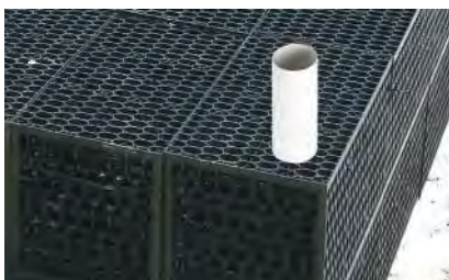
Fig. 11 Installed inspection port.
