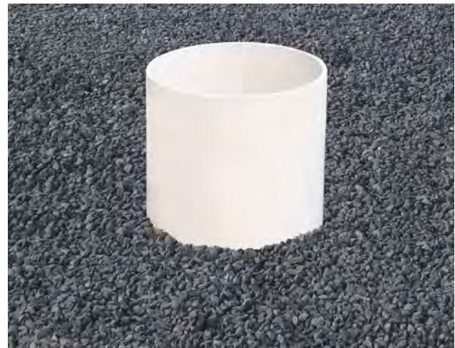
Fig. 17 Install port into RainSmart System
