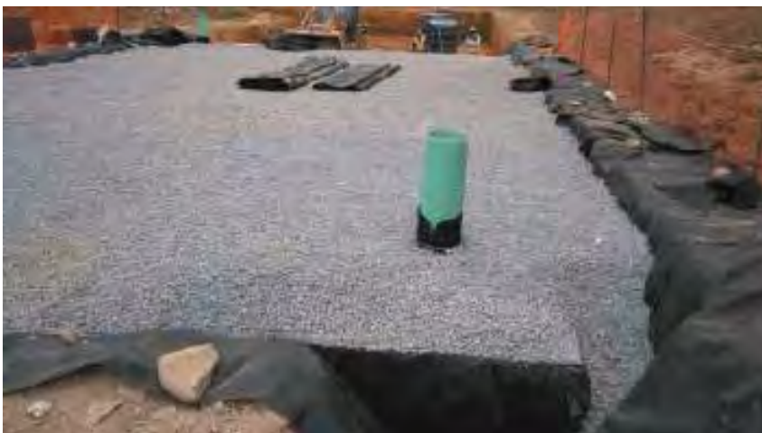
Fig. 23 Use skid-steer to place backfill over RainSmart modules.
