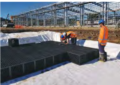
Fig. 8 Use a string line & marking paint to square the system footprint.
