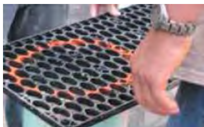
Fig. 12 Cut the horizontal plates to accommodate all ports.
