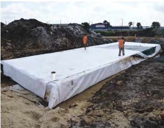
Fig. 16 Installed maintenance port
