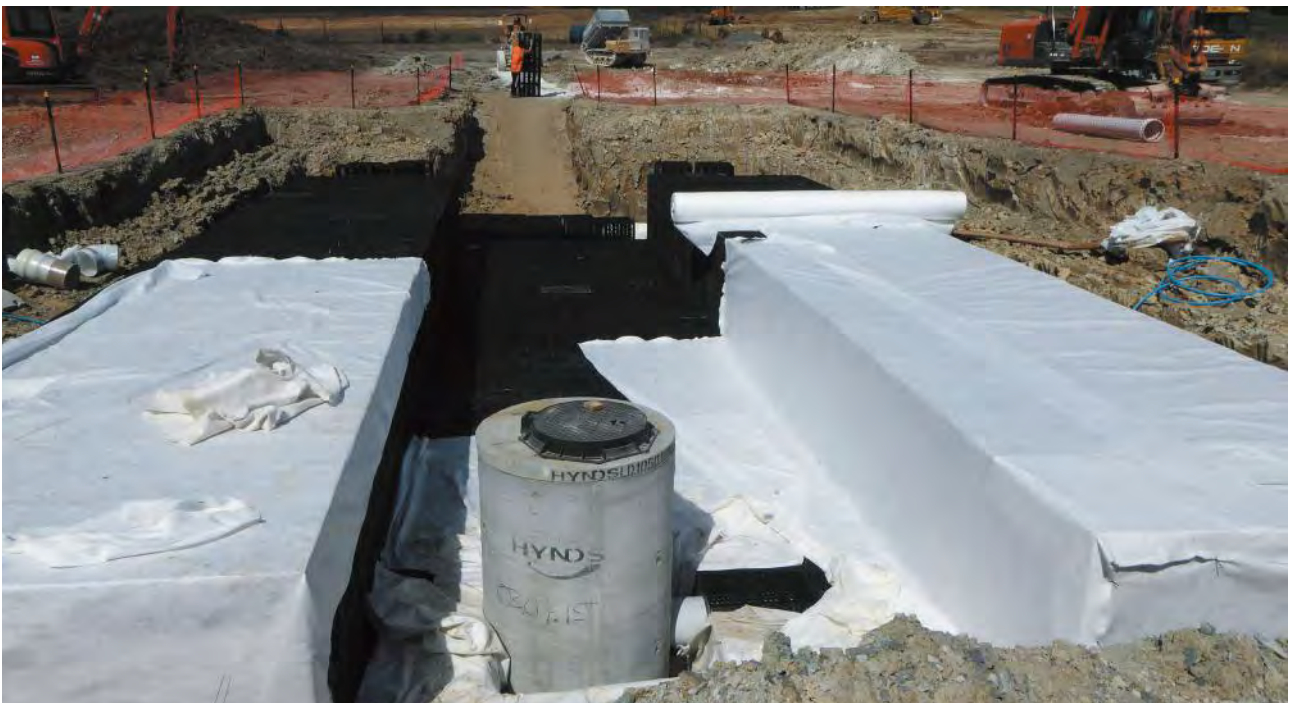
Fig. 18 Encapsulate RainSmart system with geotextile
