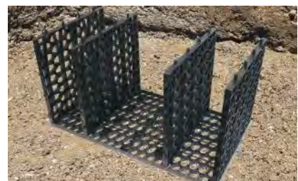
Fig. 13 Additional space for port can be created by moving the internal plates towards the ends
