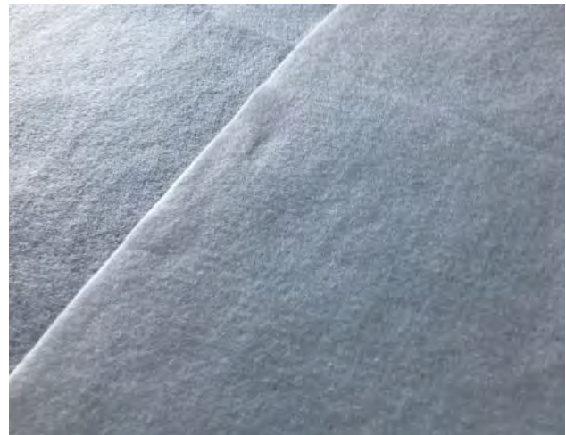
Fig. 7 Overlap geotextile by a minimum of 300mm
