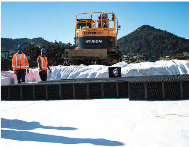
Fig. 6 Pull wrinkles out of geotextile so material lays flat
