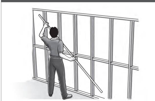
Figure 1: Frame straightness
