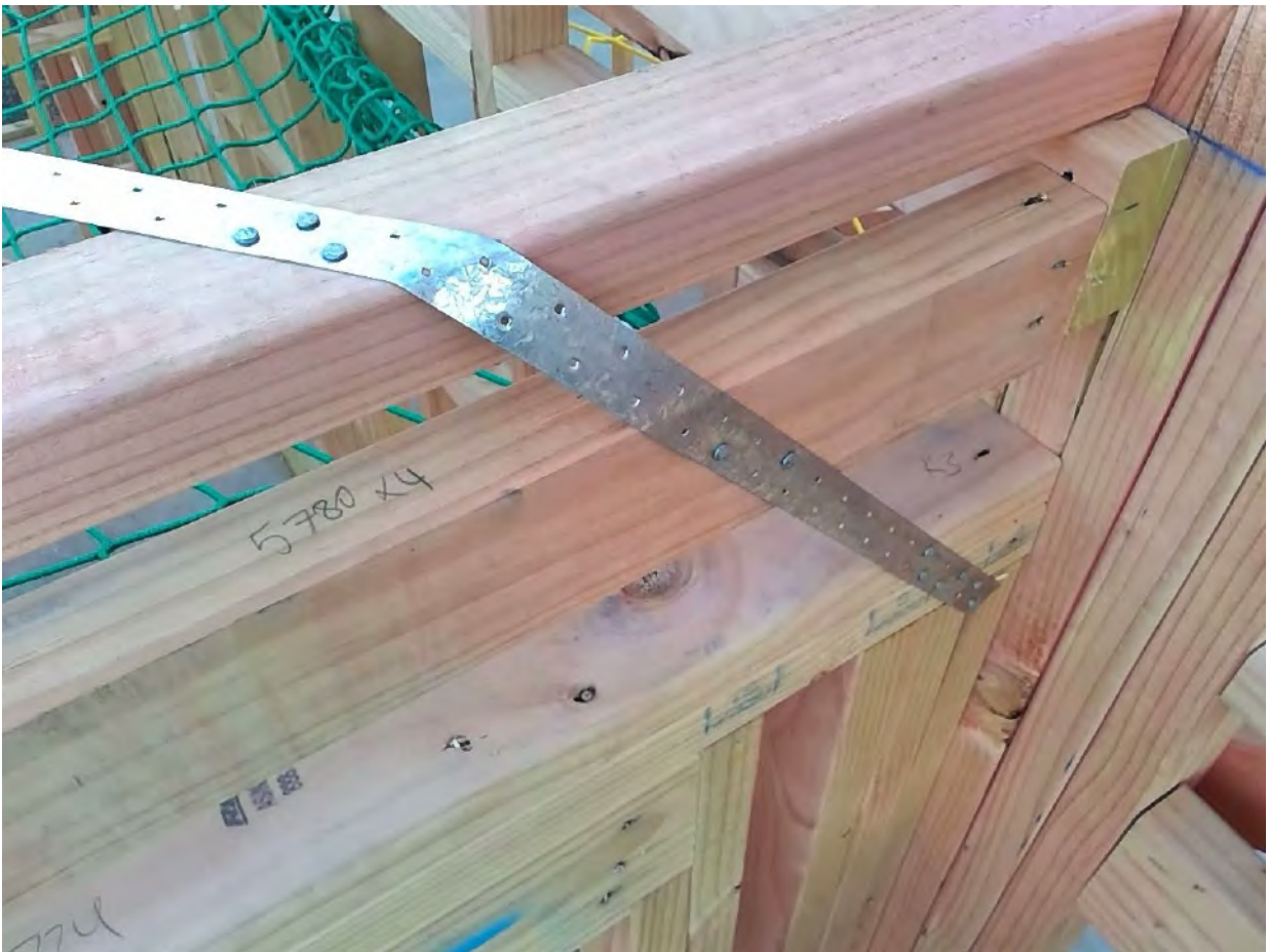
cross bracing connection Taken at 8:30 AM on Wednesday 9/06/2021
