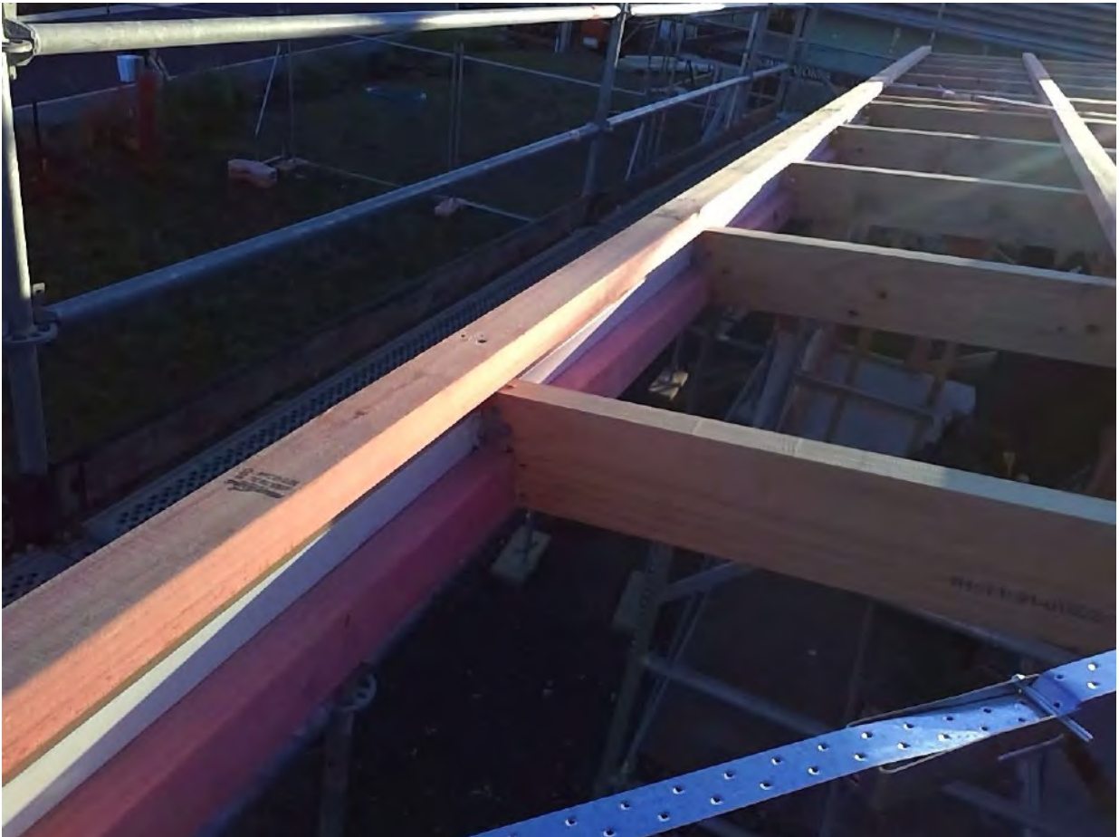
multigrip rafter connections
