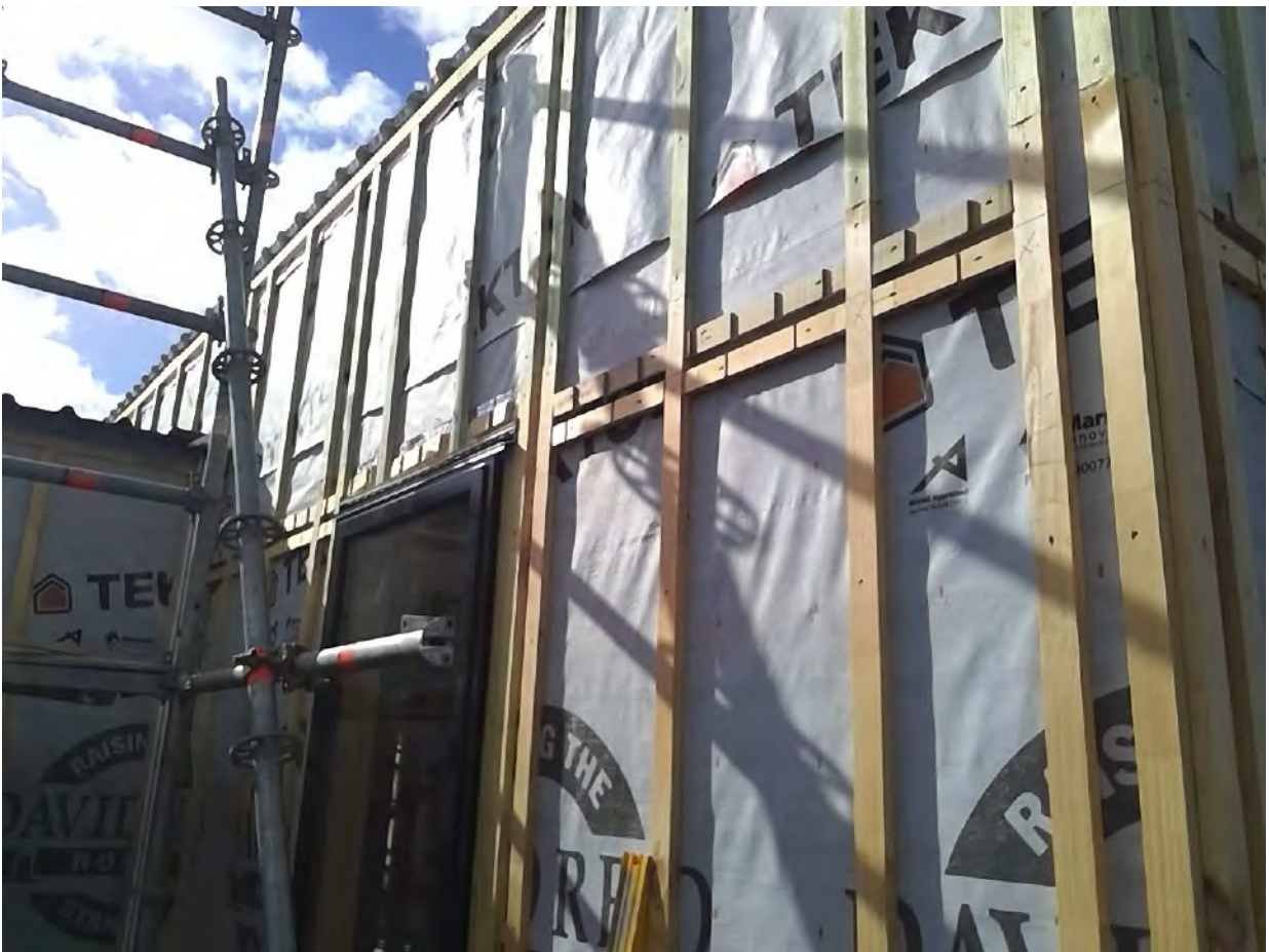
re battened gable wall. join fitted with fluted battens so cavity is maintained Taken at 11:42 AM on Wednesday 4/08/2021
