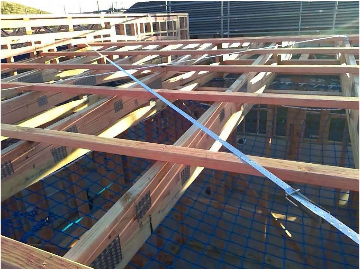
roof strap bracing Taken at 8:28 AM on Wednesday 9/06/2021
