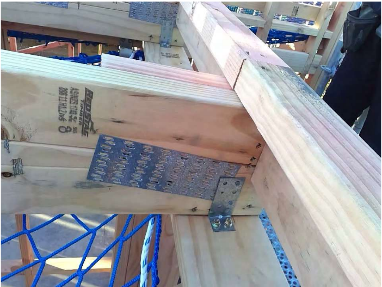
cpc40 rafters connections Taken at 8:28 AM on Wednesday 9/06/2021
