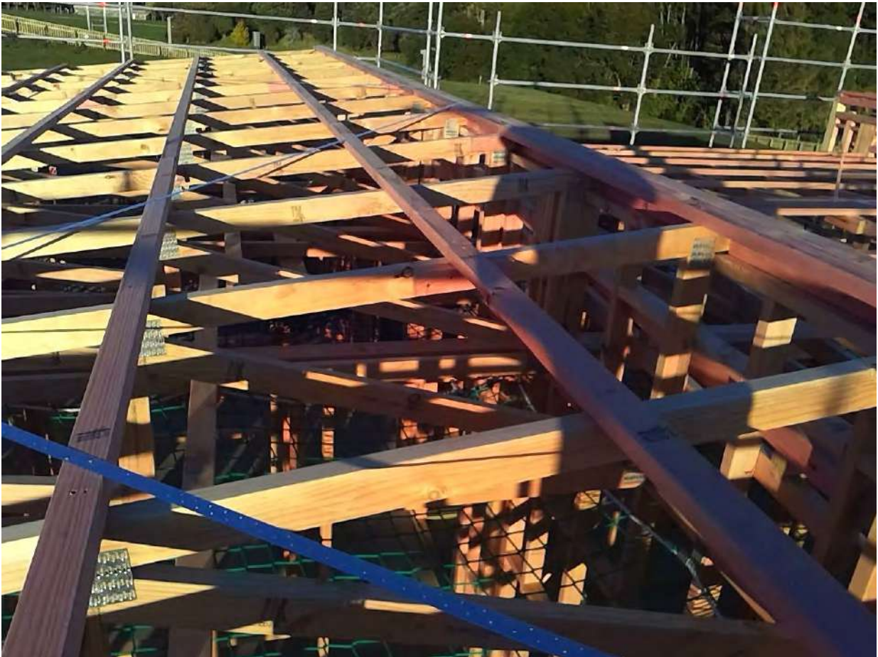
roof cross bracing Taken at 8:31 AM on Wednesday 9/06/2021
