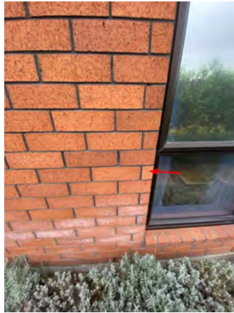
Typical cracking noted.
