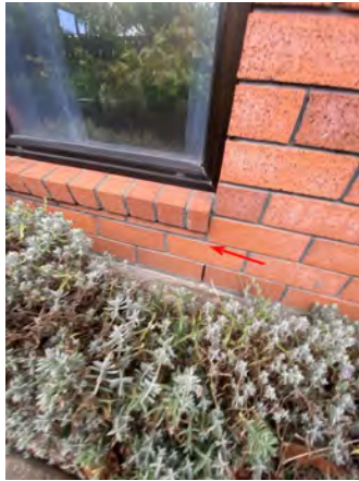
Typical cracking noted.
