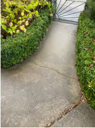
Typical cracking.
