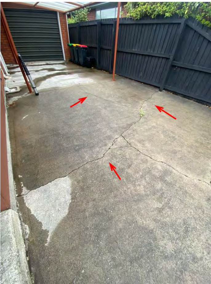
Typical cracking noted.
