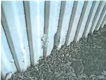
Patches to painted perspex cladding noted.
