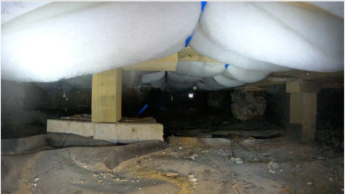
62: View of propping.
