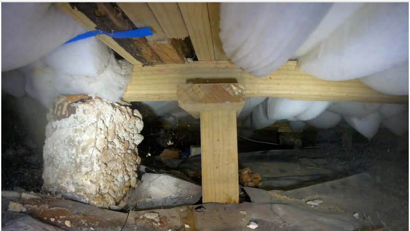
38: View of propping.
