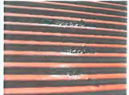
Some filler noted to roofing iron.
