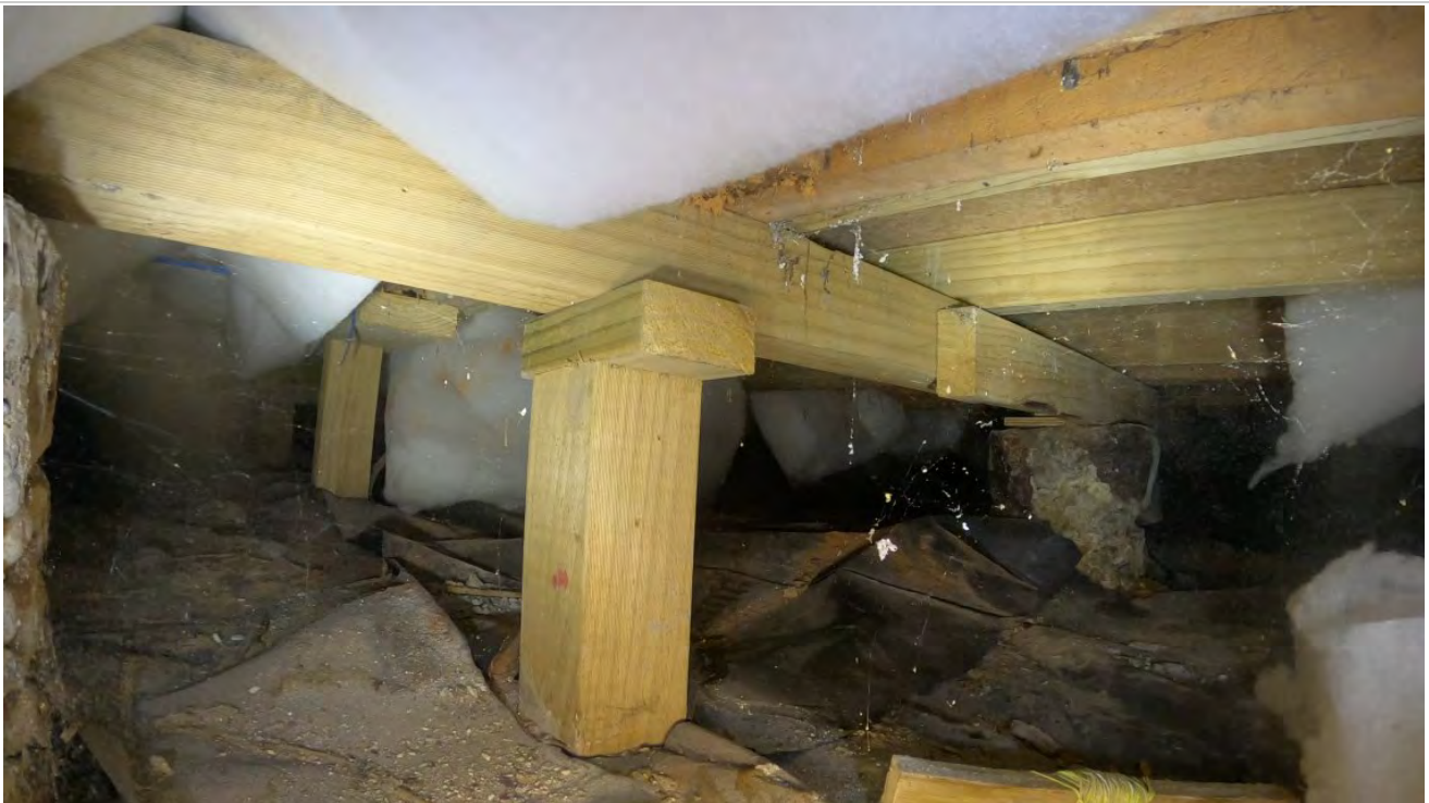
40: View of propping.
