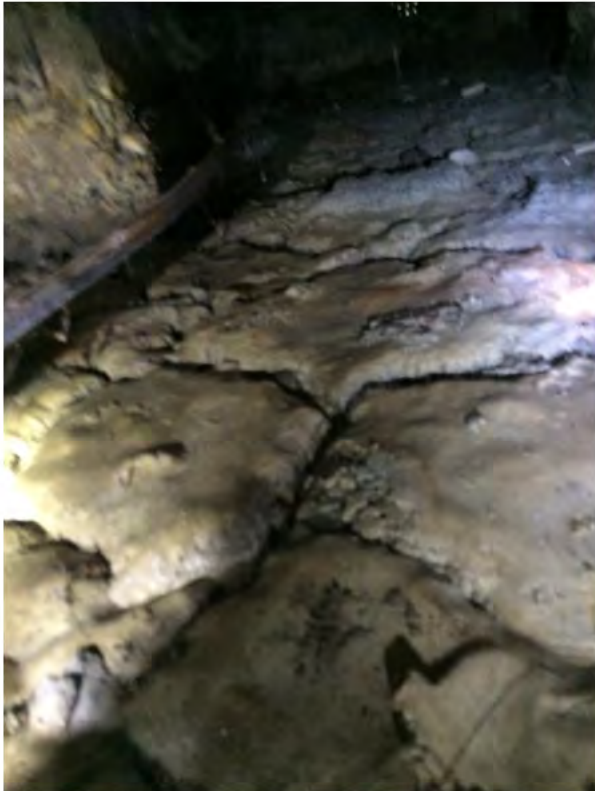
Appendix 1: Liquefaction in the subfloor space
