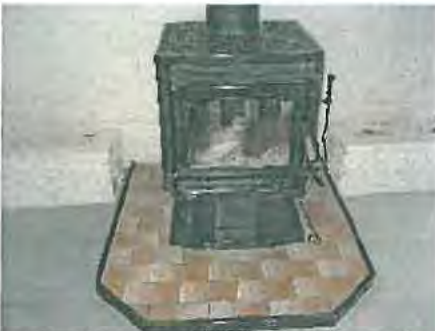
Wood burner to lounge appears in reasonable order.
