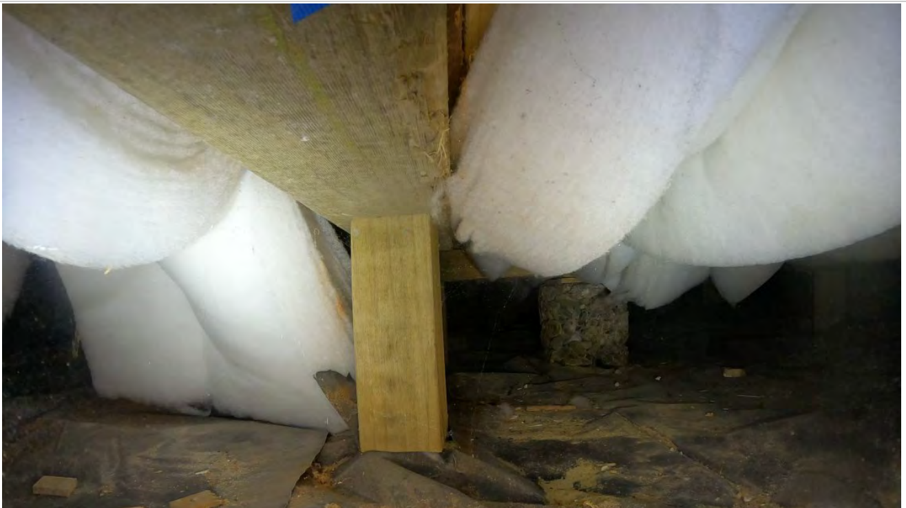
60: View of propping.
