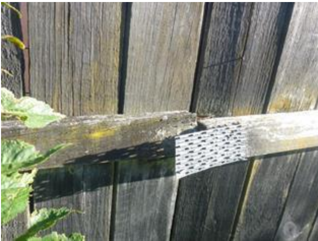
Railing repair
