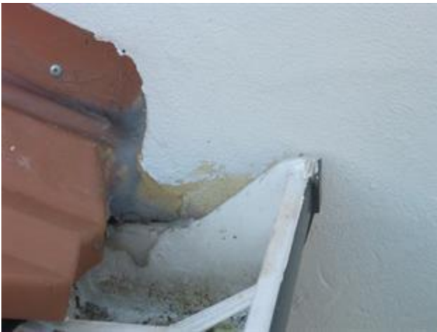
Kick out flashings recommended/ roof to wall junctions
