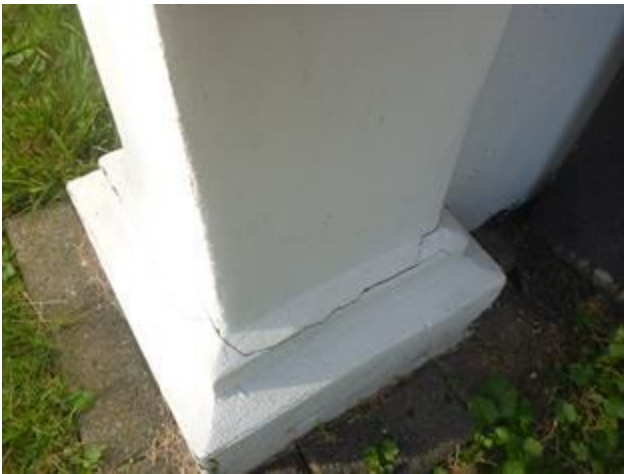
Impact damage side
