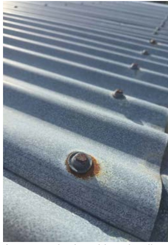
An example. Lead head nails.
