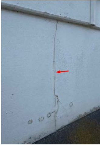
Isolated patches of cracking noted on the upstairs cladding.
