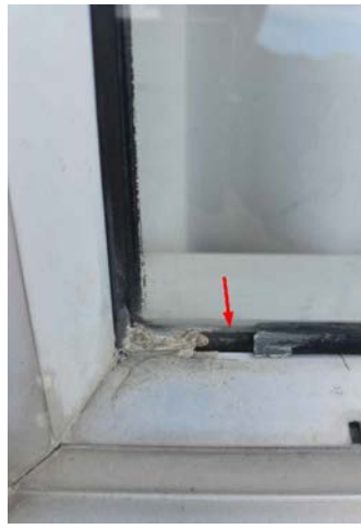
An example. The window rubbers have perished slightly.
