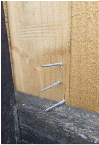
Several nails have missed throughout the east side fencing.
