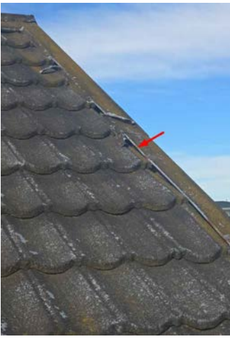
The flashing along the south side gable end is pulling up.
