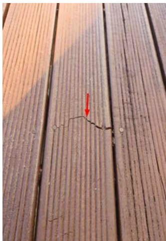
An example. The decking timber has snapped.
