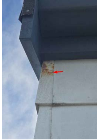
Surface rust noted on the southeastern corner soaker.
