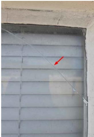
Cracked glazing.
