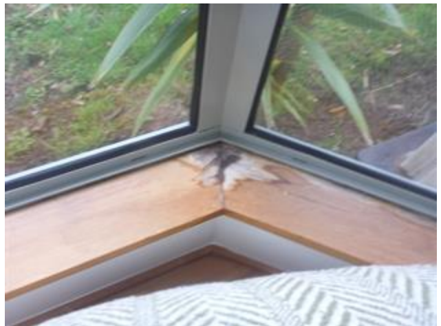
Moisture / UV damage
