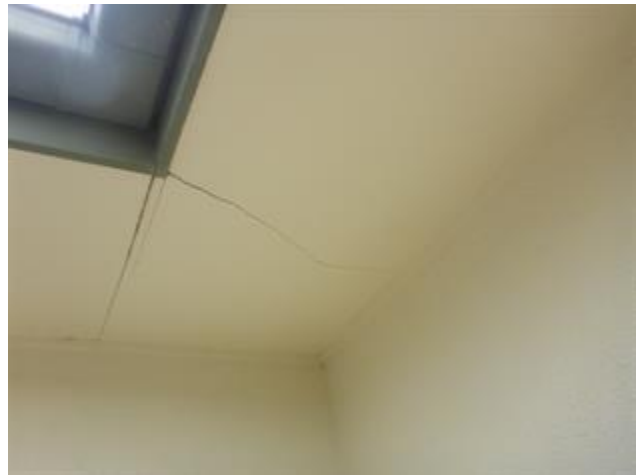
Cladding crack
