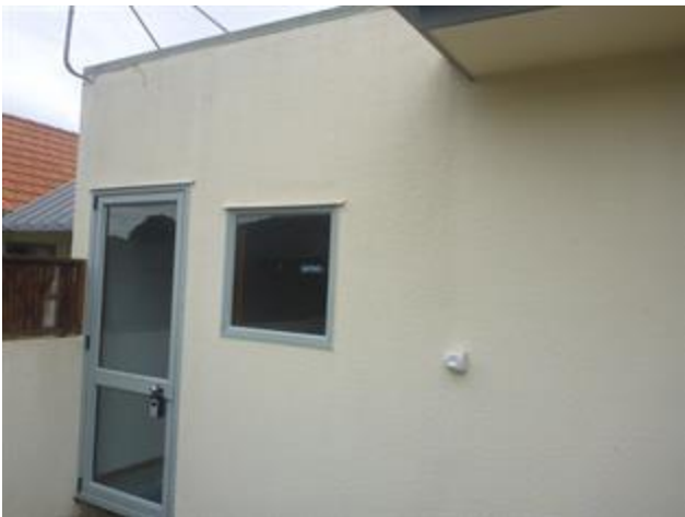
No soffit/metal cap flashed
