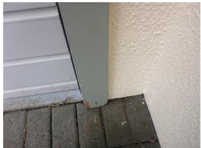
Bottom of cladding
