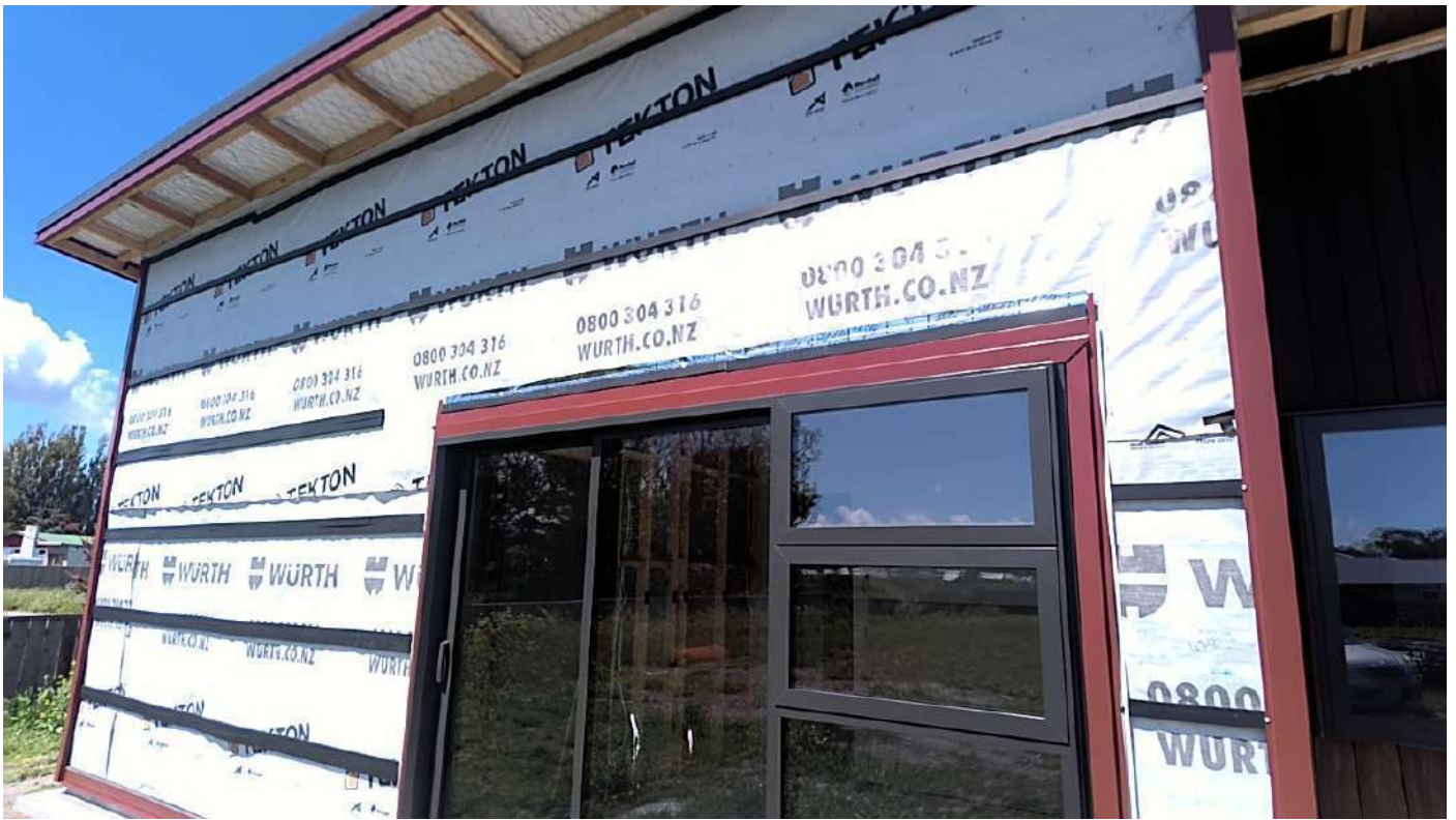
Metal cladding flashings Taken at 11:45 AM on Monday 3/11/2025
