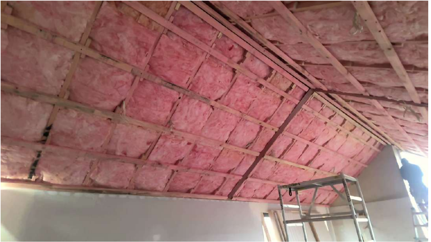
Ceiling insulation Taken at 11:45 AM on Friday 10/10/2025
