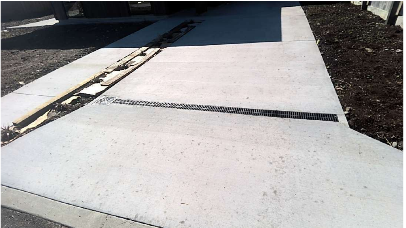
Stripdrain in driveway Taken at 10:29 AM on Wednesday 28/01/2026
