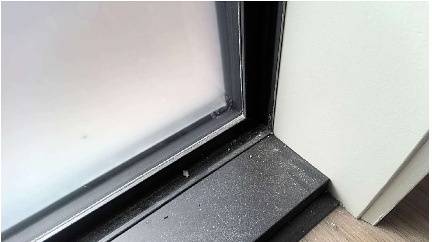
Safety glass in bathroom windows Taken at 10:46 AM on Wednesday 28/01/2026
