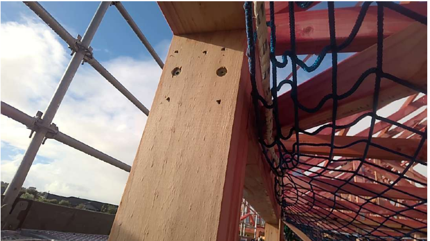
Main bedroom - indicative lintel fixing method Taken at 2:49 PM on Monday 14/07/2025
