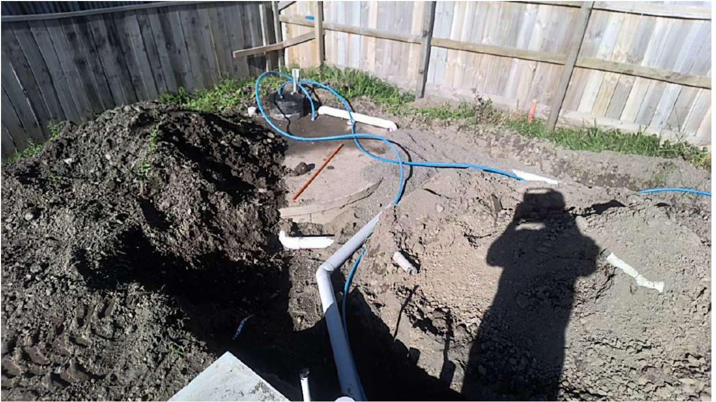
stormwater to tank
