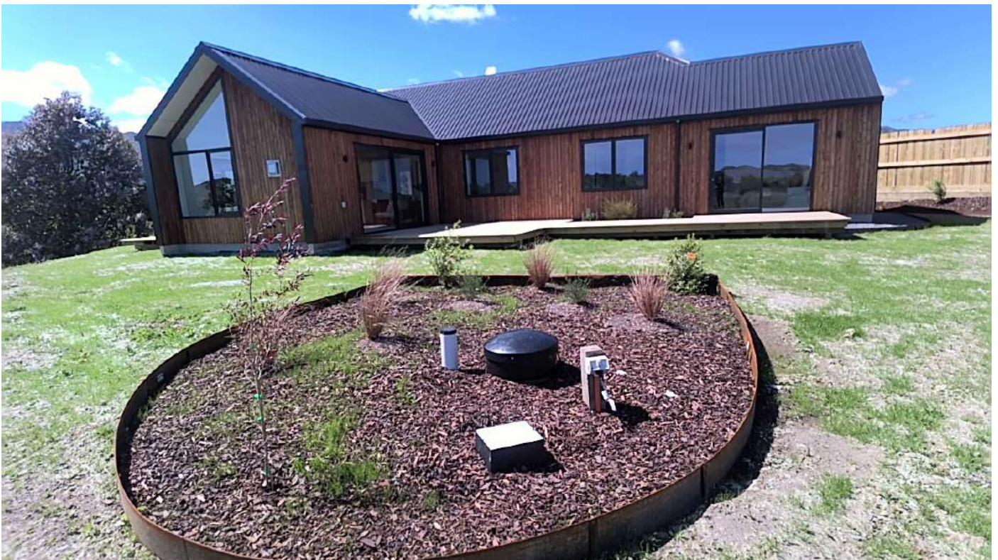
Non potable supply tank in ground
