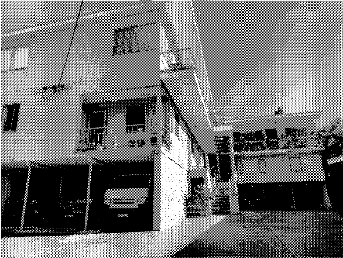
Figure 1 - Site as viewed from Gosford Road
