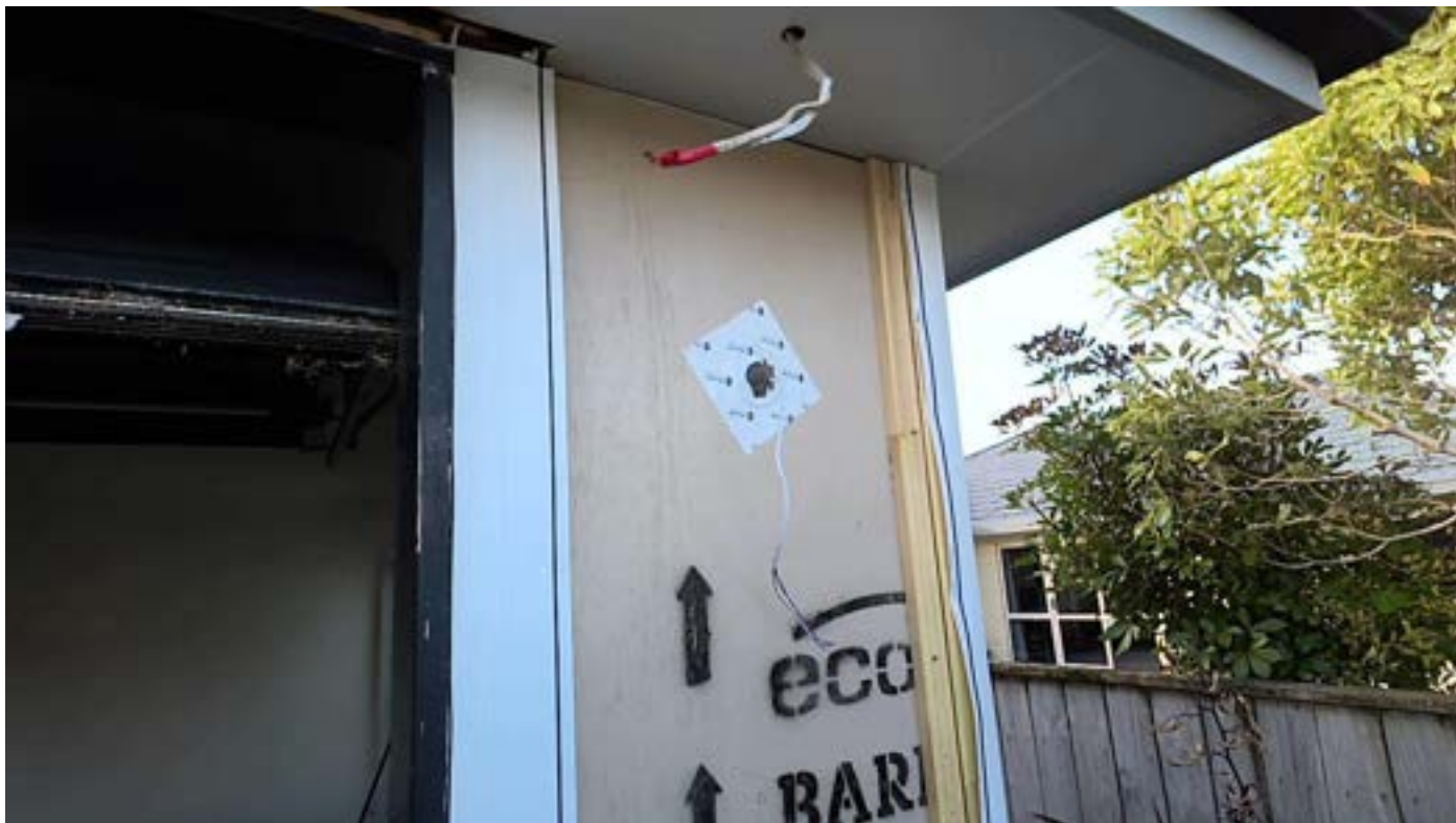
Typical marshall seal to penetration Taken at 8:27 AM on Thursday 24/08/2023
