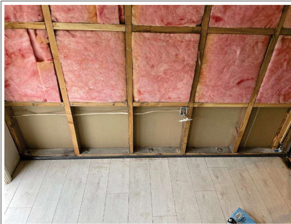
Handibracs in place
