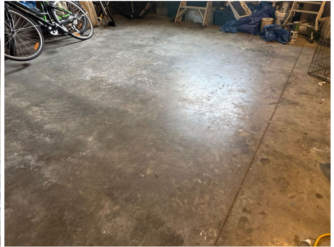
The exposed concrete slab in the garage is in an average condition for the age. No damage sighted.
