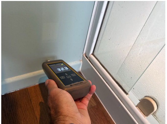
The common fail areas of the shower and plumbed areas were checked for elevated moisture. Moisture levels were within the normal range.
