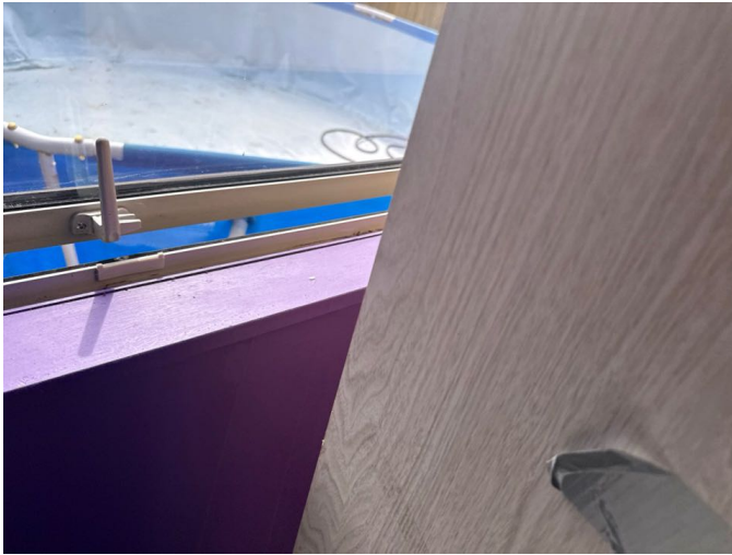
The windows are functioning throughout
