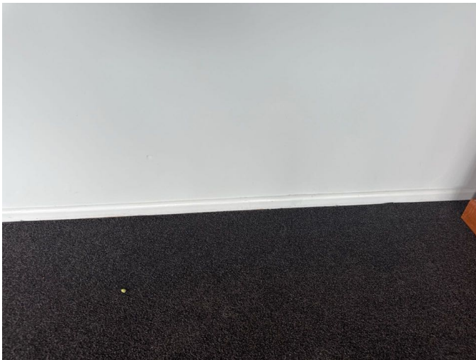
The wall and ceiling linings and carpet are in a tidy condition
