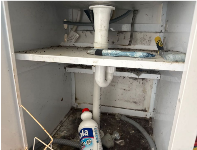
No concerns with the waste or water feeds beneath the tub
