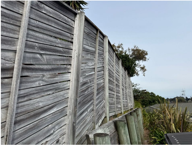
The perimeter fencing is solid and intact.
