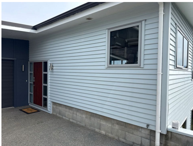
The front door faces to the Southeast
