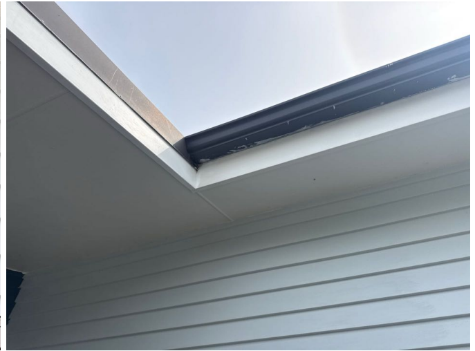
Generally good paint seal to the timber barge boards, fascia and fibre cement soffit linings
