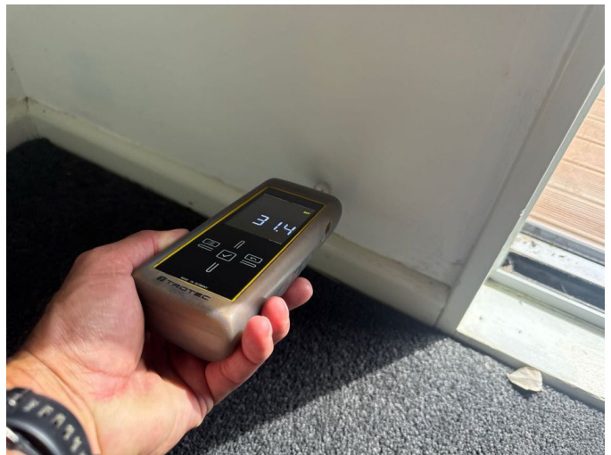
Moisture levels to the external walls were within the normal range at the time of inspection
