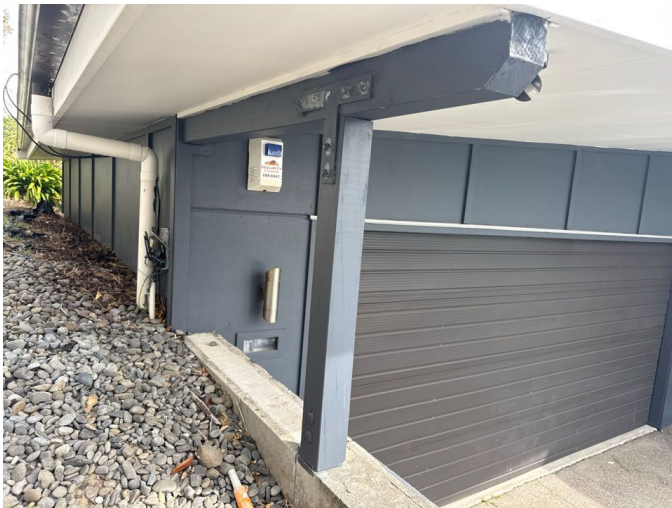
The timber roof support is solid and secure
