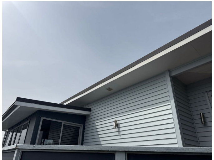
Good eave protection noted
