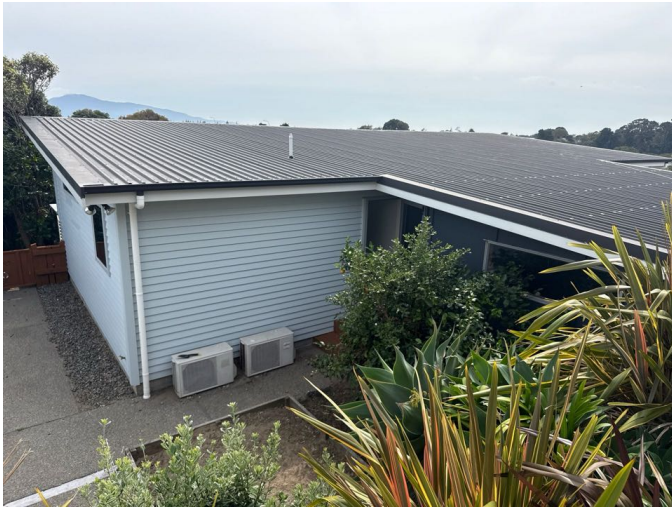
The Southwest side
