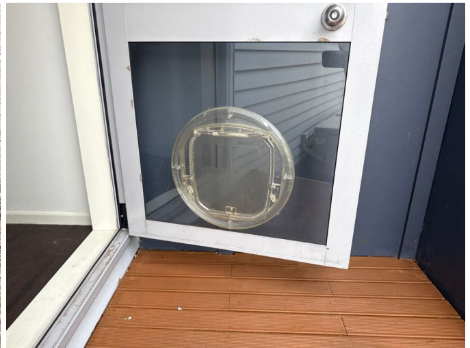
Small dog door installed
