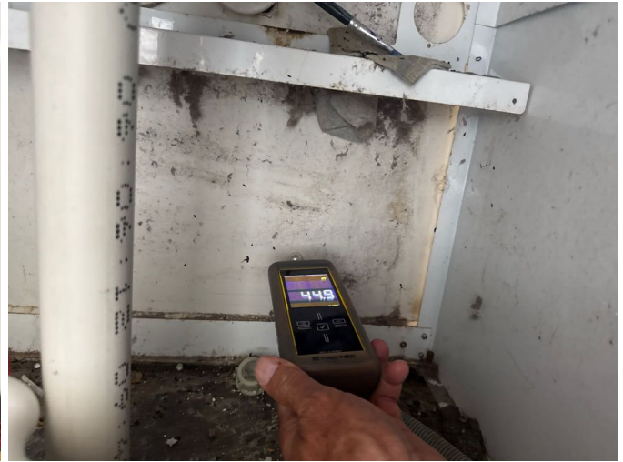
Moisture levels in the laundry were within the normal range at the time of inspection.
