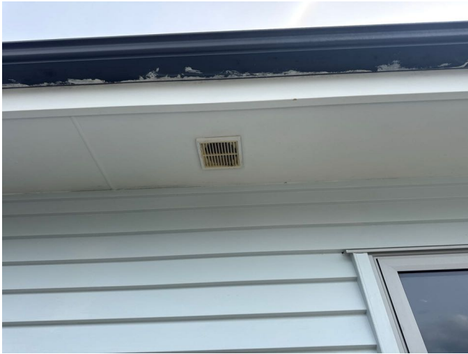
Extraction vents exit through the soffits
