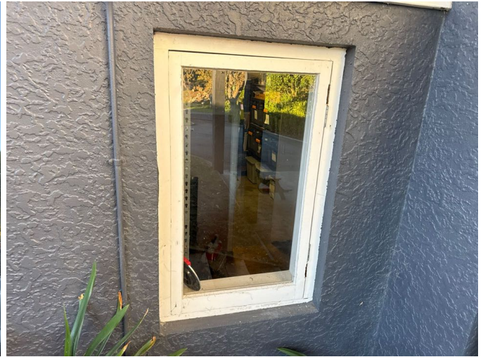
Windows rebated into the concrete foundation walls are effectively sealed
