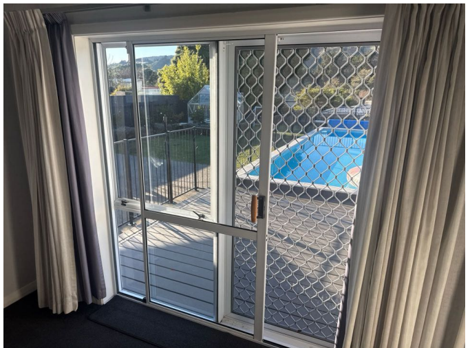
The sliding door is functioning. Security door noted.
