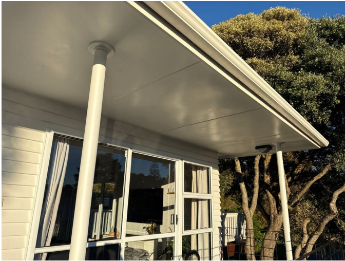
The steel roof supports are solid and secure
