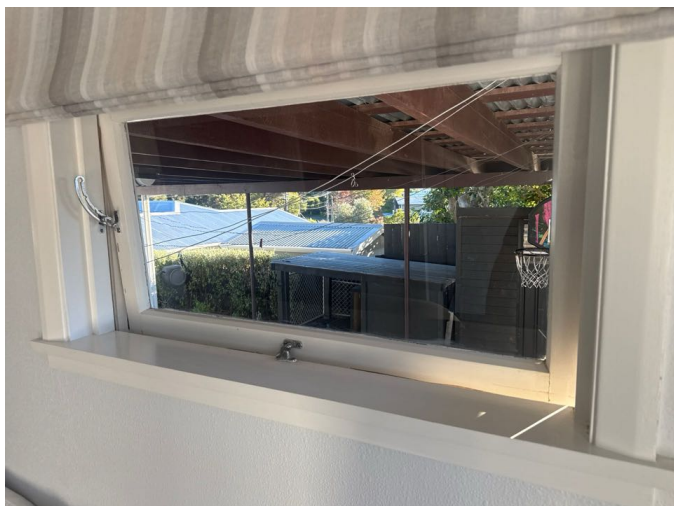
The timber windows are functional
