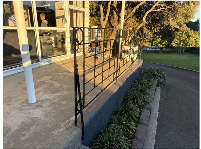
The steel balustrade is secure
