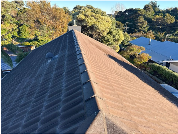
The concrete tile roof has a good overall appearance
