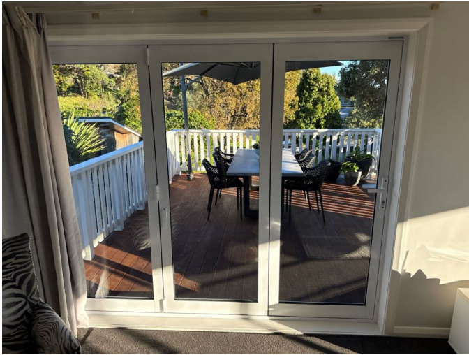
Doors and windows are functional
