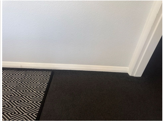
The wall and ceiling linings and carpet are in good condition
