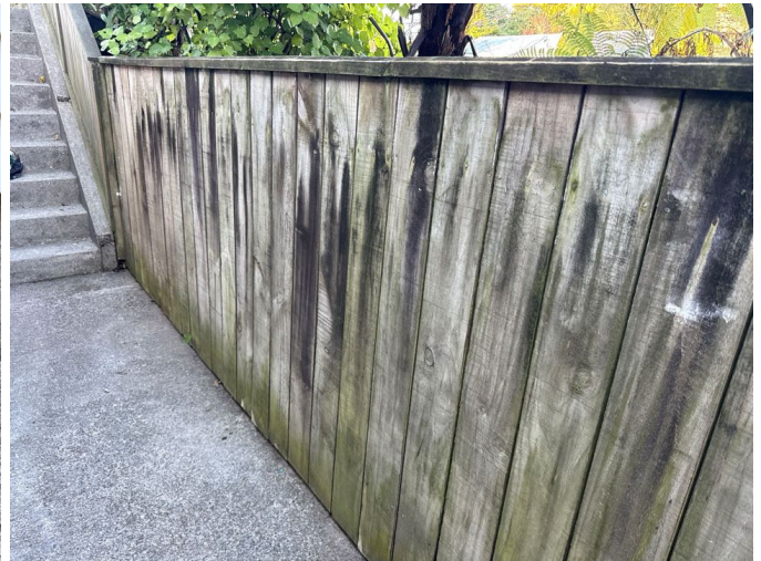
The perimeter fencing is generally solid and intact.
