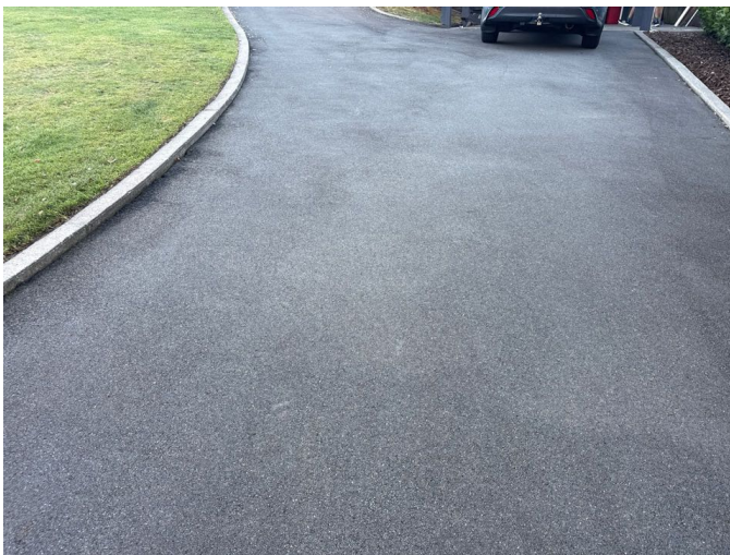
The sloping driveway is in good condition
