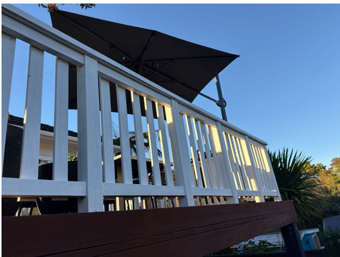
The balustrade is solid and connected sufficiently at the base
