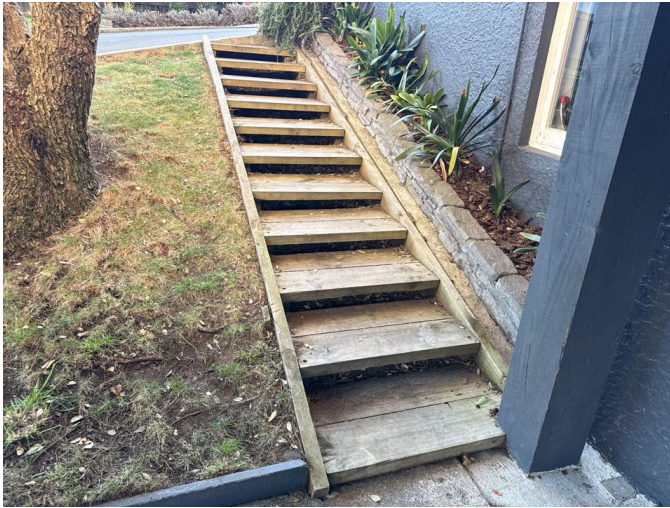
The timber stairs are secure and functional
