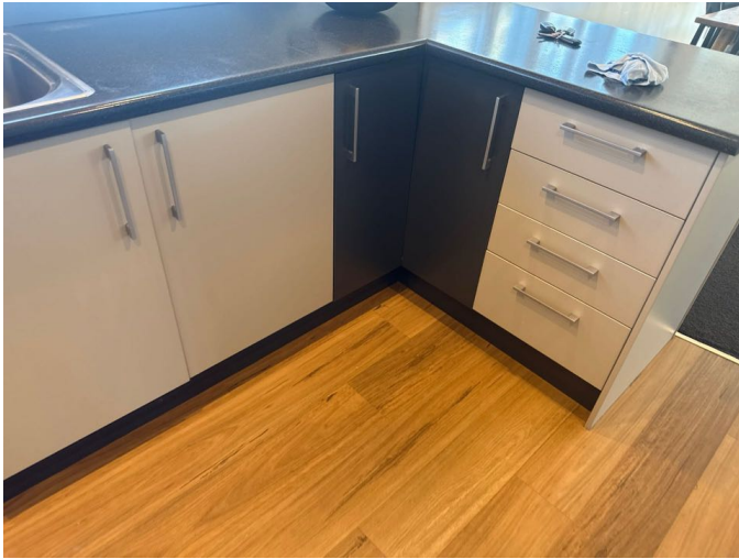
The kitchen cabinetry and vinyl floor are in good condition
