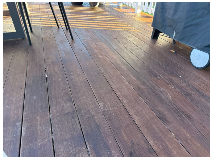
The timber decking is in good condition
