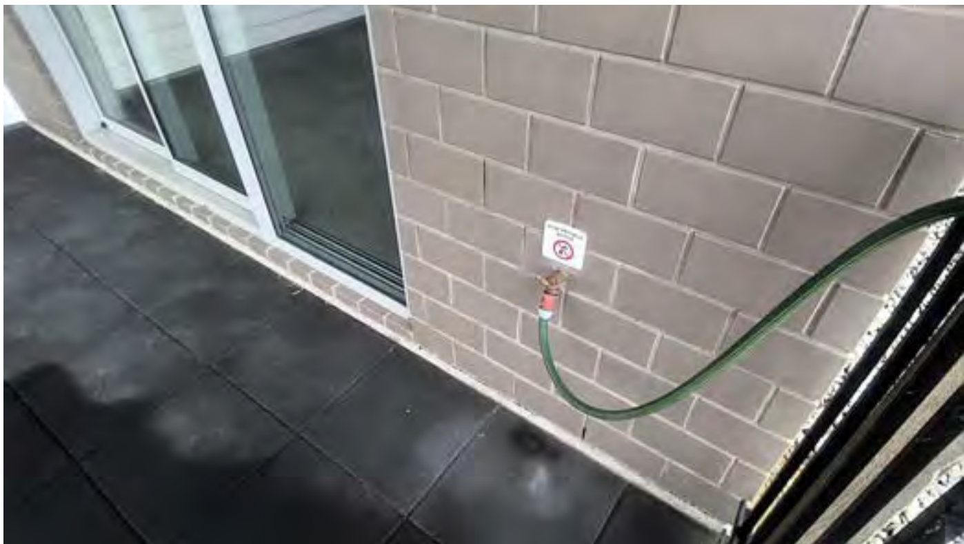
non potable water sign Taken at 9:55 AM on Friday 20/12/2024
