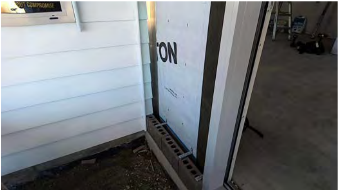
North slider off living area - typical tie set up for bottom course
