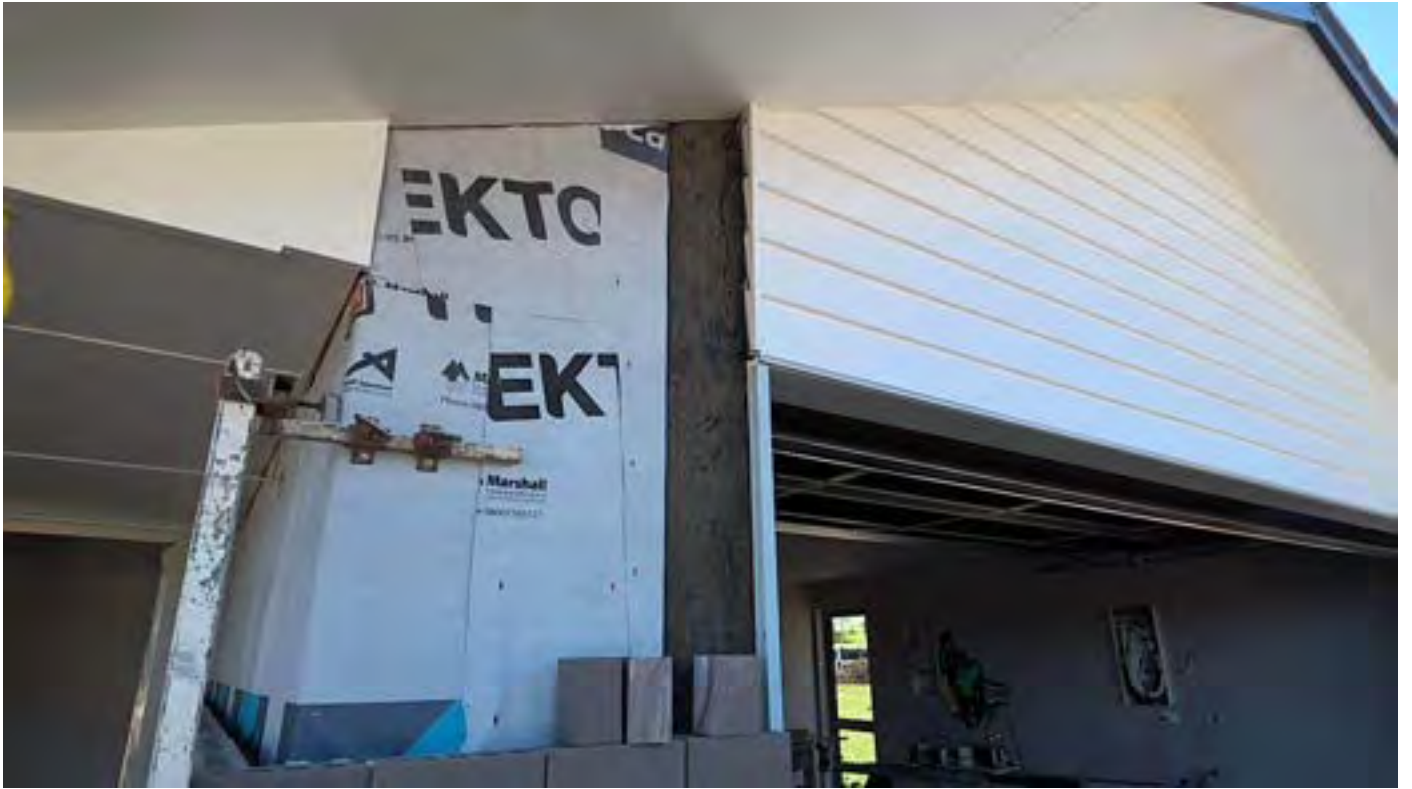
DPC at the wet/dry cavity junction Taken at 10:51 AM on Friday 8/09/2023
