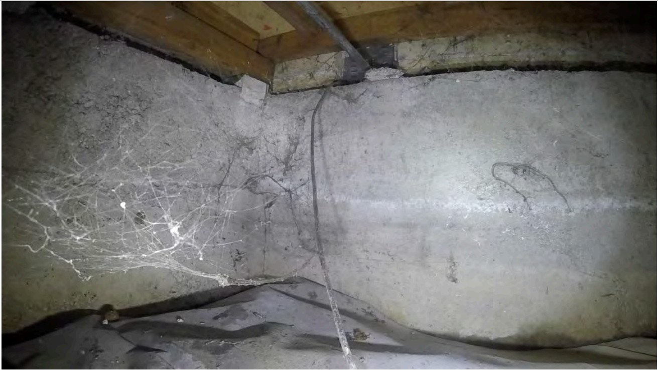
5: View of ring foundation.
