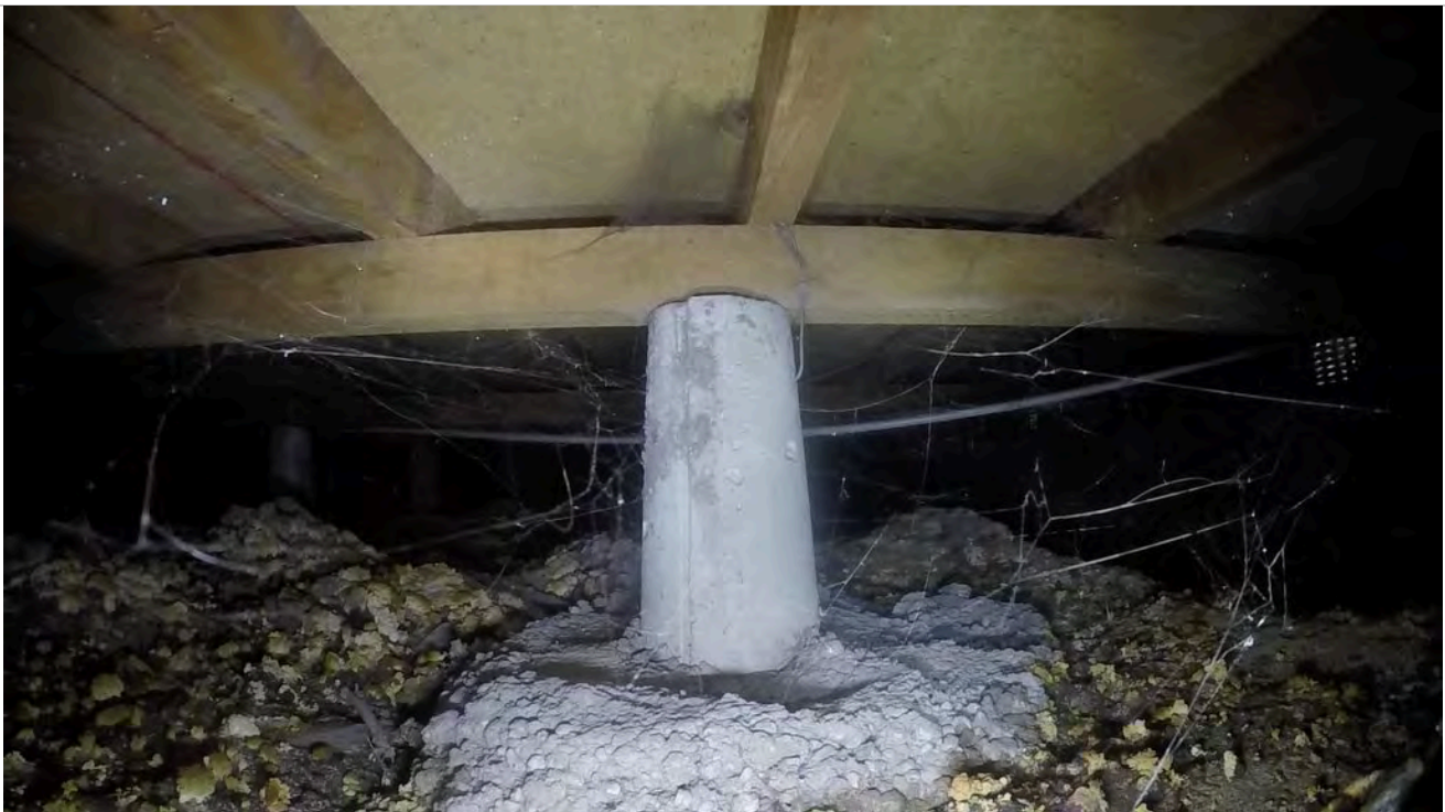
40: Pile with connection.
