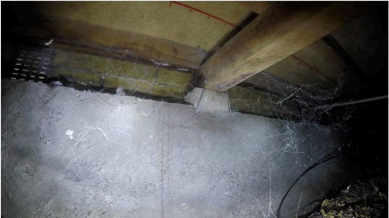
26: View of bearer meeting ring foundation with connection.
