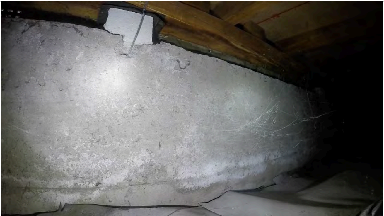
46: View of ring foundation.
