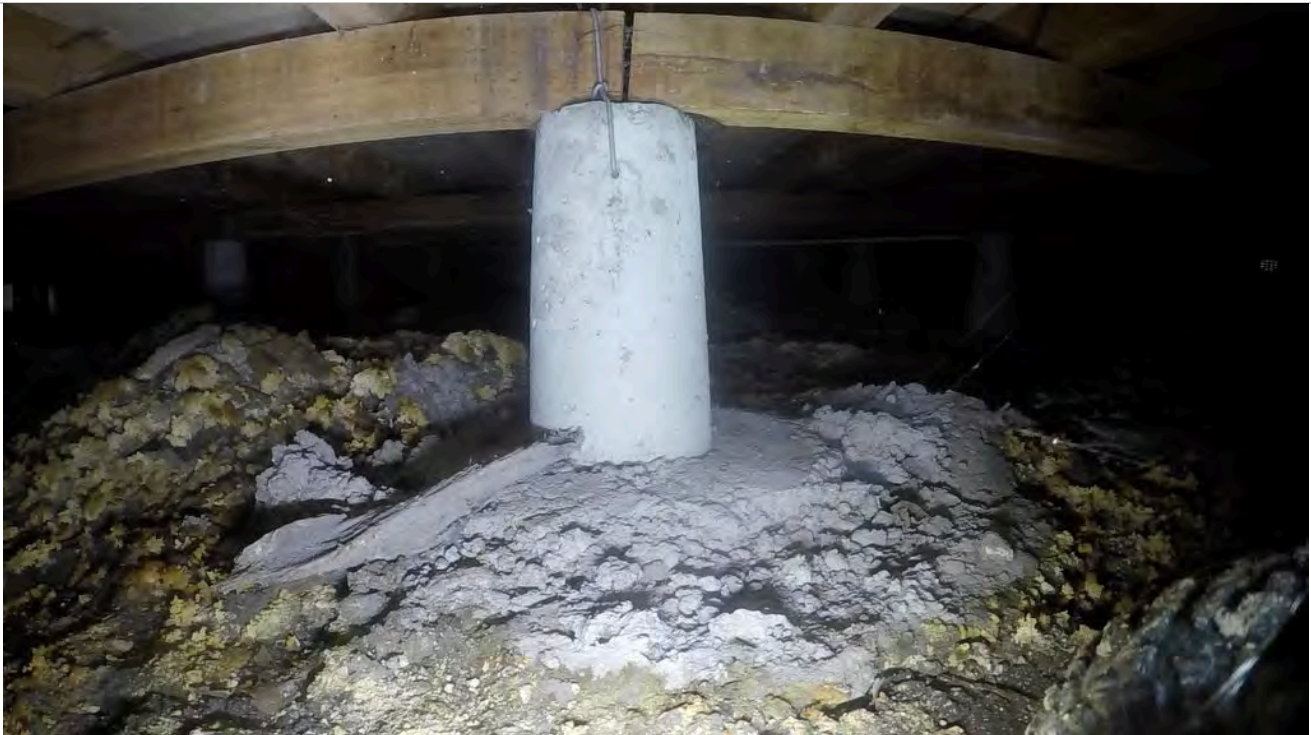
38: Pile with bearer join.
