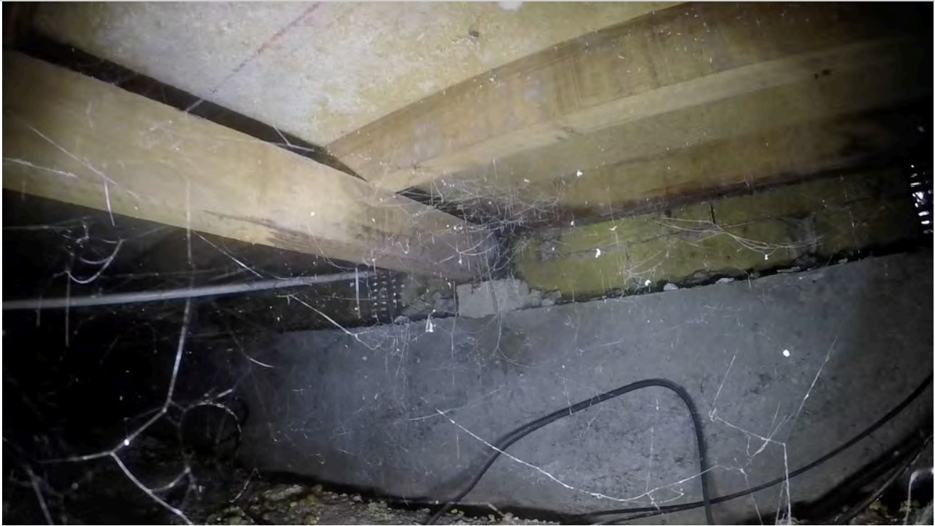
41: View of bearer meeting ring foundation with connection.
