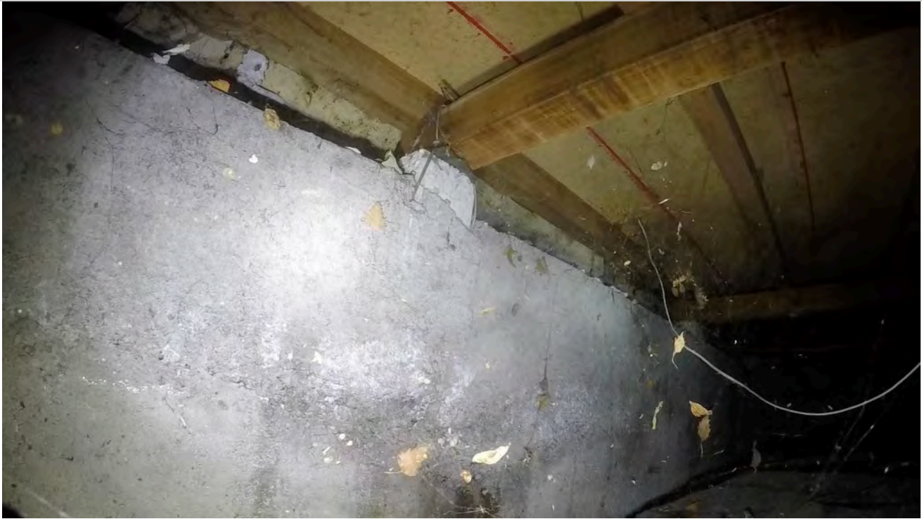
25: View of bearer meeting ring foundation with connection.
