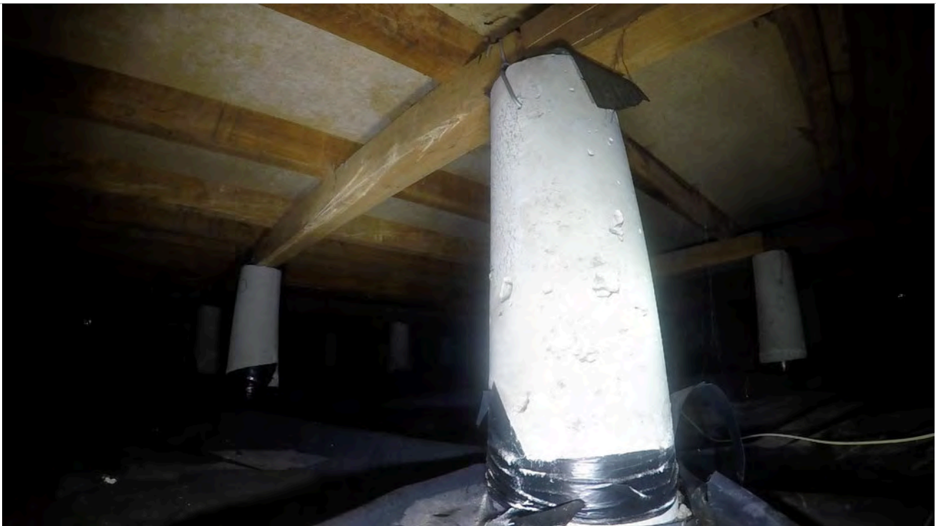
12: Pile with bearer join.
