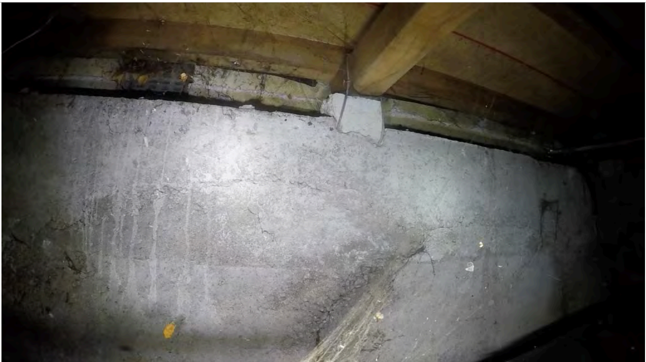
42: View of bearer meeting ring foundation with connection.
