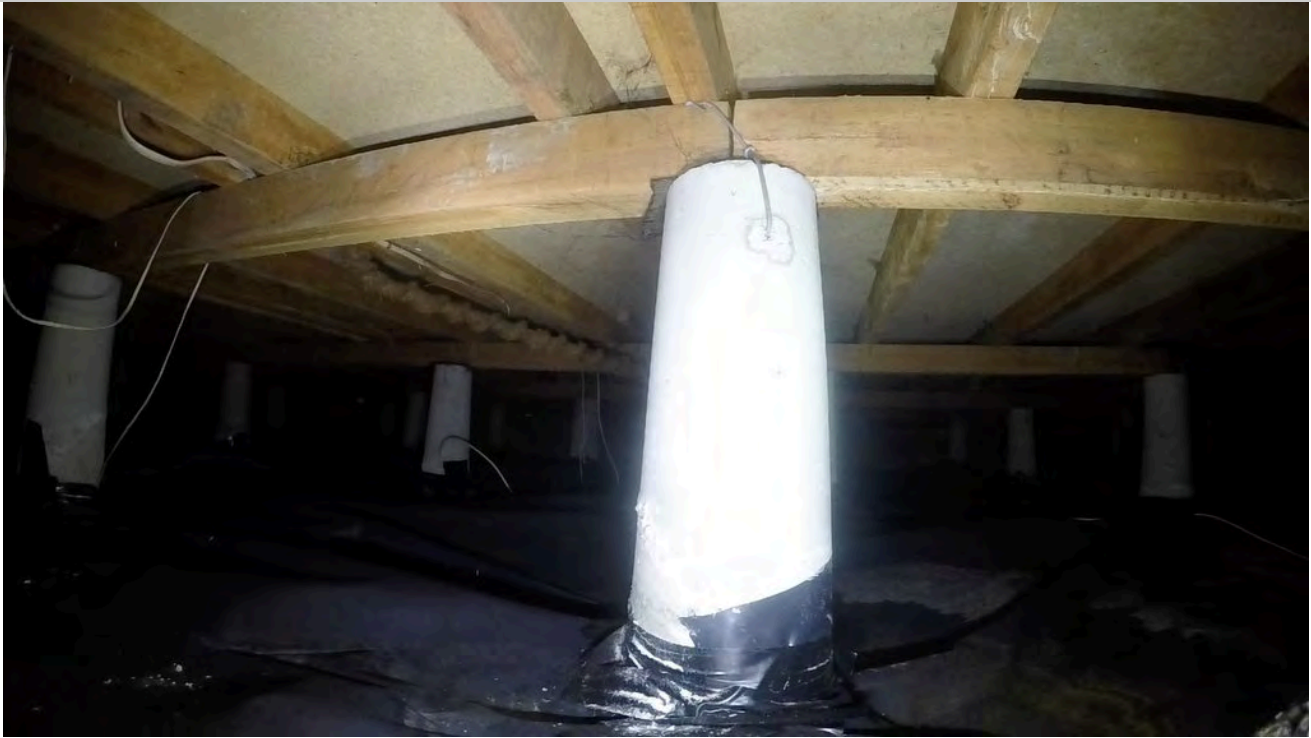
11: Pile with bearer join.
