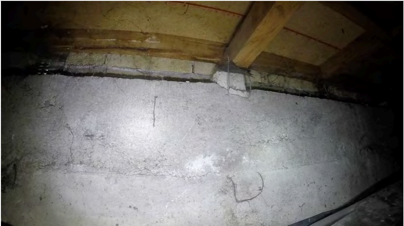
24: View of bearer meeting ring foundation with connection.
