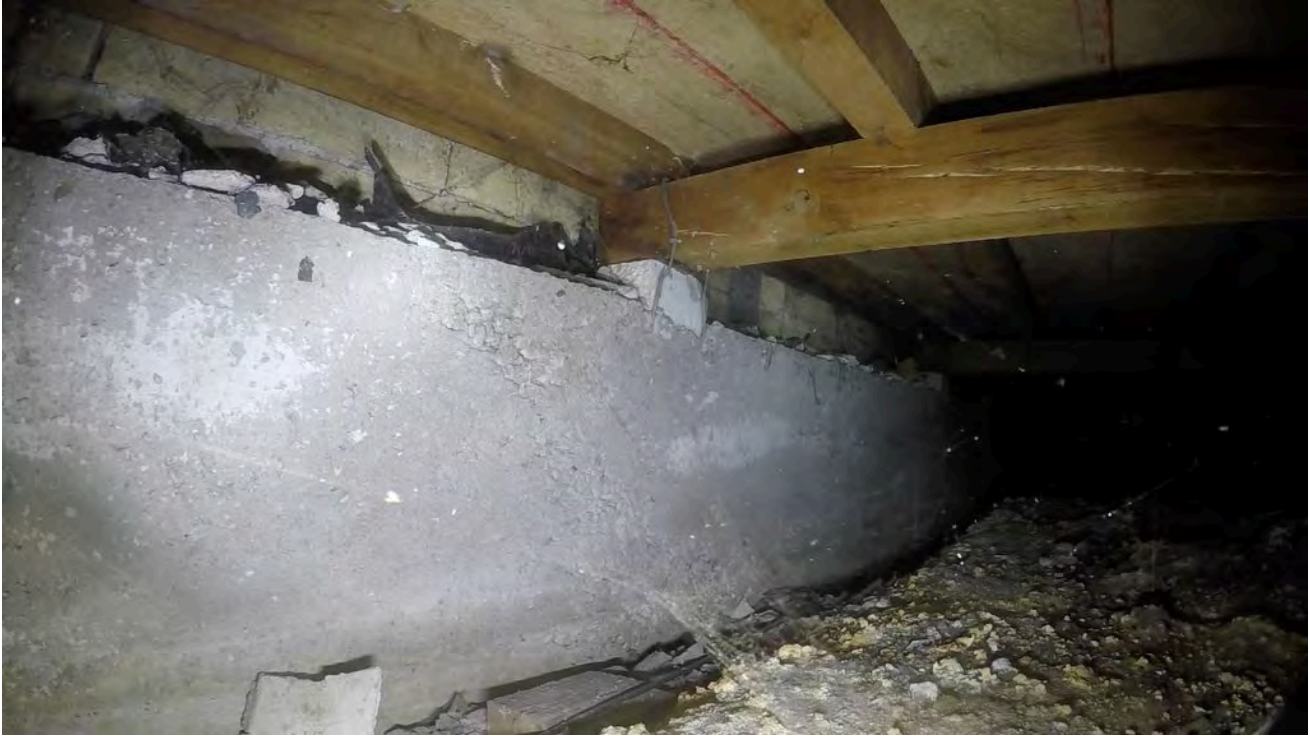
11: View of bearer meeting ring foundation with connection.
