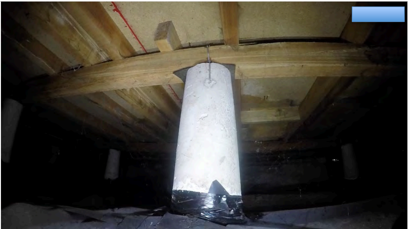
28: Pile with connection.
