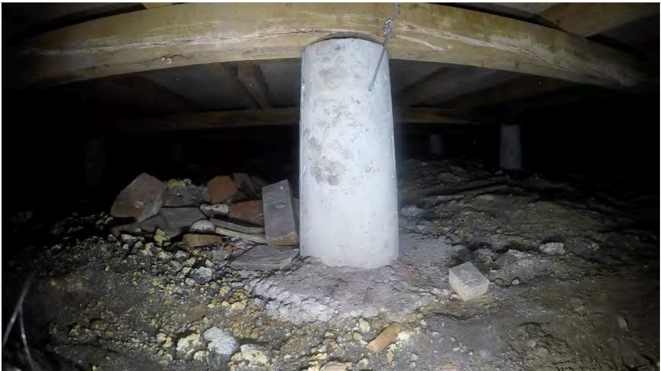
20: Pile with connection.
