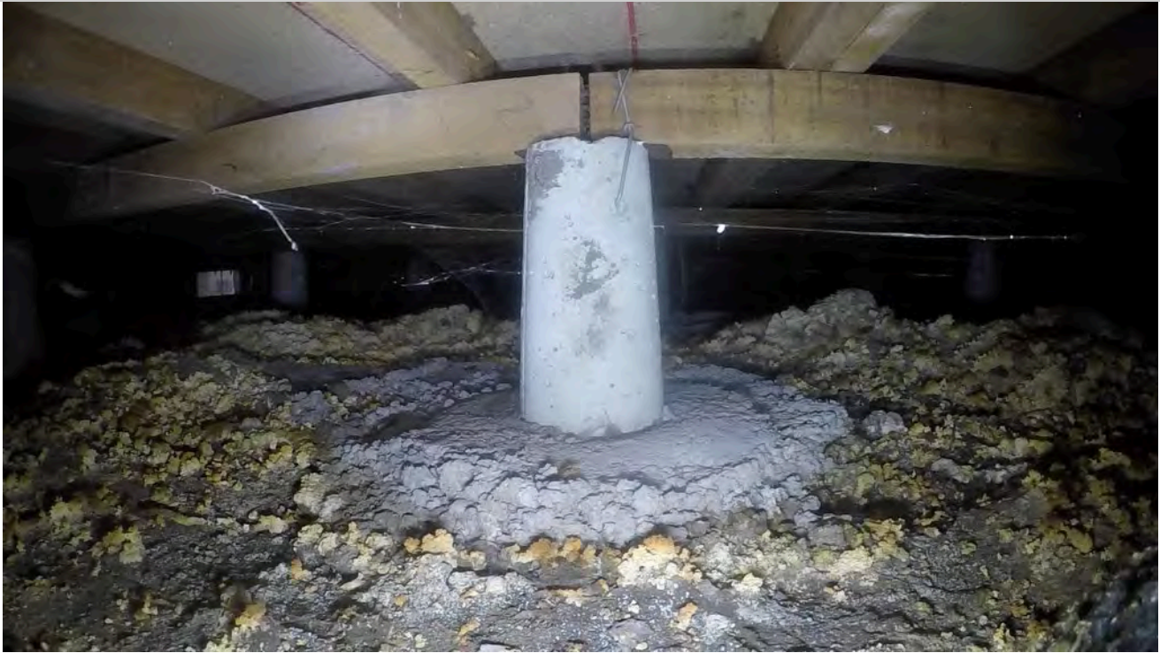
37: Pile with bearer join.
