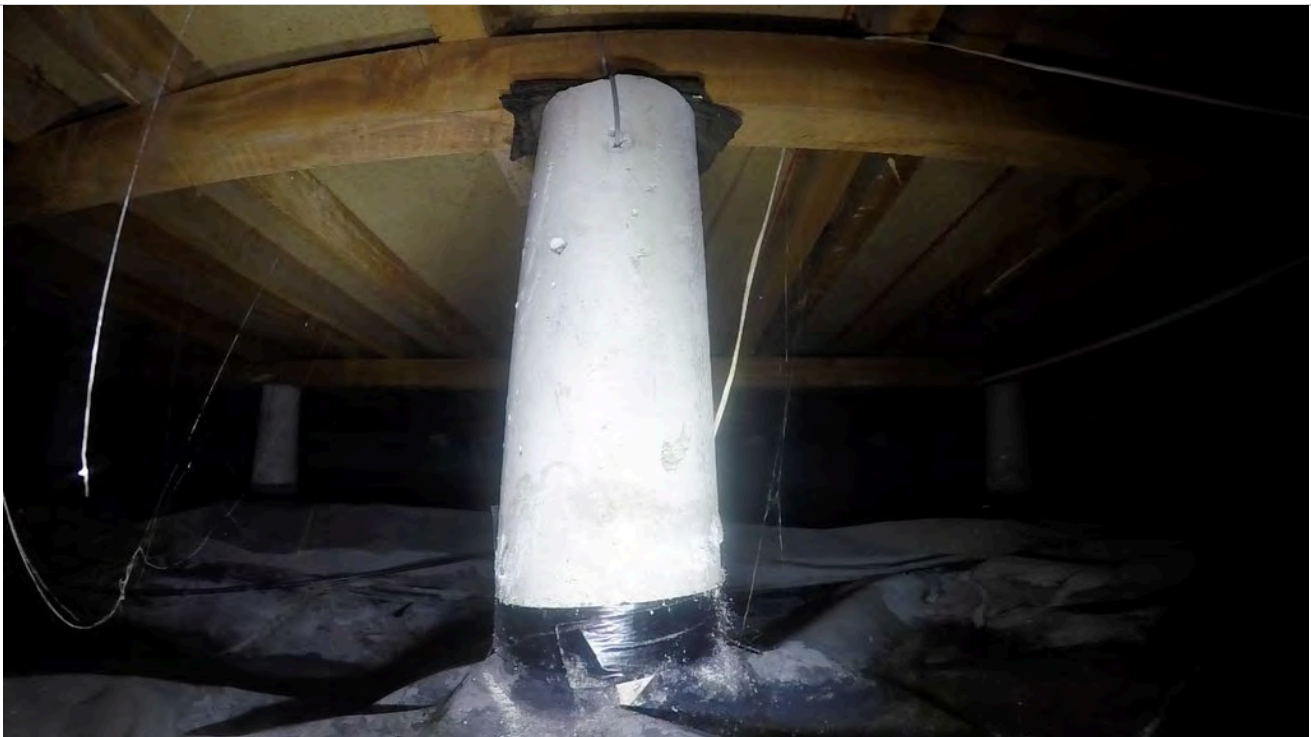
22: Pile with connection.
