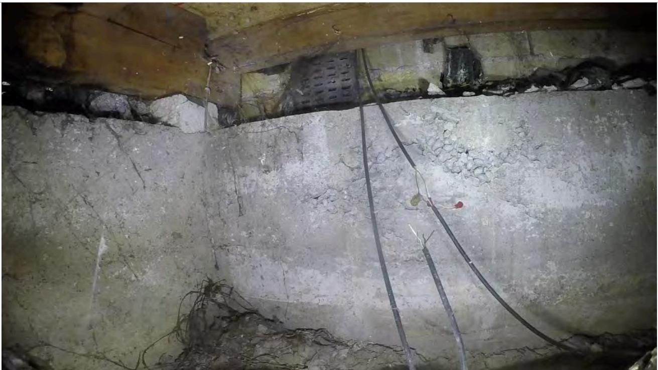
10: View of ring foundation.
