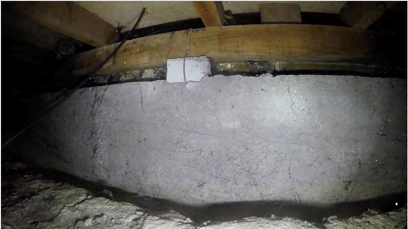
8: View of ring foundation.
