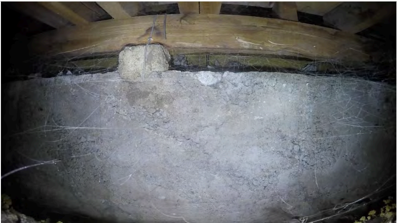
44: View of ring foundation.
