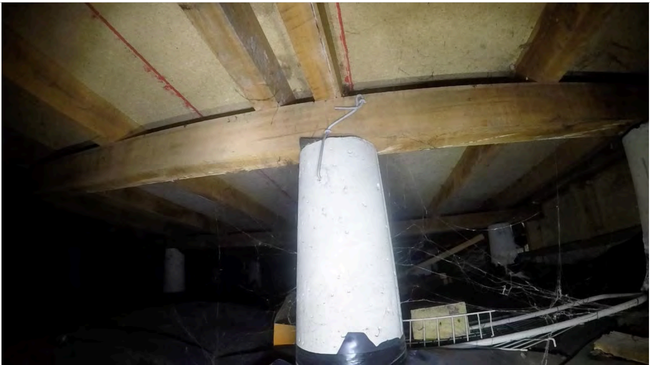
14: Pile with connection.
