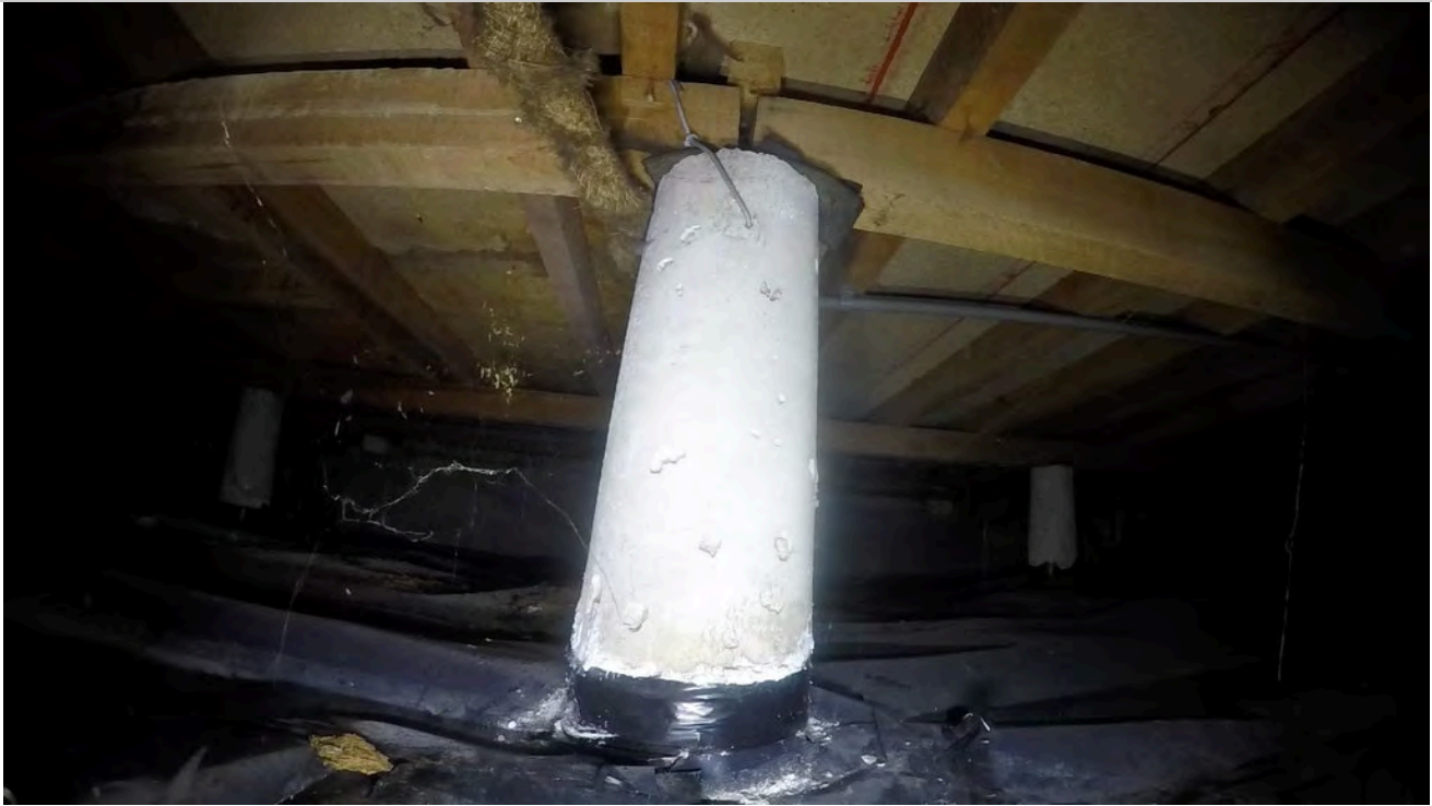
29: Pile with bearer join.
