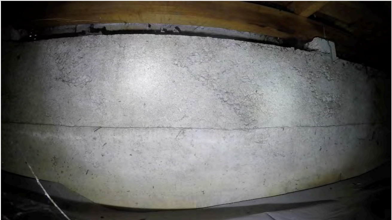
6: View of ring foundation.
