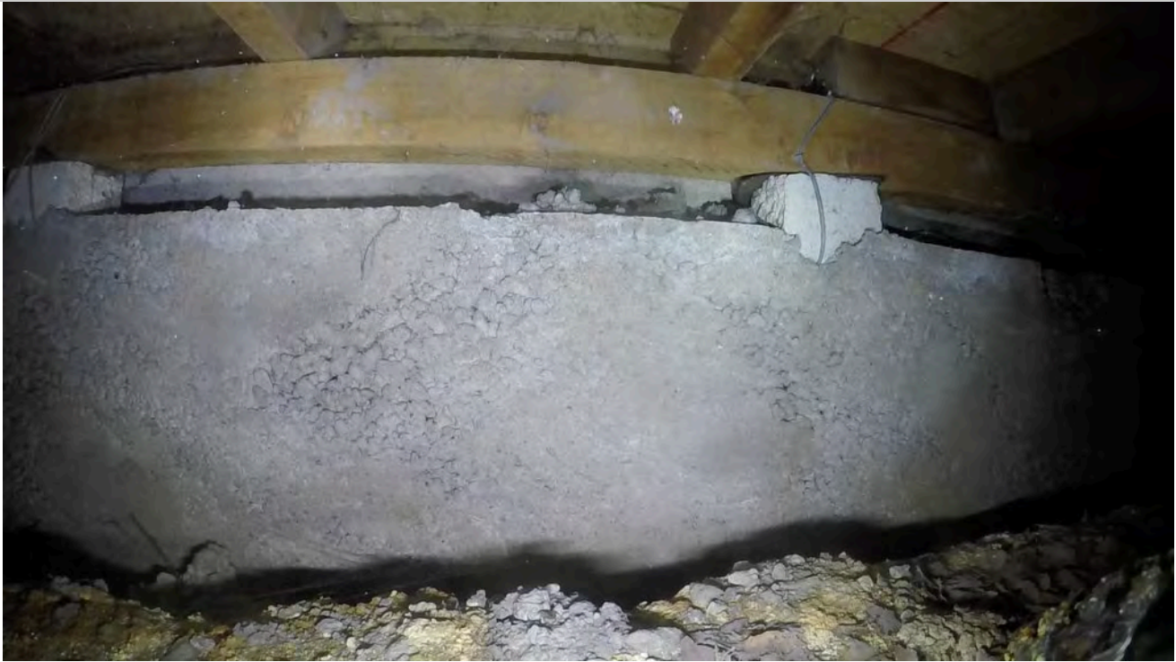
43: View of ring foundation.
