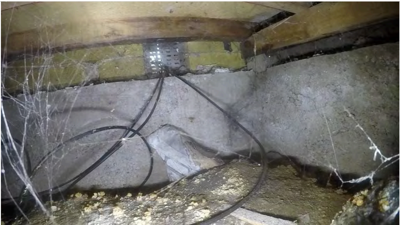
42: View of ring foundation.
