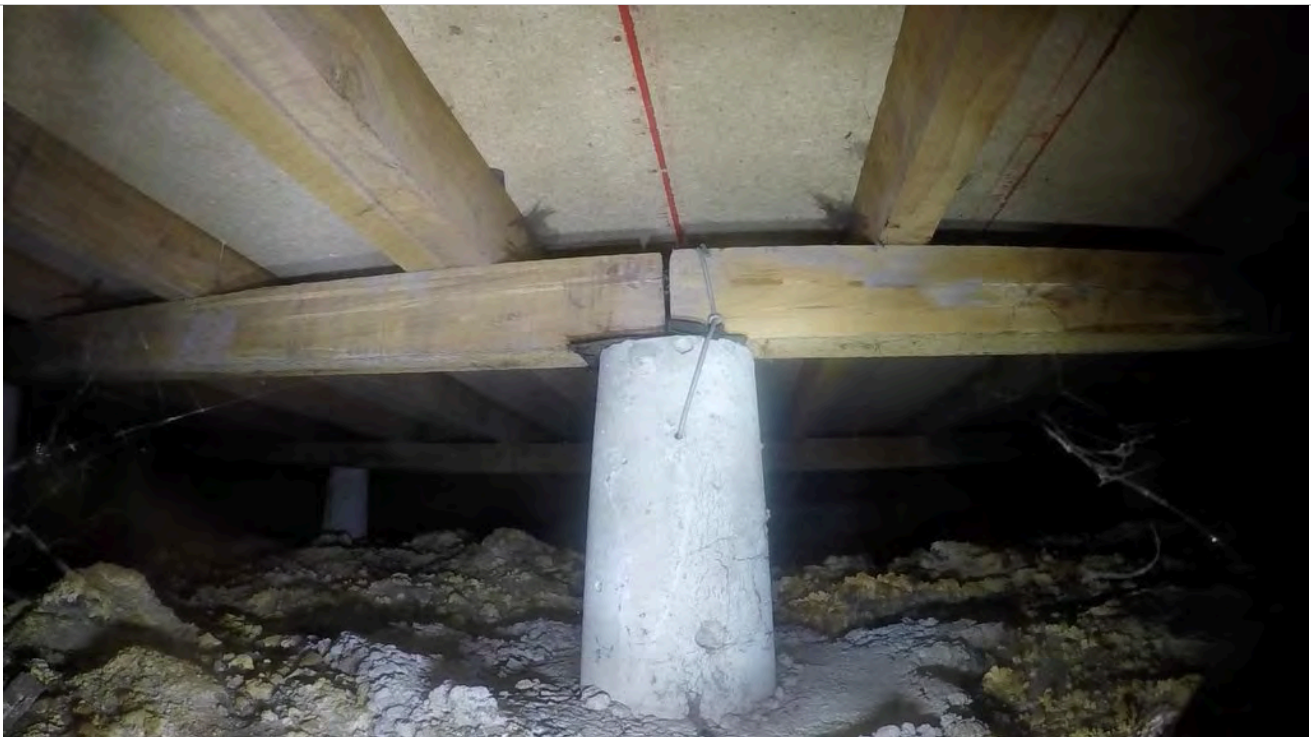
30: Pile with bearer join.
