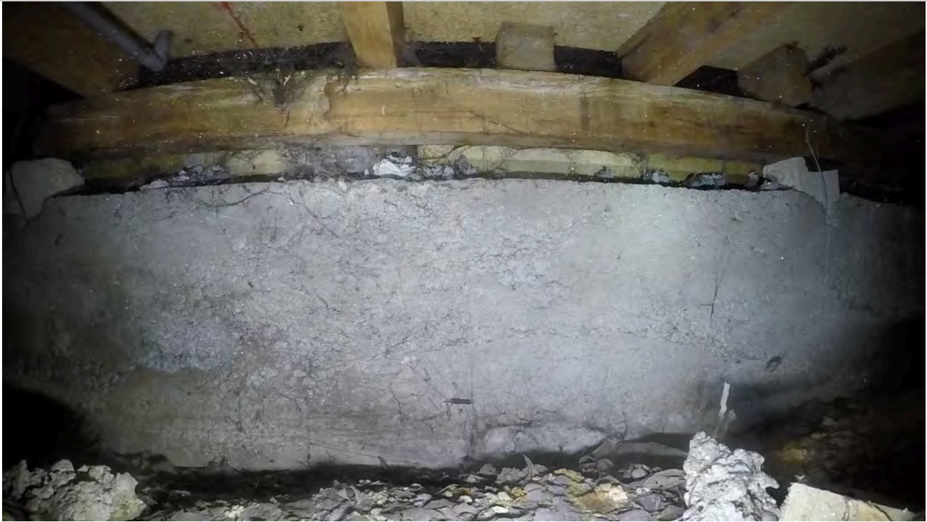
7: View of ring foundation.
