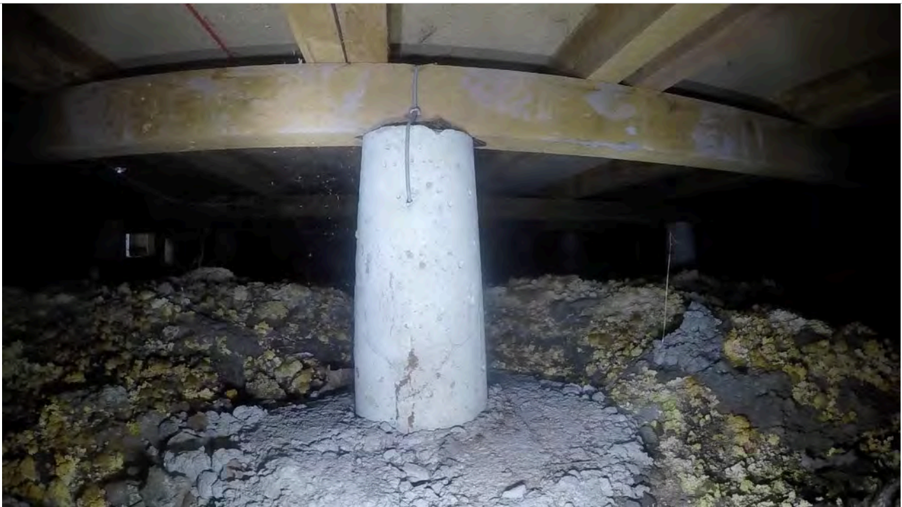
36: Pile with connection.
