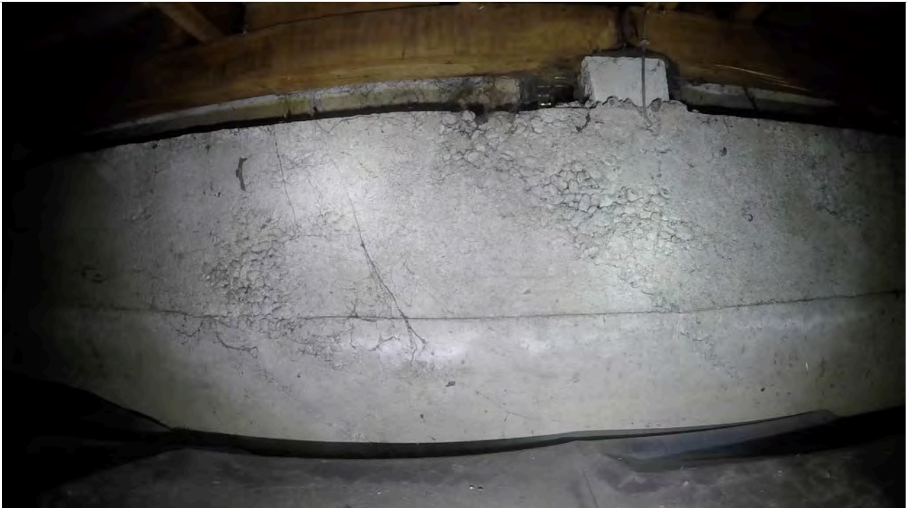
4: View of ring foundation.
