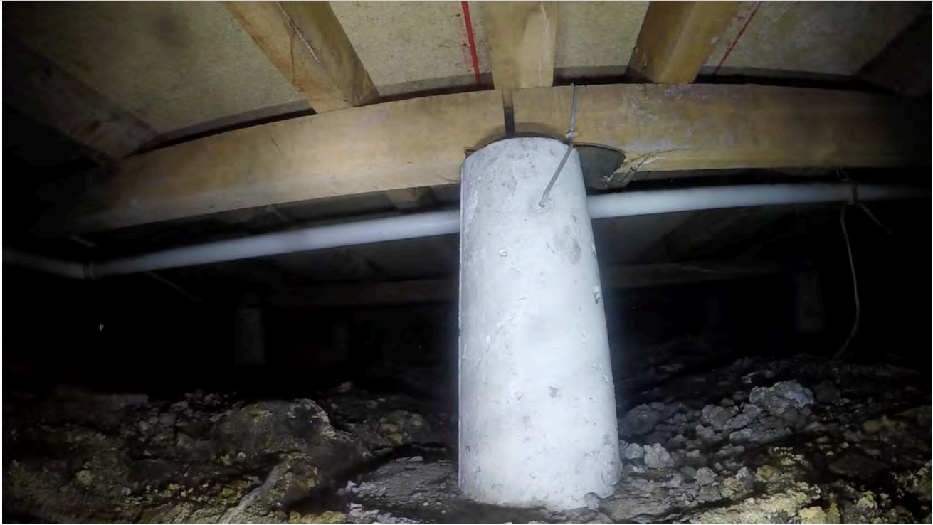
15: Pile with bearer join.
