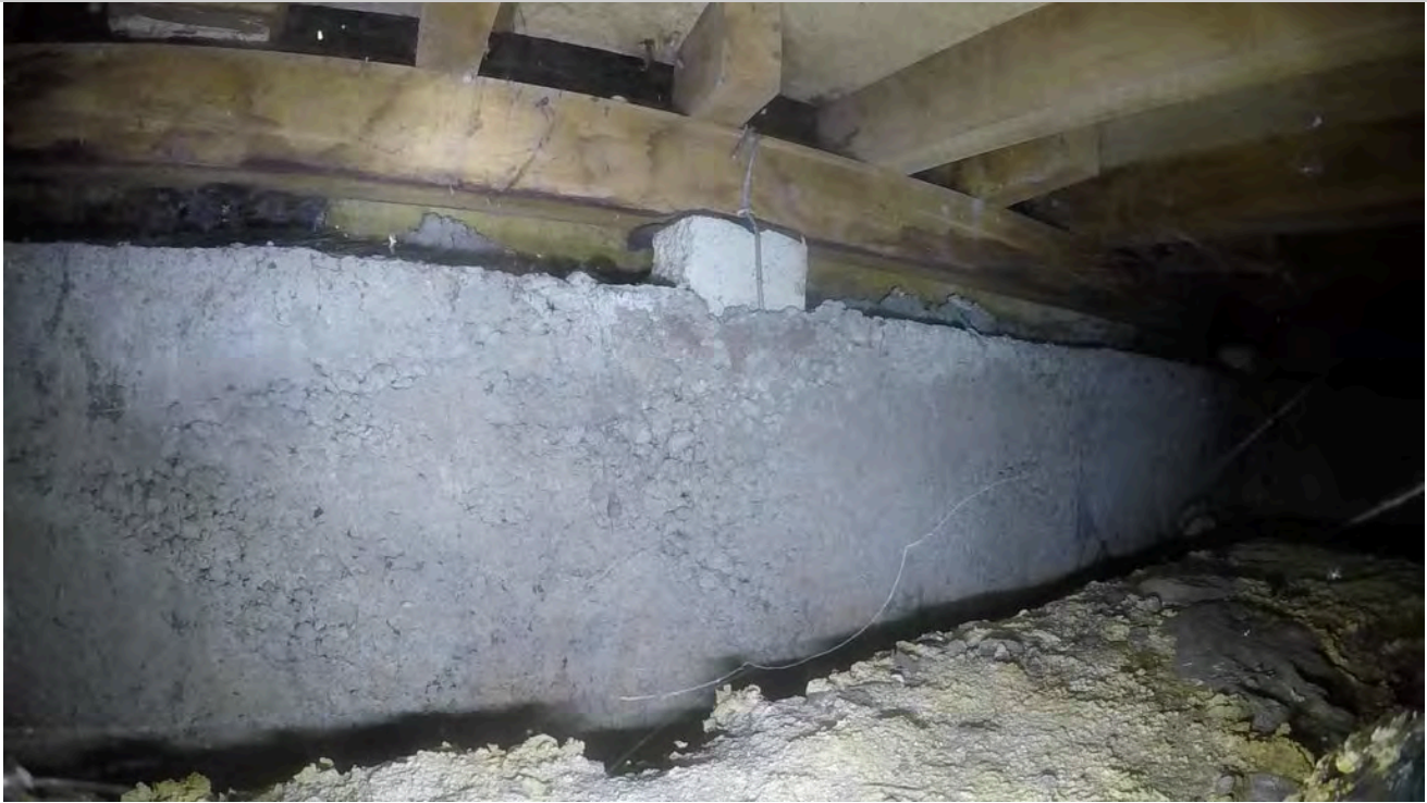
45: View of ring foundation.
