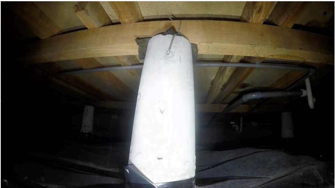
30: Pile with connection.
