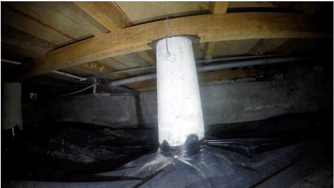
40: Pile with connection.
