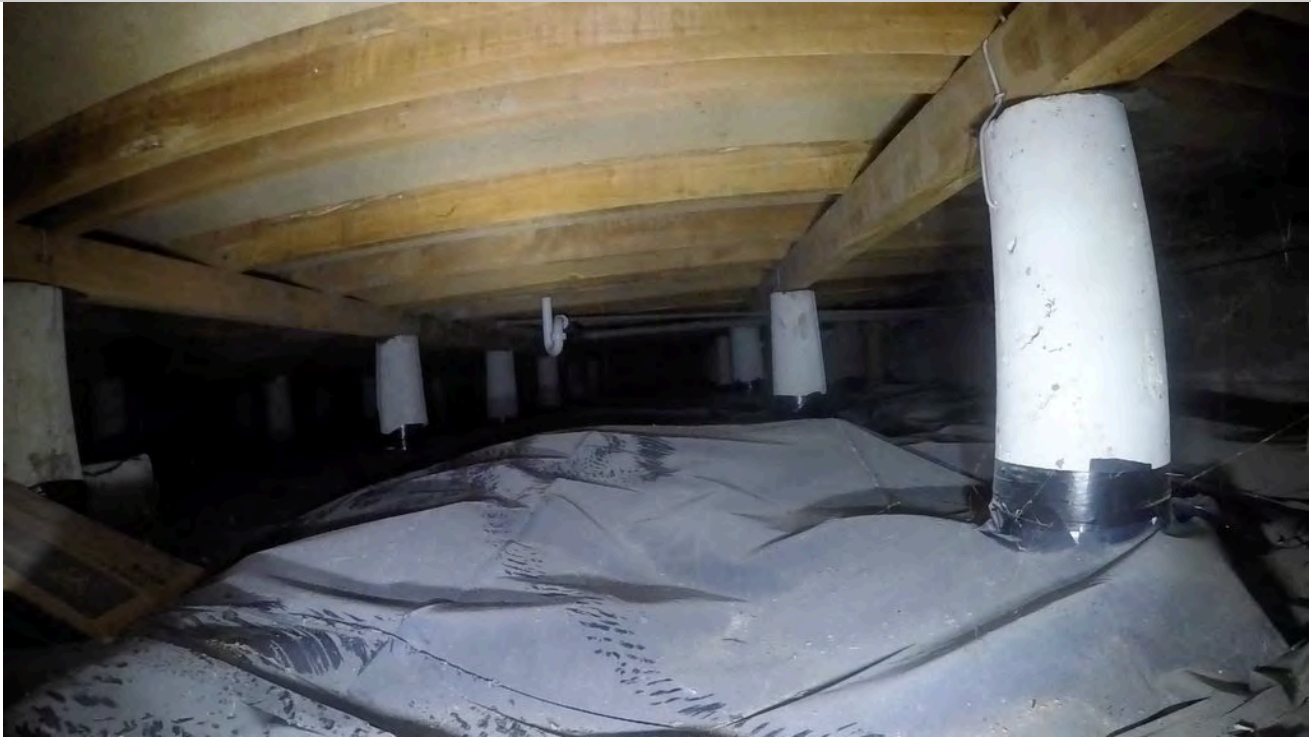
35: View along piles.
