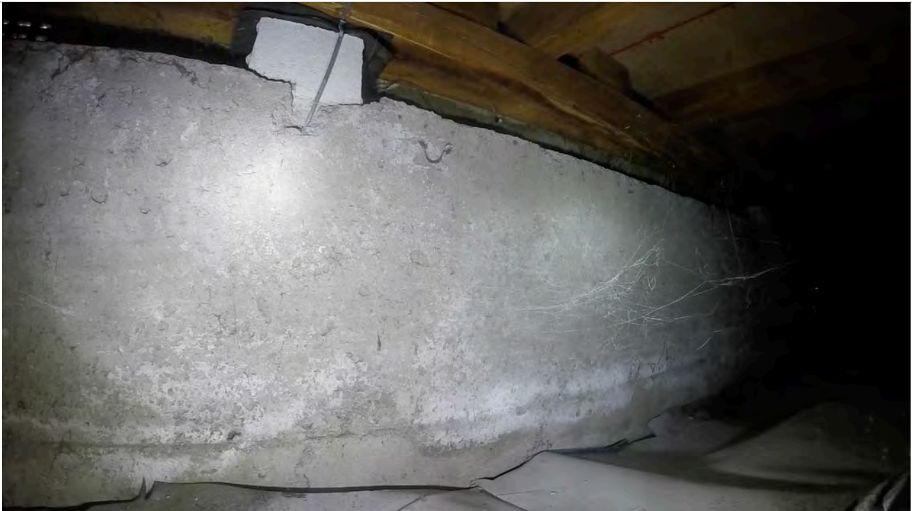
46: View of ring foundation.
