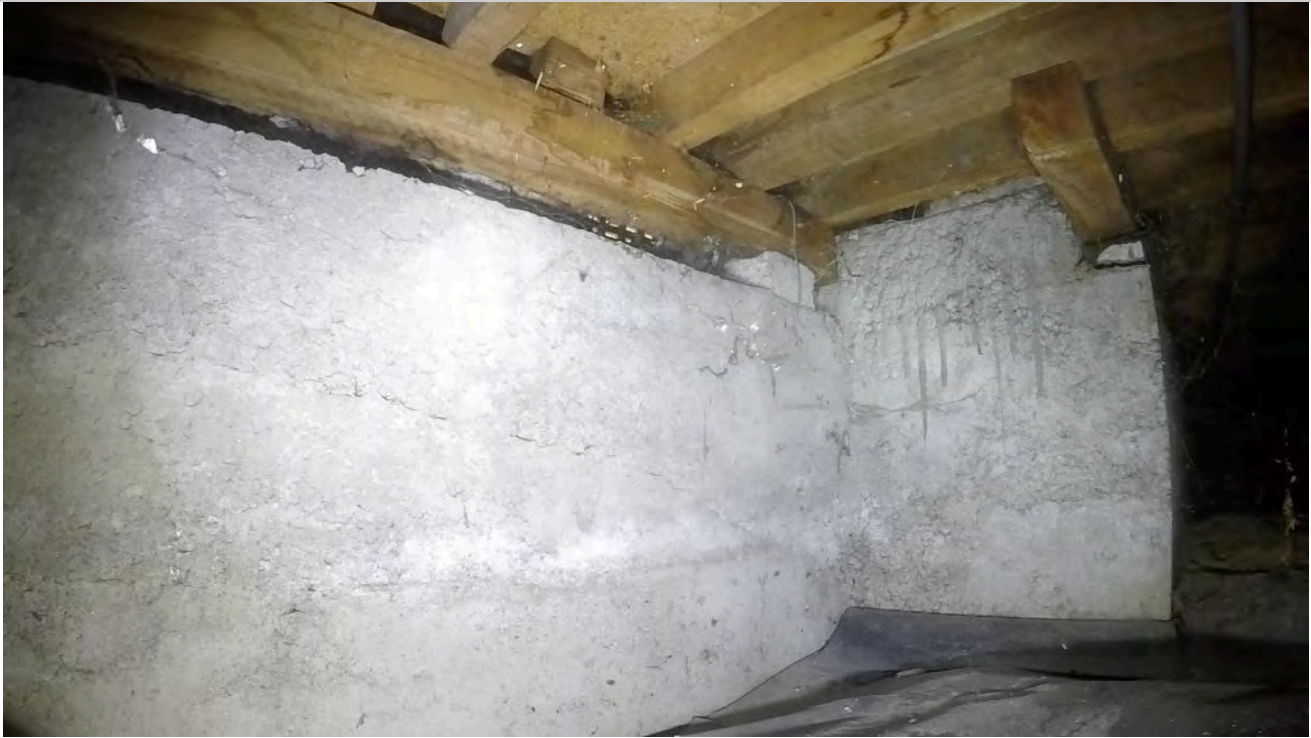
45: View of ring foundation.
