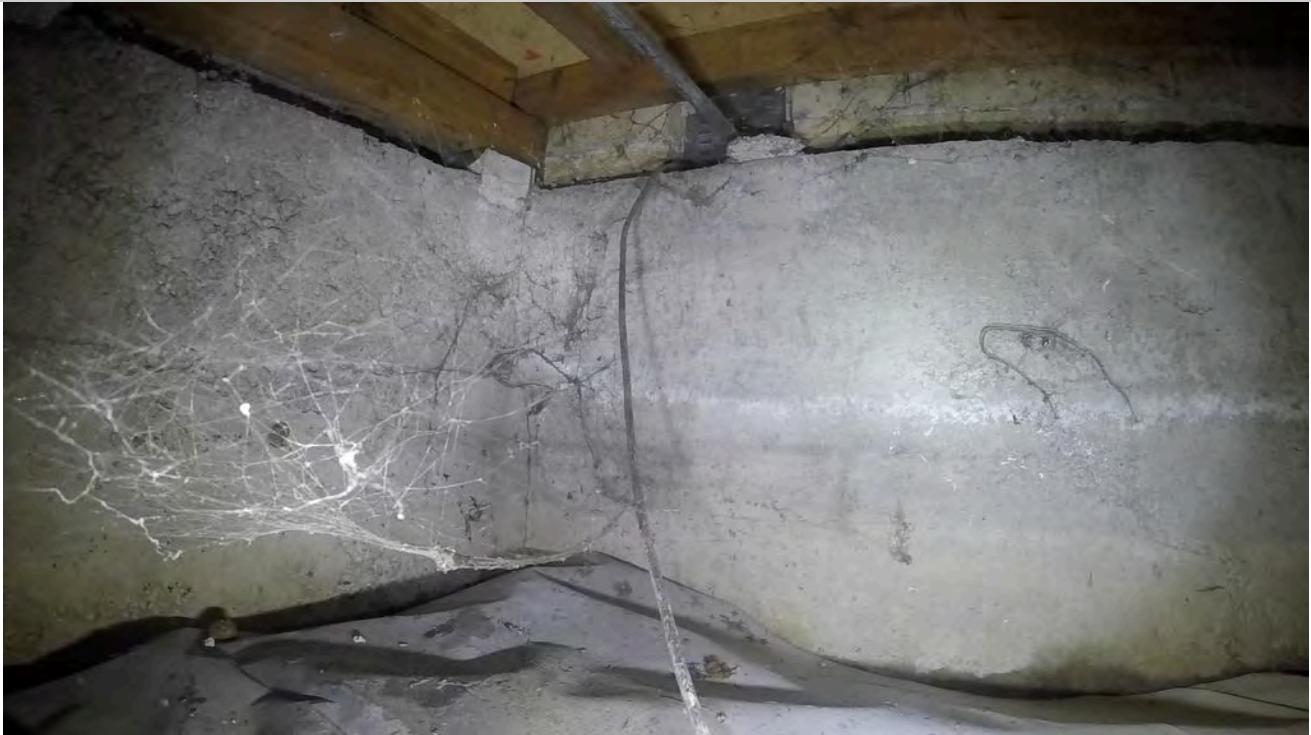
5: View of ring foundation.
