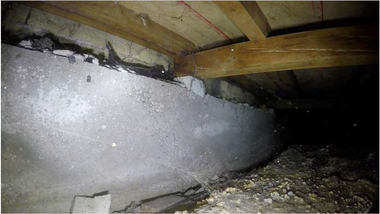
11: View of bearer meeting ring foundation with connection.
