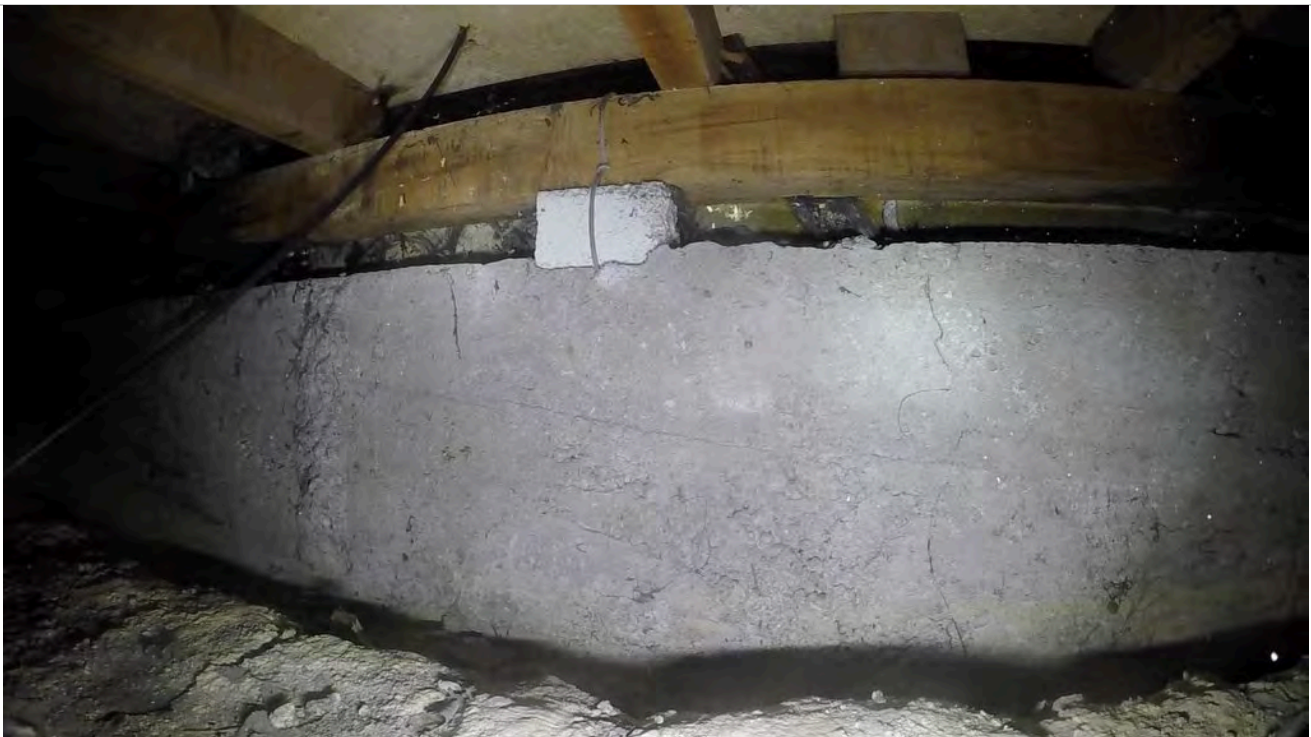
8: View of ring foundation.
