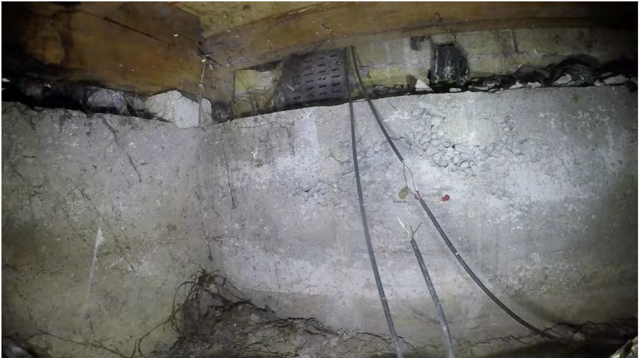
10: View of ring foundation.
