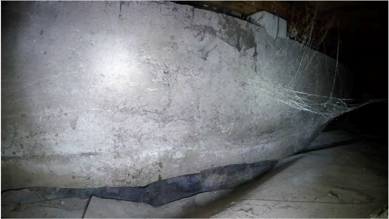
47: View of ring foundation.
