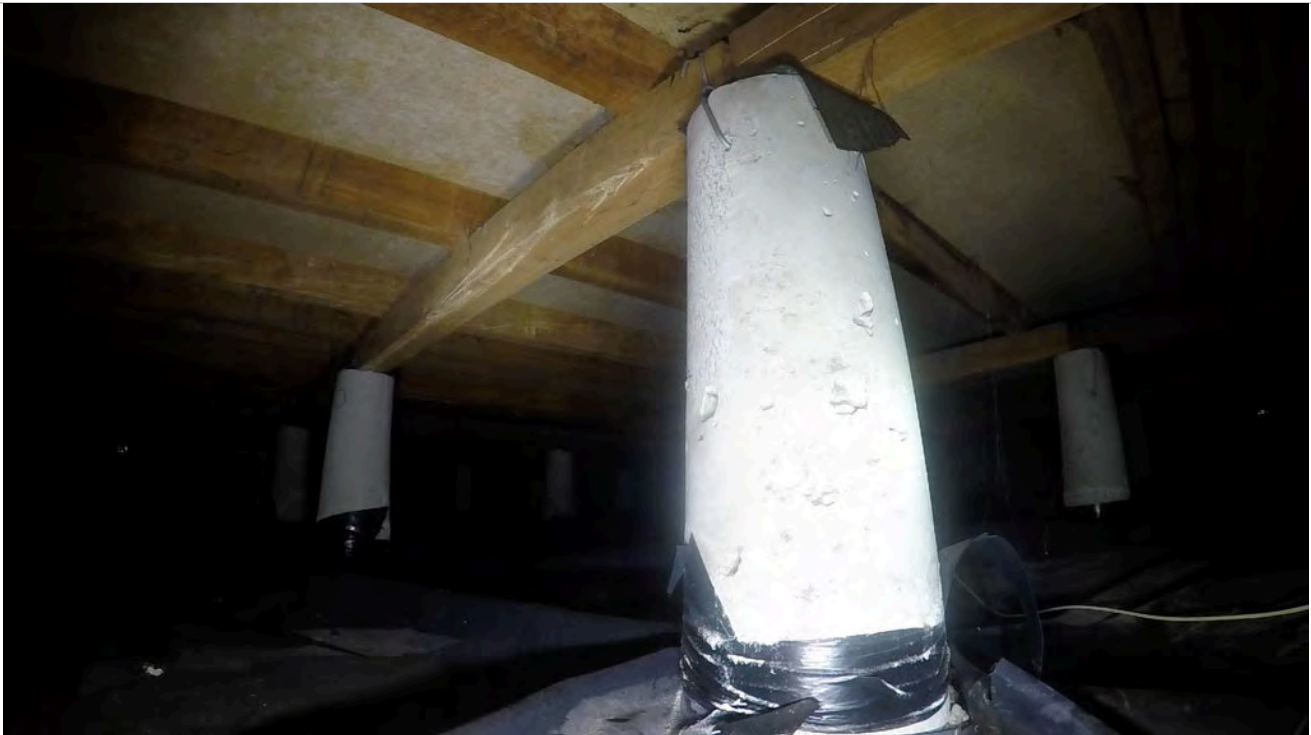
12: Pile with bearer join.
