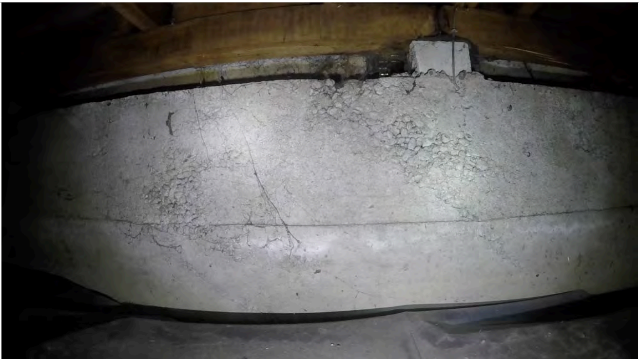
4: View of ring foundation.
