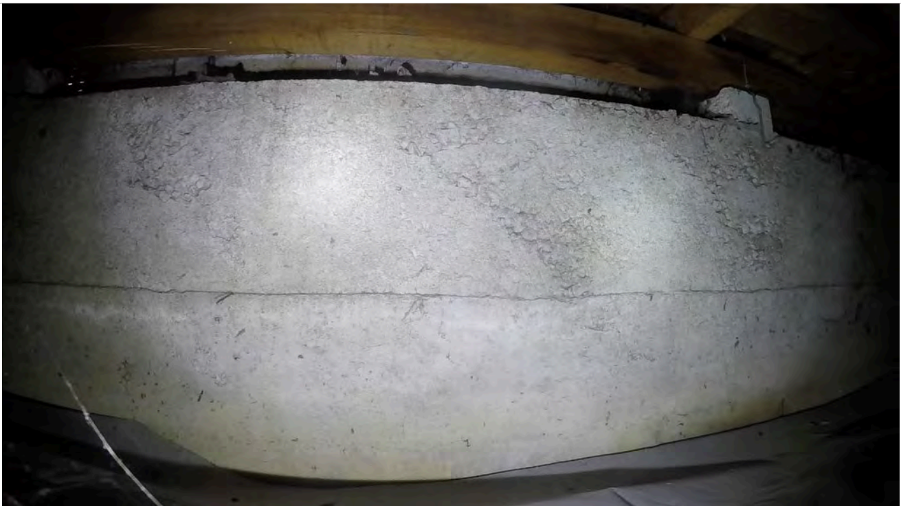
6: View of ring foundation.
