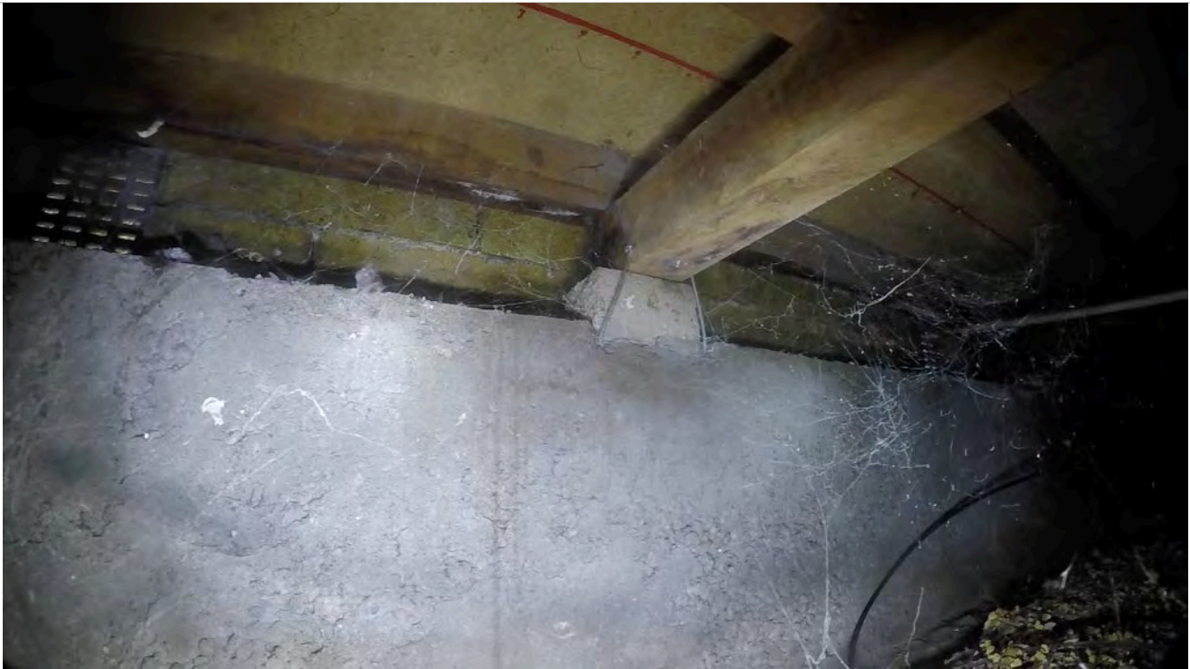
26: View of bearer meeting ring foundation with connection.
