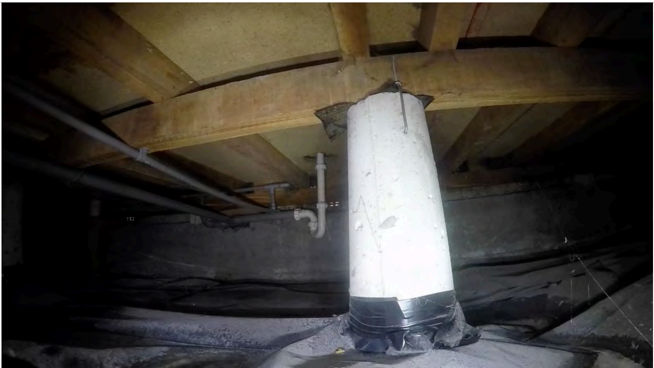
36: Pile with connection.
