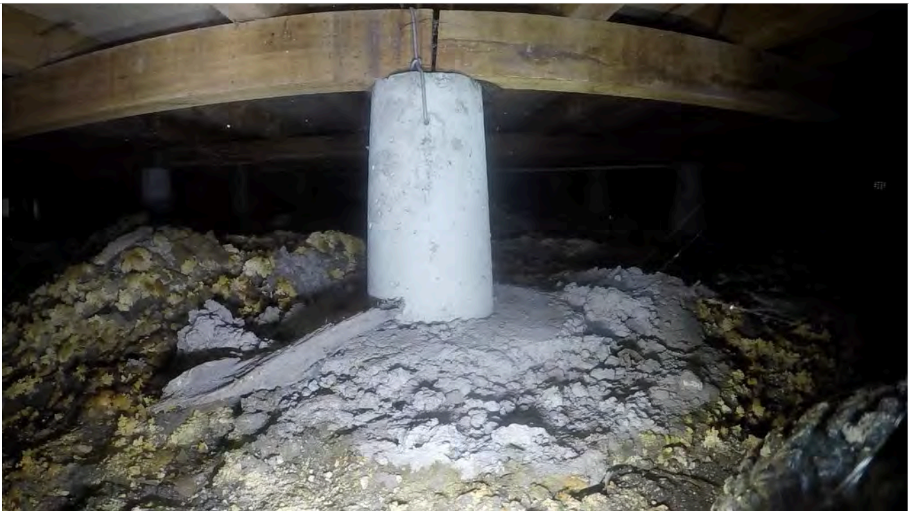
38: Pile with bearer join.
