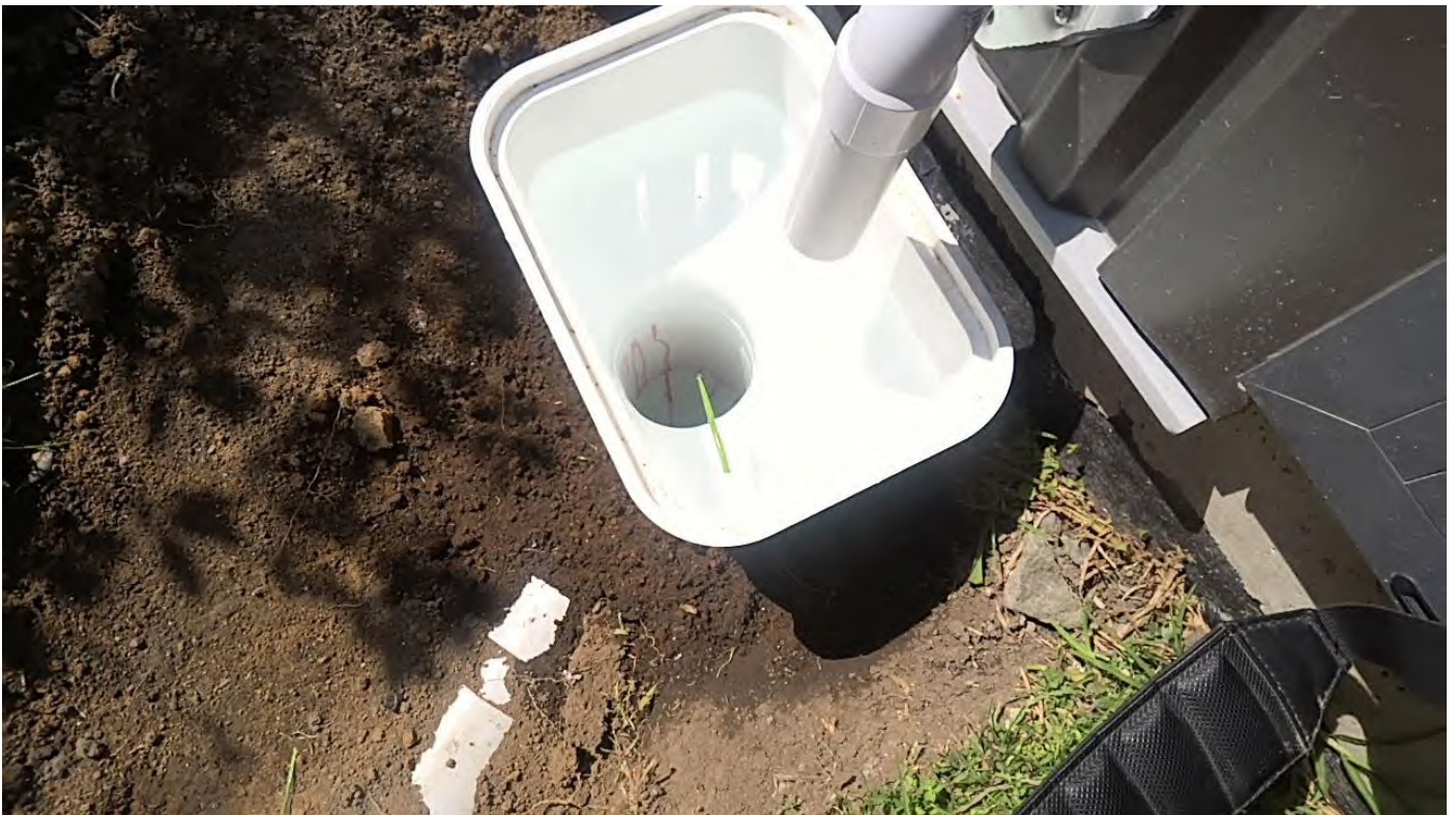
Water test complete
