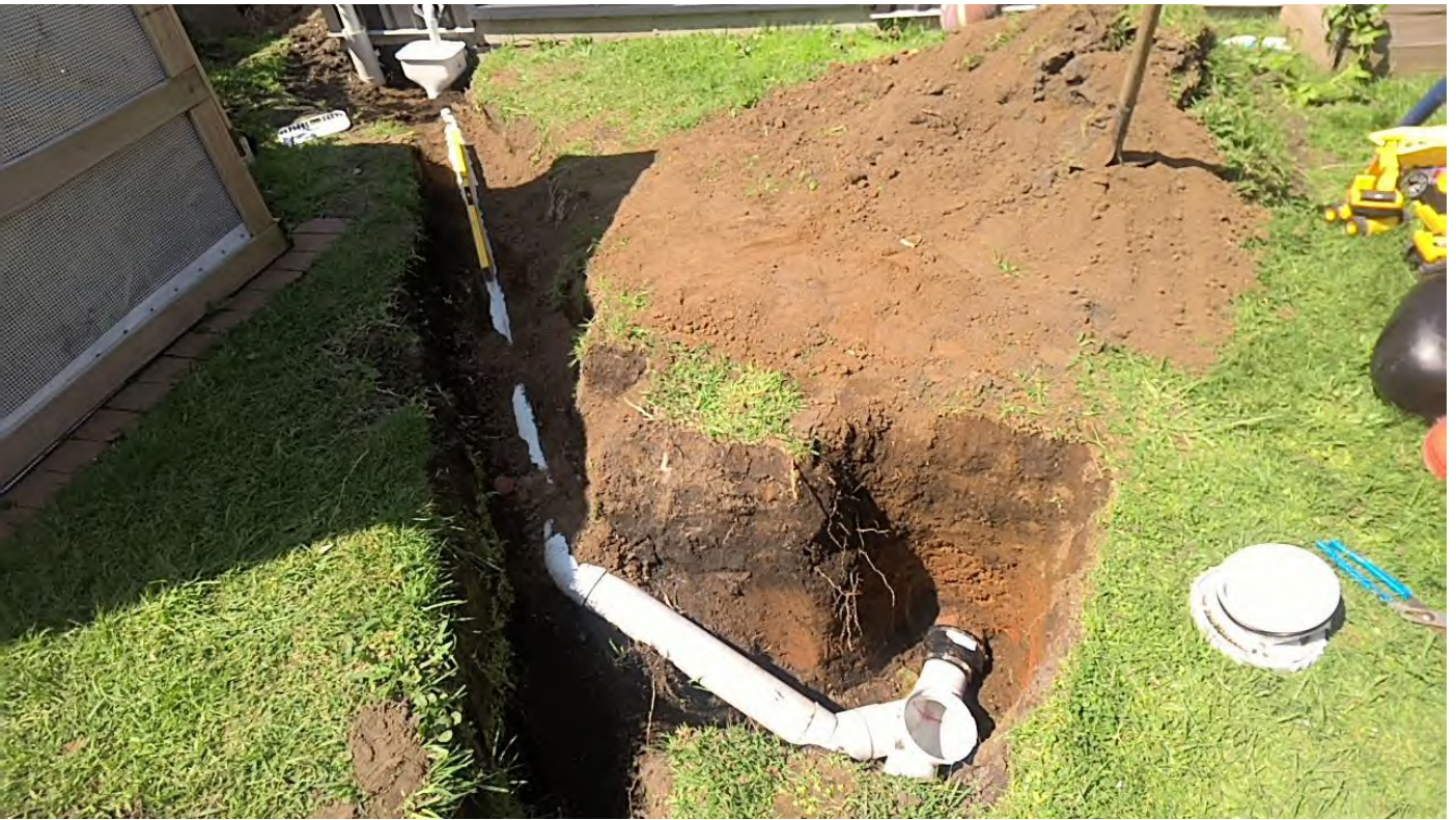
Mains connection complete
