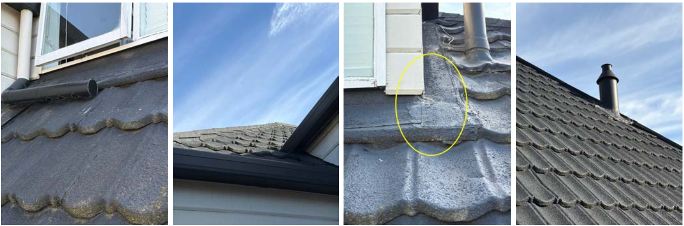
Example of junctions with sealant added to monitor for weather-tightness.
