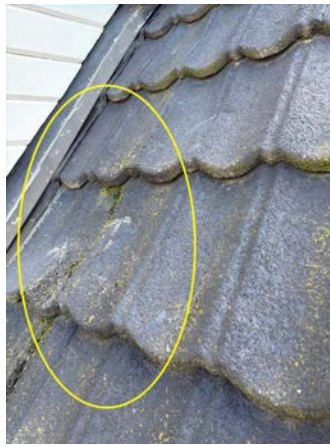
Stone chip coating aging in some areas and example of dented tiles , likely from foot traffic.
