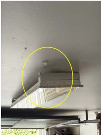
The light needs refixed to the ceiling.
