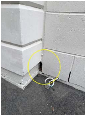
Gap noted to be filled/sealed. South face.
