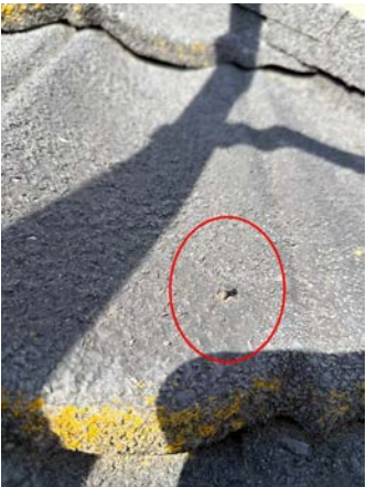
Example of popped roof cladding fixings.
