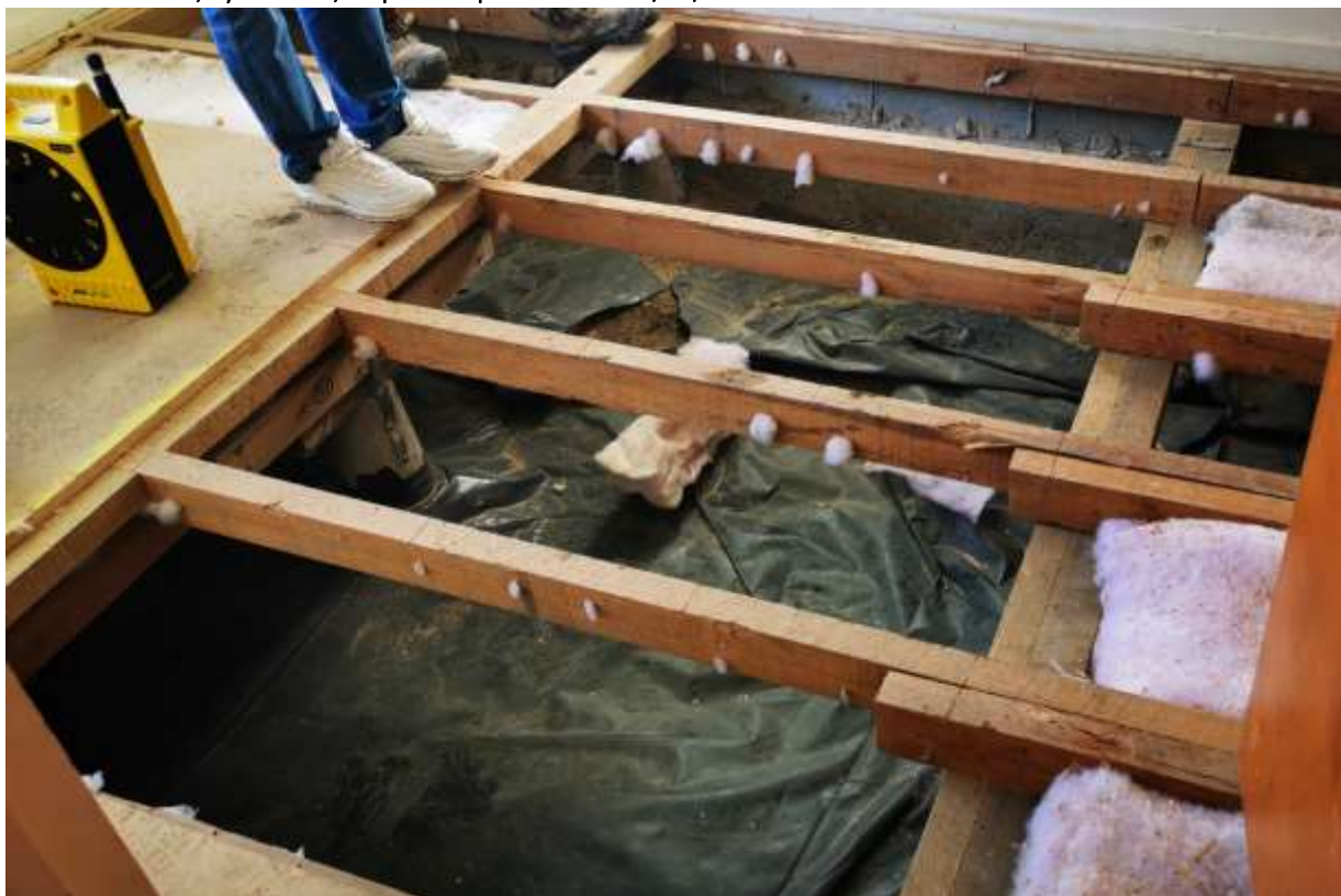
54 Devon Street, Sydenham, Inspection photos 04 – 04/07/2024
