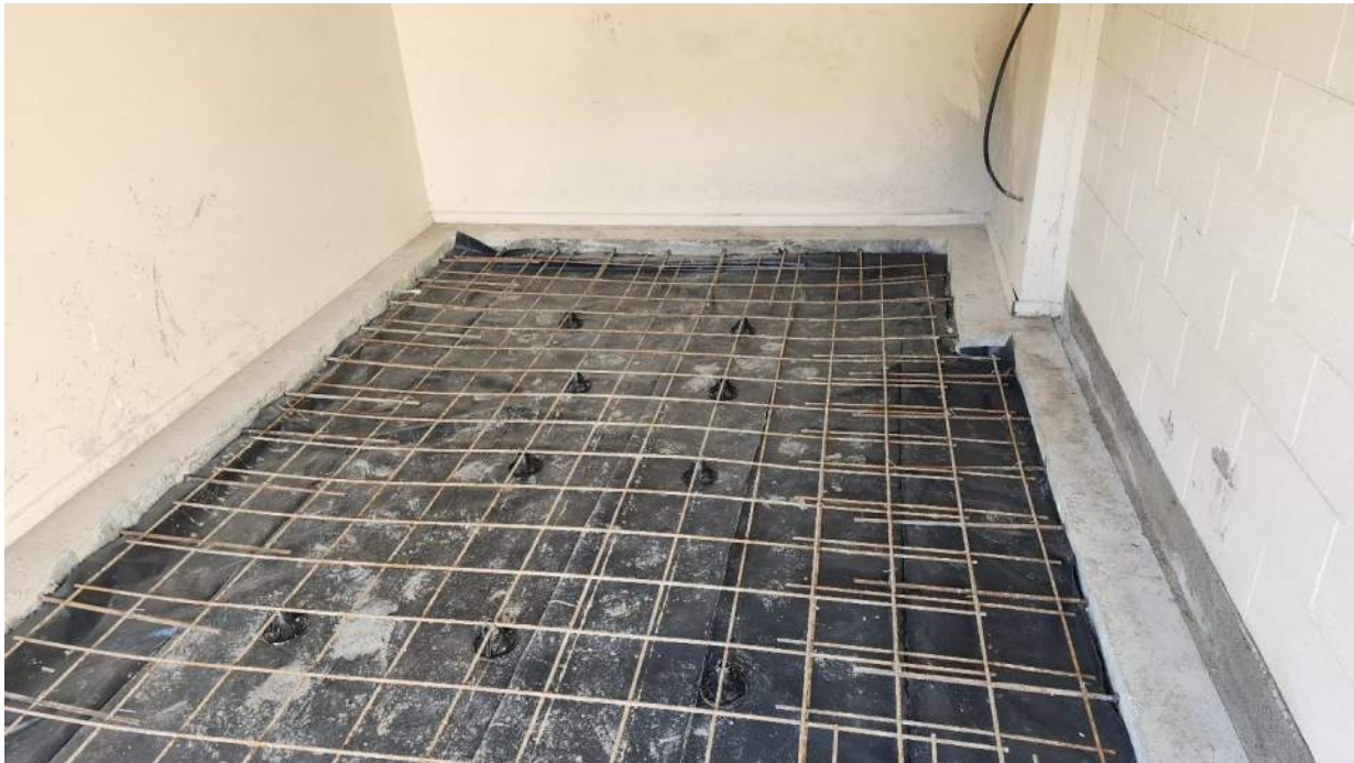
54 Devon Street Inspection photos – 24/06/2024
