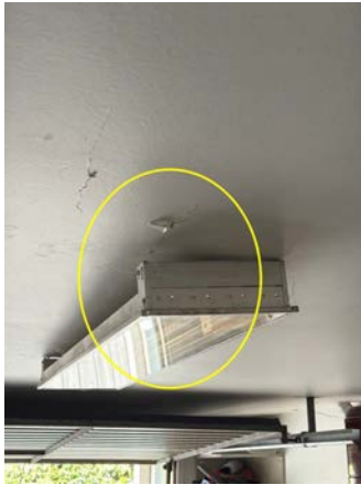
The light needs refixed to the ceiling.
