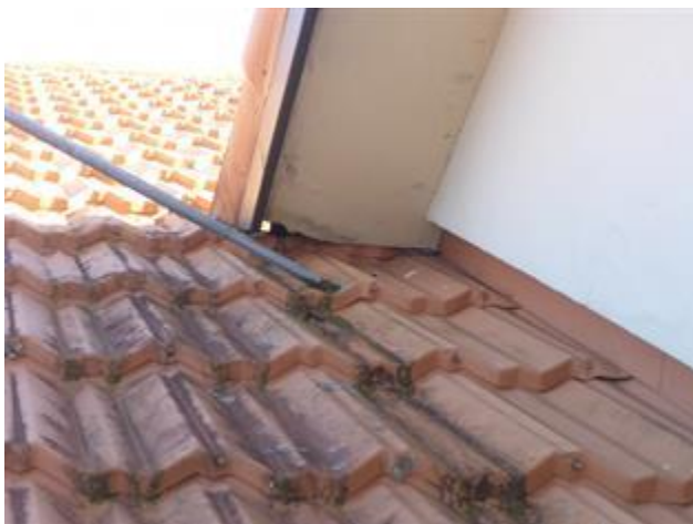
In contact/soffit deterioration
