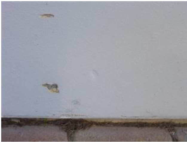
Impact damage side
