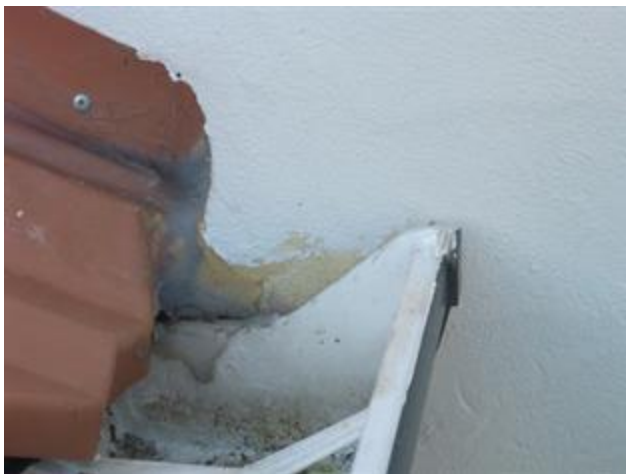
Kick out flashings recommended/ roof to wall junctions
