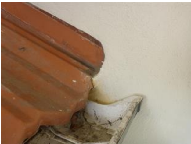
Kick out flashings recommended/ roof to wall junctions
