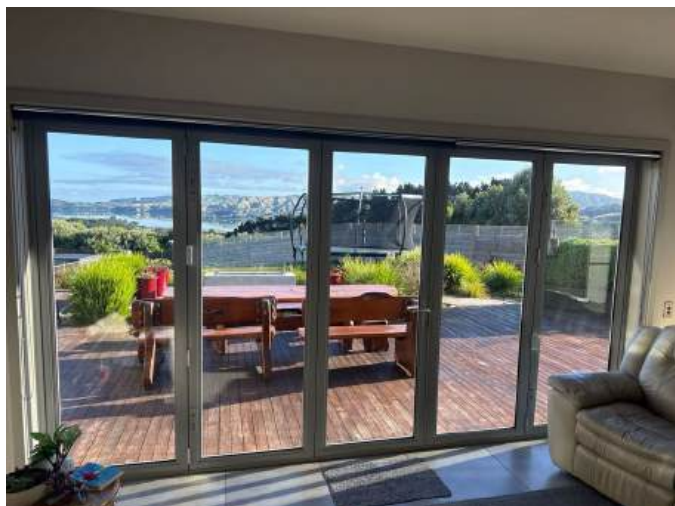
The external doors and windows are functioning
