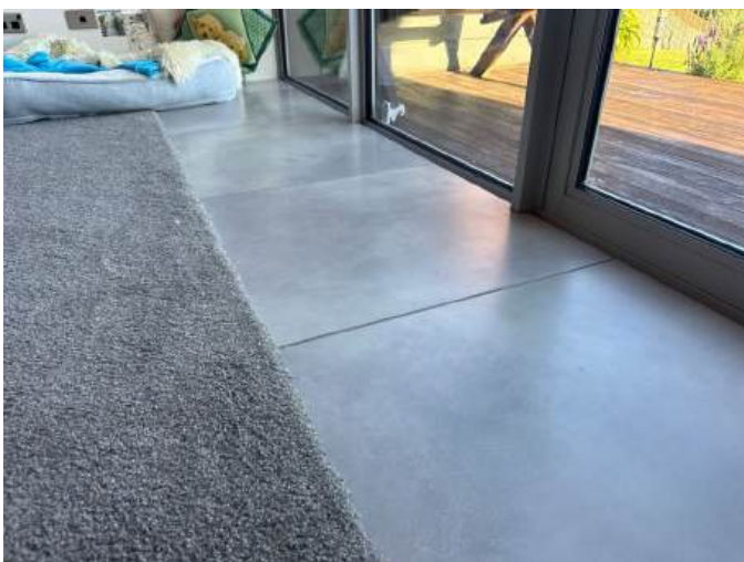
The tiles are intact and are well adhered to the floor beneath
