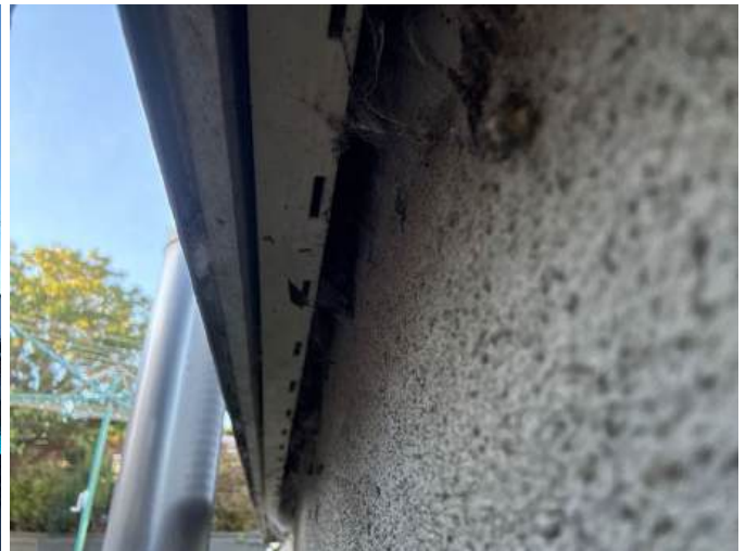
Cavity system detail clearly visible at the base of the metal cladding. The cavity system is a modern detail that allows moisture to escape and ventilation to the back of the cladding.
