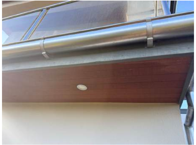
The timber fascia and soffits are in an average/good condition
