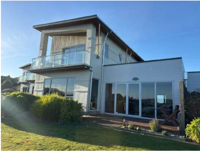
The Northwest side
