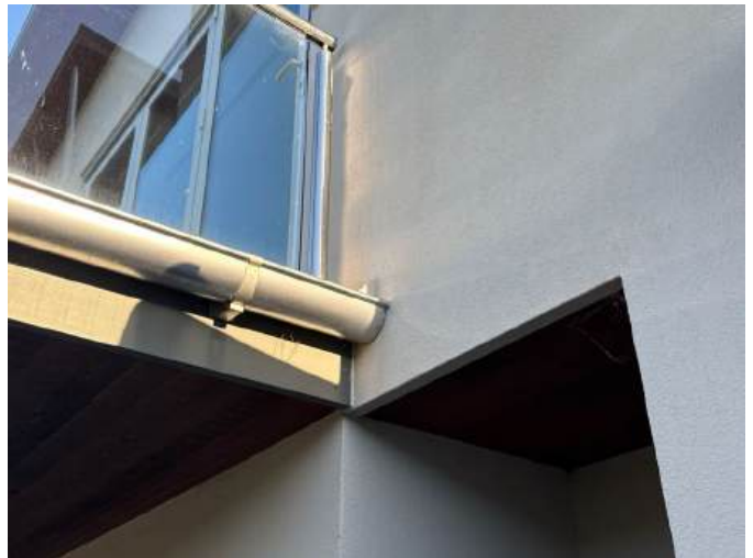
Good use of the diverter flashings at the roof/cladding junctions. These are an effective waterproofing detail that channels water away from common water tightness risk areas.
