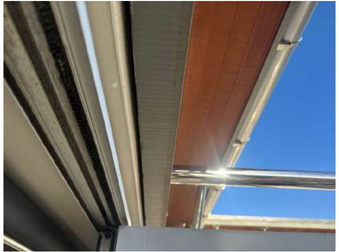
The stainless steel pergola is secure and has been installed clear of the cladding
