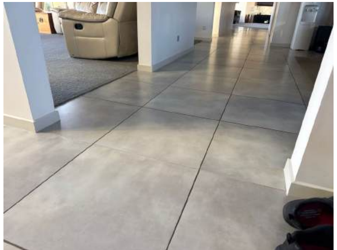
The tiles to the entrance and hallway are intact and are well adhered to the floor
