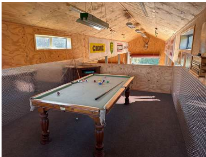
The mezzanine floor area is in good condition
