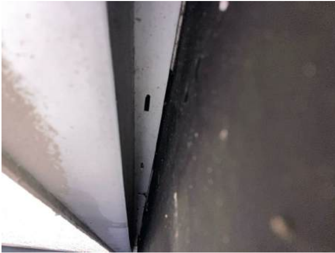
Vented cavity system identified beneath the parapets
