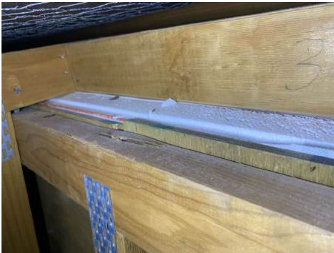
Ceiling cavity. The EIFS cladding has a plywood base at the upper level at least. T.H.I.S was unable to confirm the presence of plywood at all locations as it is mostly concealed. The council file will note this. The plywood sheets will provide bracing to the structure and an additional waterproofing layer.
