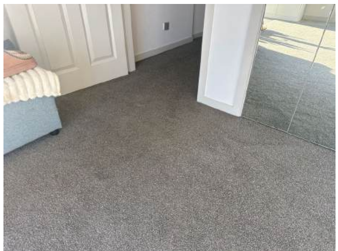
The condition of the internal linings and carpet is good
