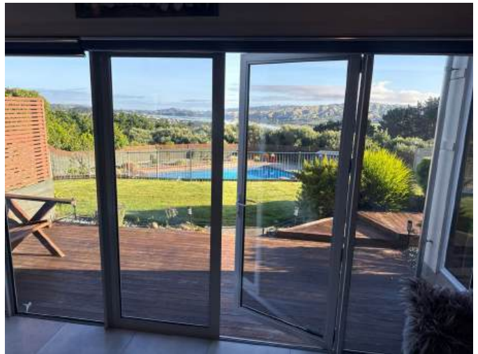
The external doors are functioning well
