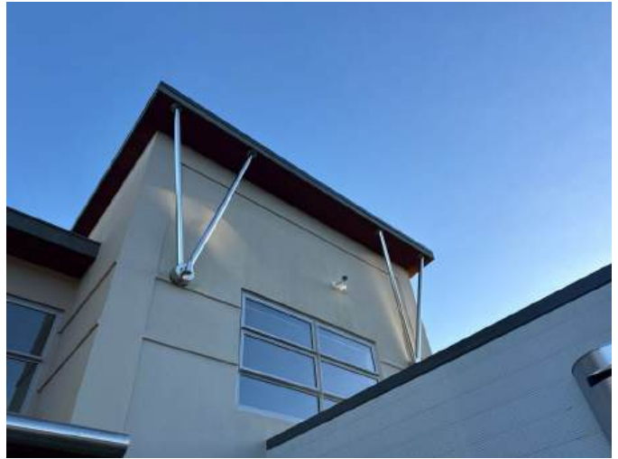
The stainless steel supports are secure
