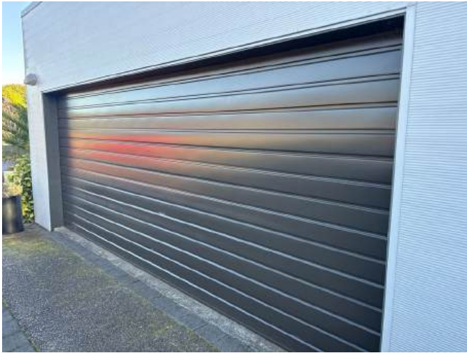
The surface condition of garage door #1 is good (new)
