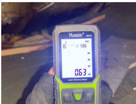
Subfloor height View High Resolution Image Here
