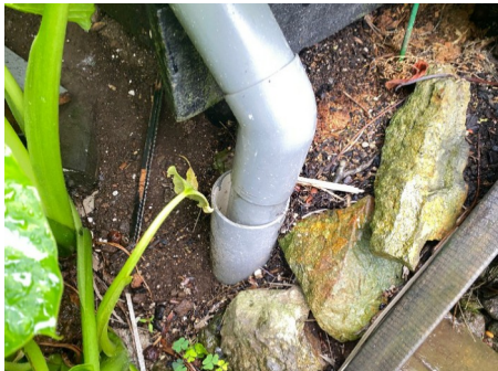
Front of property - downpipe Downpipe leads to an appropriate outfall. View High Resolution Image Here
