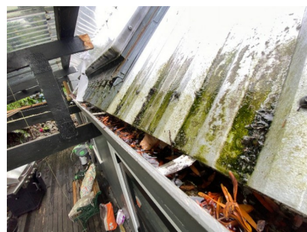
Rear of property - spouting Spouting is blocked by plants or debris preventing effective drainage. View High Resolution Image Here
