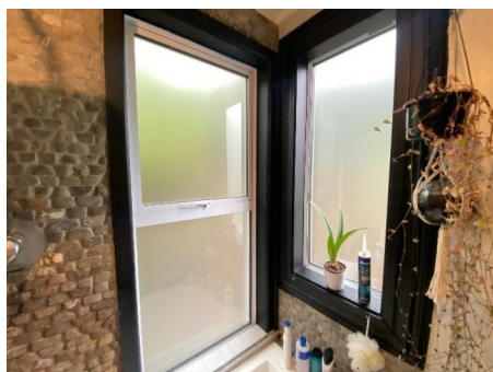
Bathroom The window is compliant for draught stopping. View High Resolution Image Here
