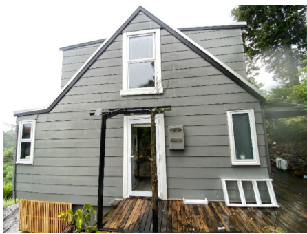
Subfloor surrounds - Right side of property Context View High Resolution Image Here
