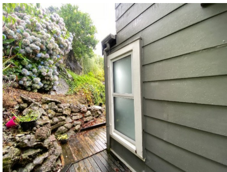
Rear of property - downpipe Downpipe is in good condition/ or near new condition and affixed securely to building. View High Resolution Image Here
