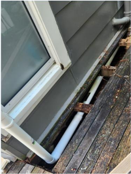
Drainage remediation View High Resolution Image Here 02/02/2026
