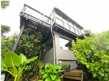
Front of property - downpipe Downpipe is in good condition/ or near new condition and affixed securely to building. View High Resolution Image Here
