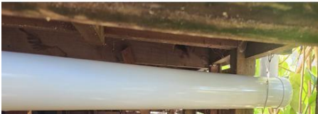
Drainage remediation View High Resolution Image Here 02/02/2026
