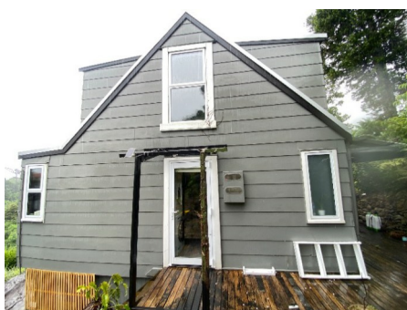
Right side of property - gable end No spouting system installed and not required. View High Resolution Image Here
