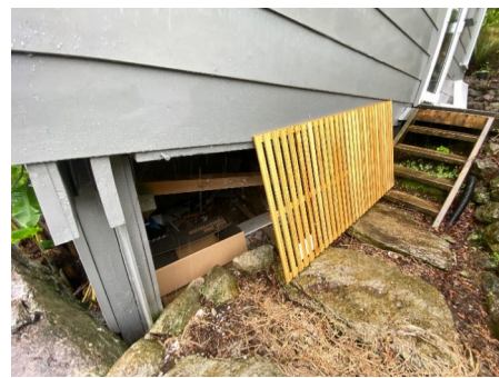
Subfloor access Right side of the property View High Resolution Image Here
