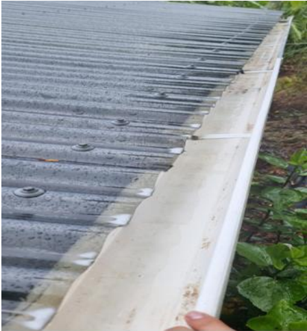
Drainage remediation View High Resolution Image Here 02/02/2026
