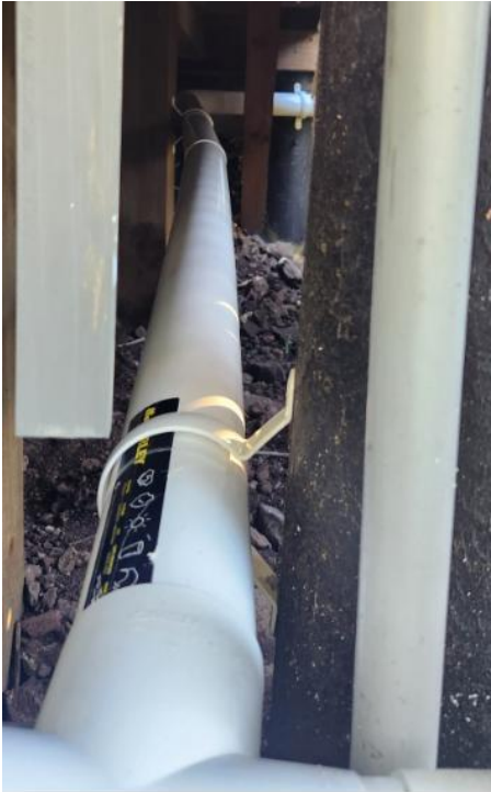
Drainage remediation View High Resolution Image Here 02/02/2026
