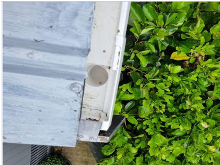
Drainage remediation View High Resolution Image Here 02/02/2026
