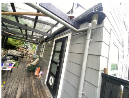
Rear of property - spouting Spouting system is in good condition/ or near new condition. View High Resolution Image Here
