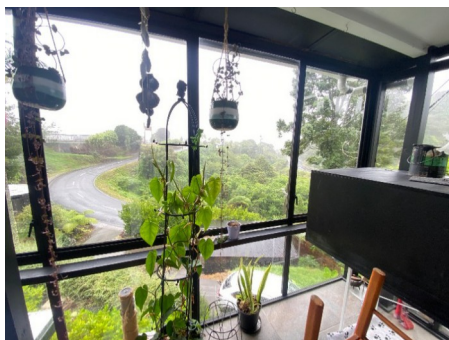
Conservatory The window is compliant for draught stopping. View High Resolution Image Here
