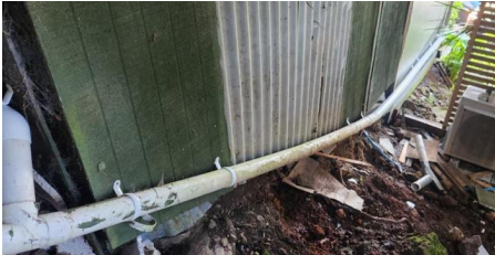
Drainage remediation View High Resolution Image Here 02/02/2026
