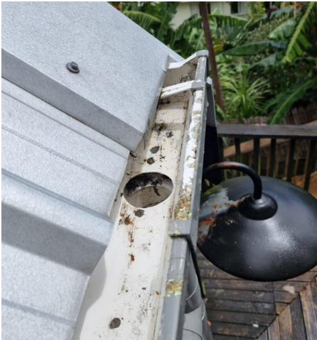
Drainage remediation View High Resolution Image Here 02/02/2026
