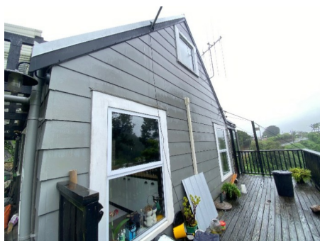
Left side of property - gable end No spouting system installed and not required. View High Resolution Image Here
