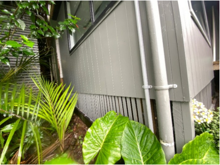
Subfloor surrounds - Left side of property Context View High Resolution Image Here
