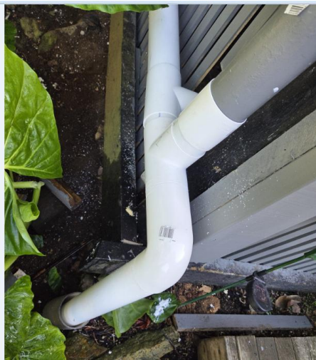
Drainage remediation View High Resolution Image Here 02/02/2026
