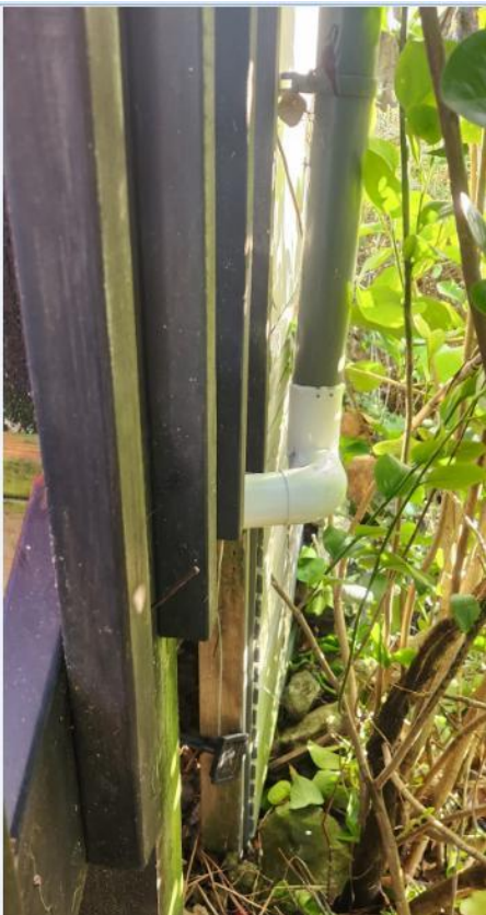
Drainage remediation View High Resolution Image Here 02/02/2026
