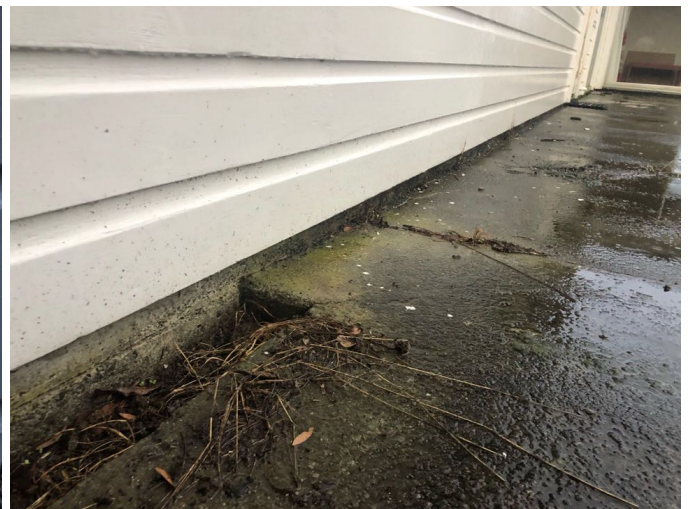
Modern concrete floor slab with a vapour barrier installed at the time of construction.
