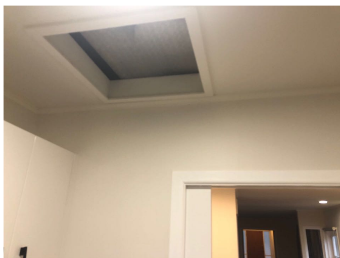
Insulation and ceiling cavity viewed from this access point.
