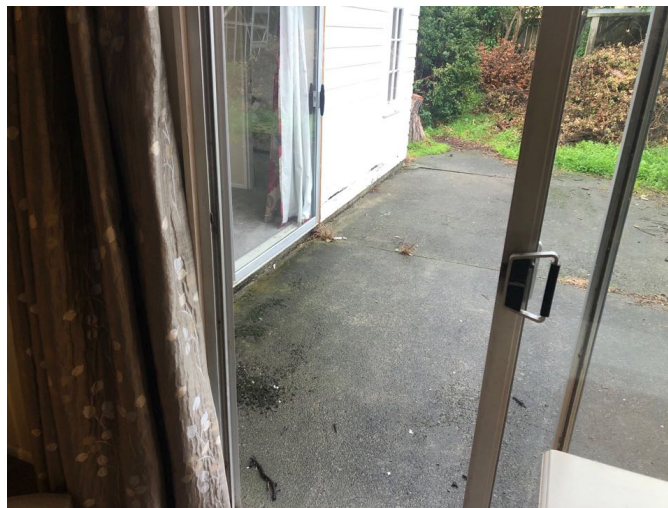
The openable doors comply with the 5% ventilation requirement for this room and section 21 of the Healthy Homes Standard.
