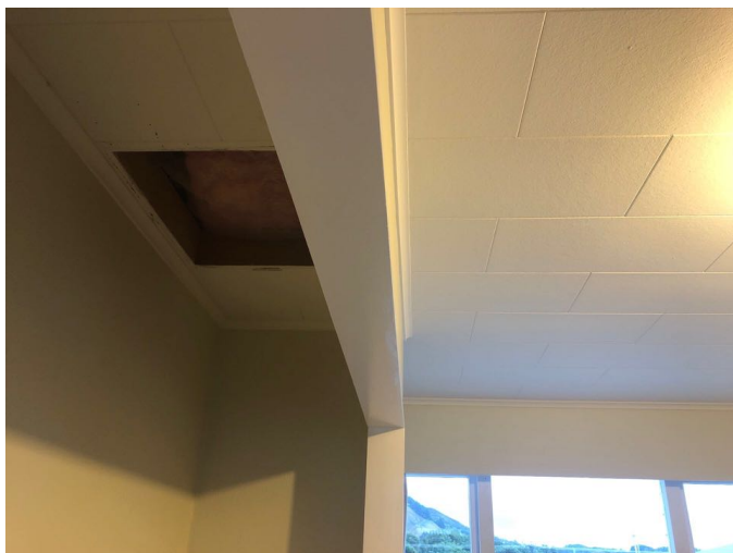
Ceiling insulation viewed from this access point.
