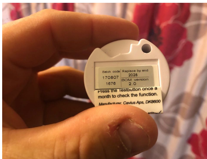
Qualified smoke detector noted and tested. Expiry 2028
