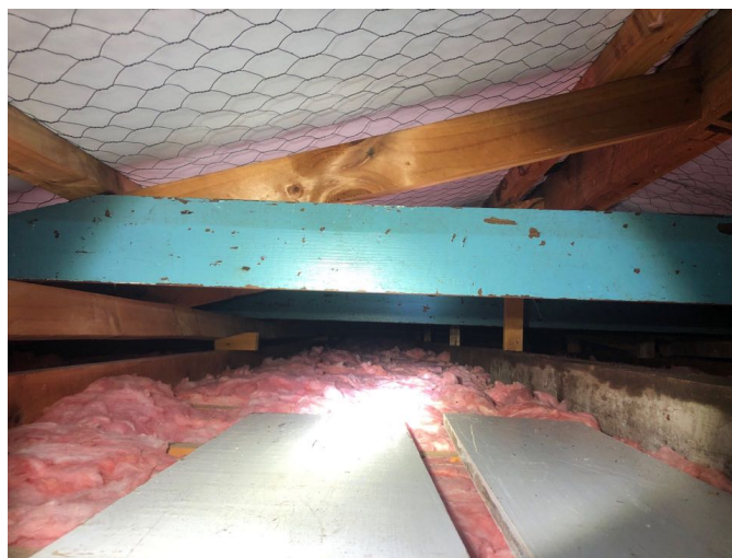
The Ceiling areas appear sufficiently insulated with R3.2 fibreglass batts to meet the insulation requirements for the Healthy Homes Standards.
