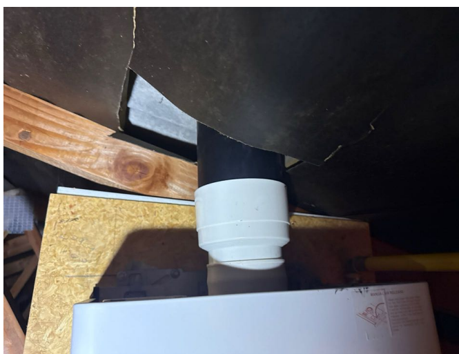
The roof penetrations were effectively sealed at the time of the inspection
