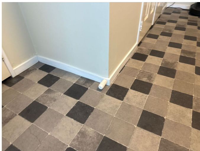
The wall linings and vinyl flooring are tidy
