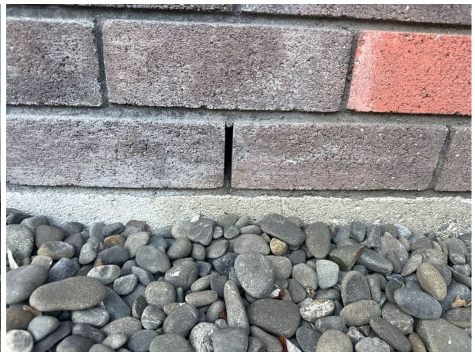
The brick facade has a cavity and weep hole detail which allows ventilation and drainage to and from the cavity behind the bricks. Weep holes and ventilation gaps must be kept clear for this to be effective.
