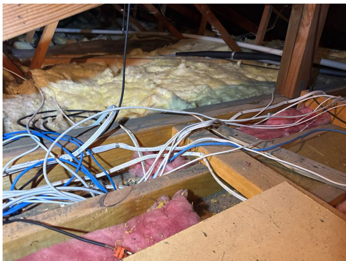
The insulation is a combination of loose fill and batts
