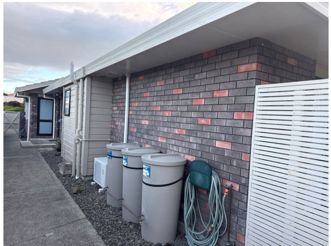
The Southwest side
