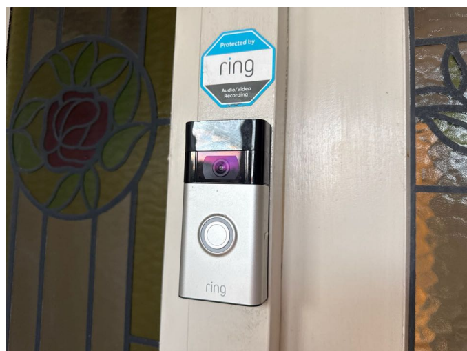
Security camera/door bell installed at the front entrance - untested
