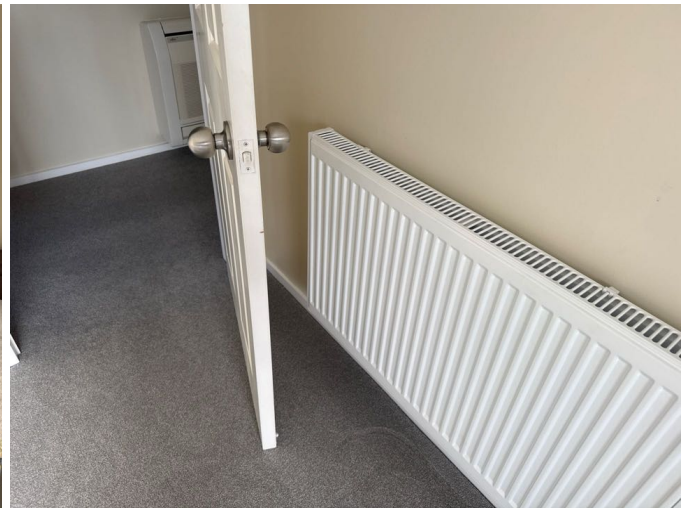
The internal doors are functioning well. Door stops installed behind the doors. Door stops should be installed where missing to prevent the door hitting the radiator.
