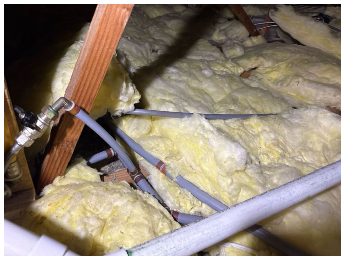
There was no evidence of plumbing failure found at the time of the inspection
