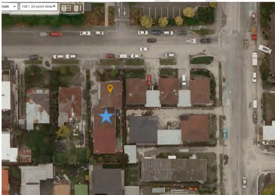
Figure 3: Aerial photo taken 24 Feb. 2011; note liquefaction deposits on driveway and nearby
