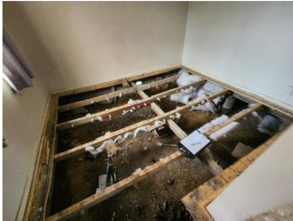
Figure 6: View of the sub-floor space at the northeast corner of the dwelling
