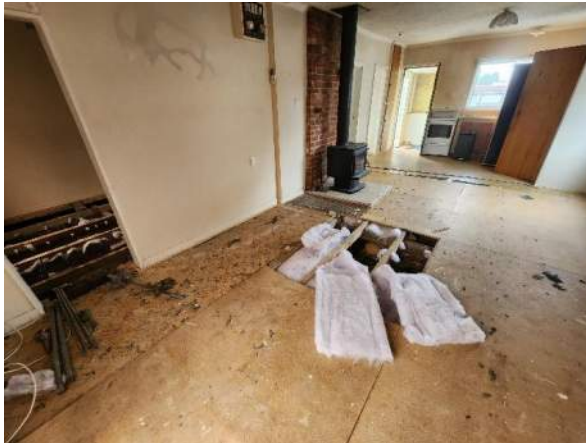
Figure 12: View of the lifted floorboards in the lounge area (below this void is the fill material shown in Figure 7)
