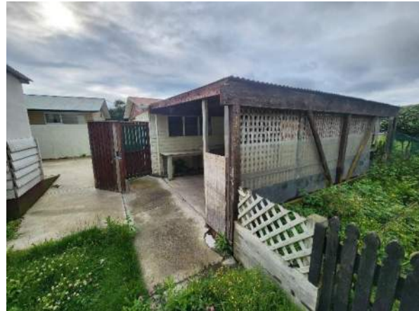
Figure 13: View of the detached garage/lean-to from southwest of the dwelling looking southeast
