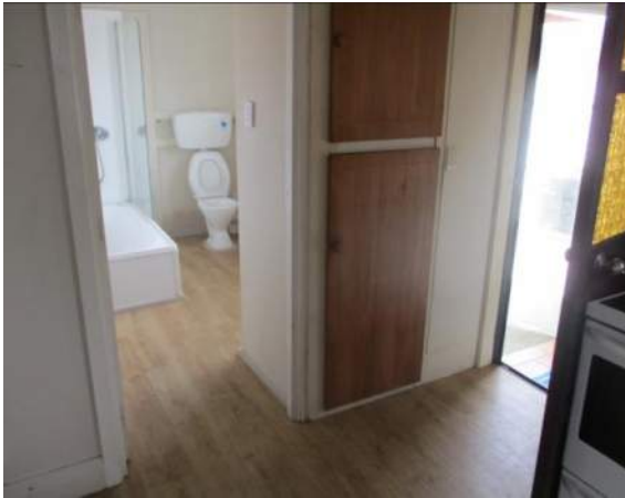
Kitchen to bathroom
