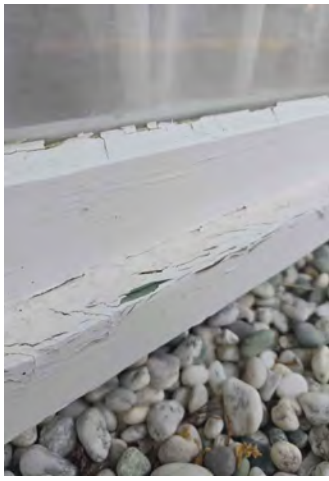
An example. Paint flaking noted.
