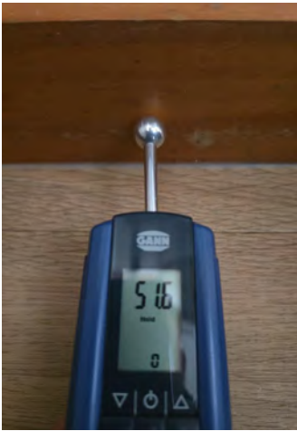
Under the toilet connection water pipe.
