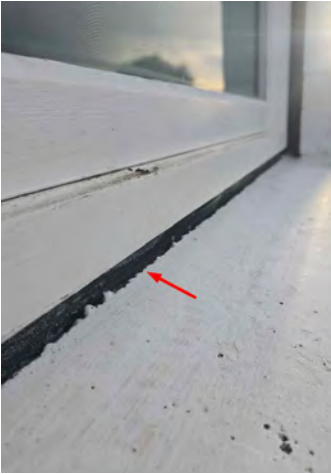
Missing sealant.
