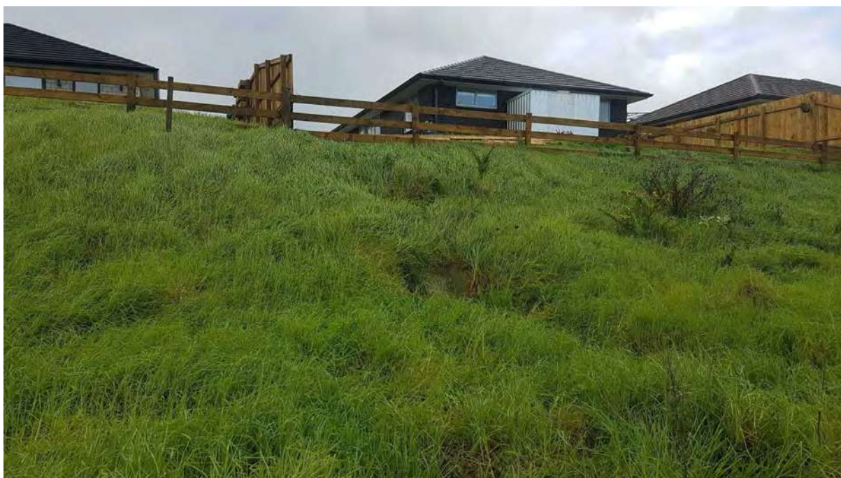
Figure 4-4: Stormwater Outlet on Slope Below Southern Stage 2
