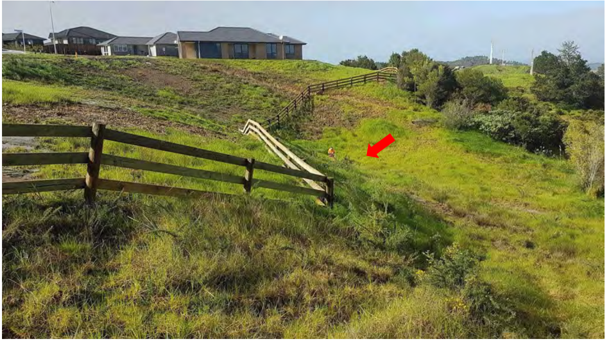
Figure 4-1: Northern Stage 2 Looking South. Arrow shows approximate Tension Crack Location
