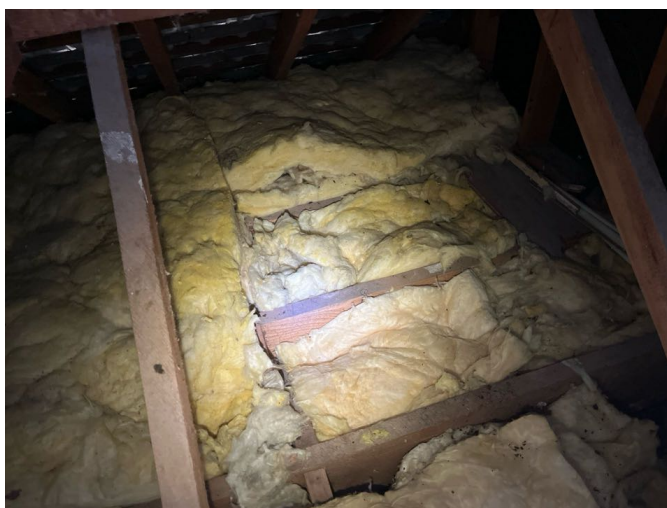
Ceiling areas well covered.
