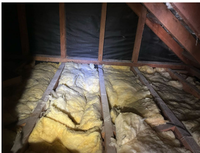
Ceiling areas well covered.
