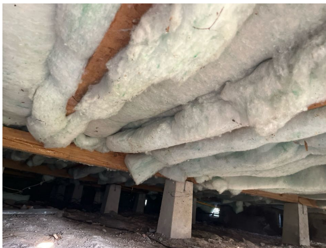
Underfloor areas well covered.
