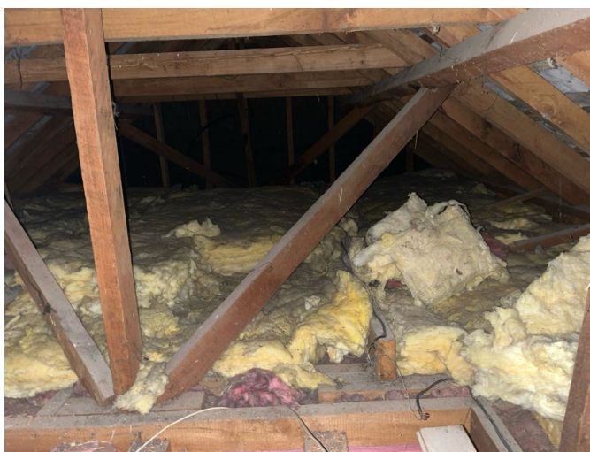
Ceiling areas well covered.
