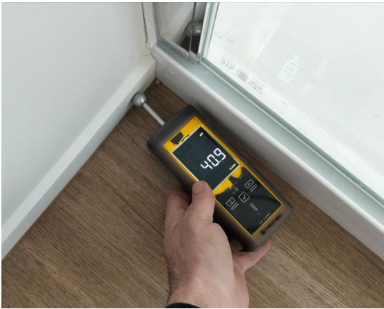
Moisture readings – dry range
