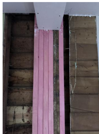
Photograph 14 – New 2/200x90 hySPAN living-area beam installed and wrapped (approx. 180 mm overall width)
