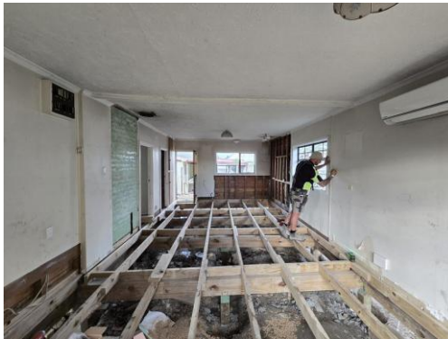
Photograph 1 – view inside house with lifting complete
