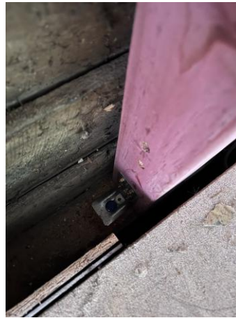
Photograph 18 – Angle-bracket base connection (subfloor) typical throughout
