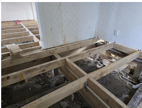
Photograph 7 – internal subfloor framing
