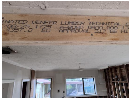
Photograph 12 – New living-area beam: LVL product stamp (A-bond structural laminated veneer lumber)
