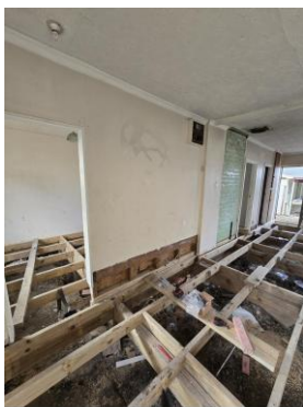
Photograph 3 – view of strengthened floor
