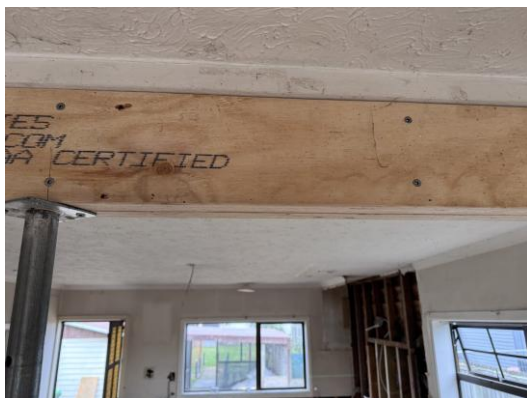
Photograph 13 – New living-area beam: installed directly below the retained original living-area beam (Beam 1 of 2)
