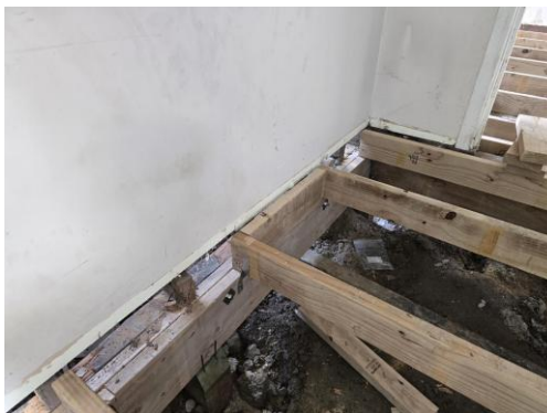
Photograph 5 – perimeter timber framing
