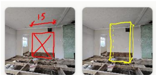
Photograph 19 – Contractor location mark-ups: TV bracing wall (BL1, shown red) and wardrobe lintel (2/190×45 SG8, shown yellow)
