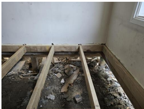
Photograph 6 – joists on new bearers and piles
