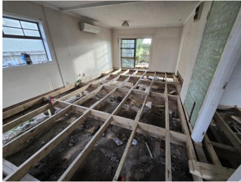
Photograph 10 – view towards front of house
