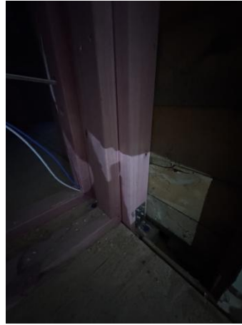
Photograph 16 – Angle-bracket connection at post base
