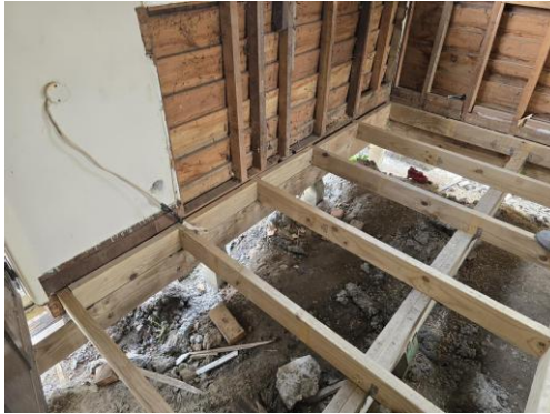
Photograph 9 – new timber subfloor
