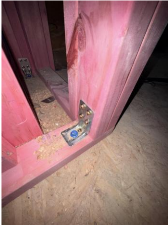
Photograph 15 – Proprietary angle bracket (handibacket) fixing at the beam support in wardrobe area
