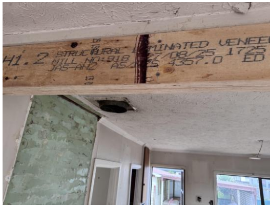
Photograph 11 – New living-area beam: LVL grade stamp confirming H1.2-treated structural laminated veneer lumber to AS/NZS 4357.0 (Mill No. 818)
