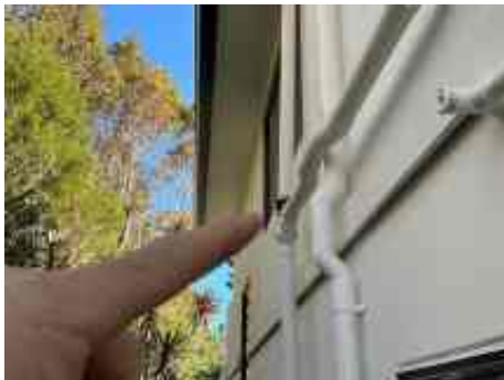
Pipe adjustments and clips required.
