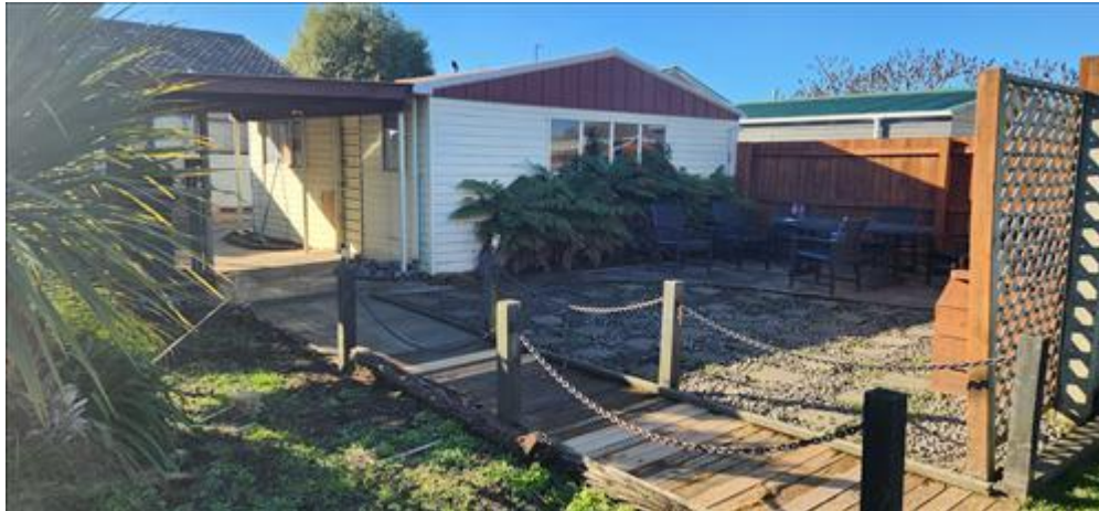
Rear courtyard, garage and carport.
