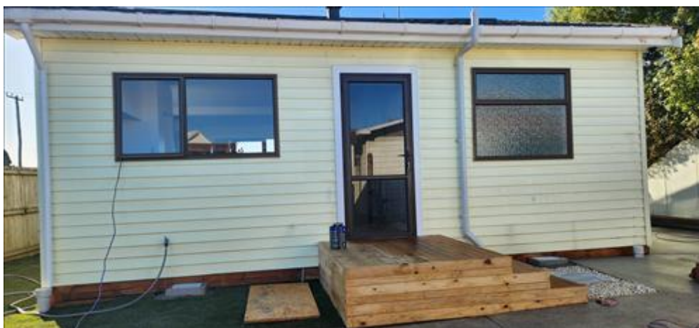
Rear view of the house.
