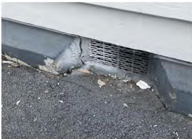
Figure 6 Sample of new foundation cracks
