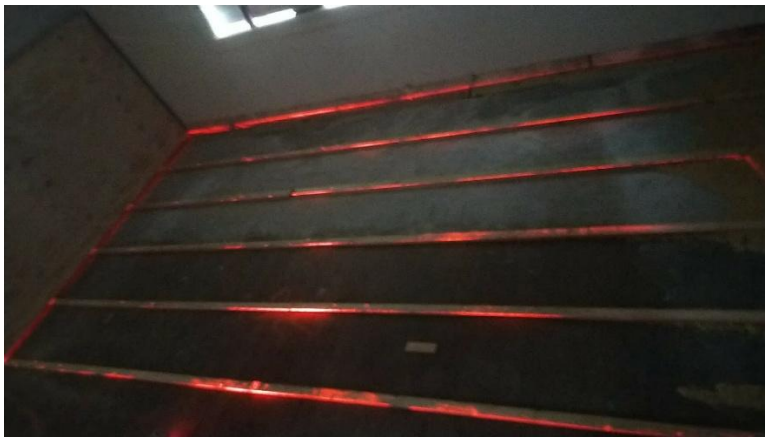
Laser over floor to demonstrate level
