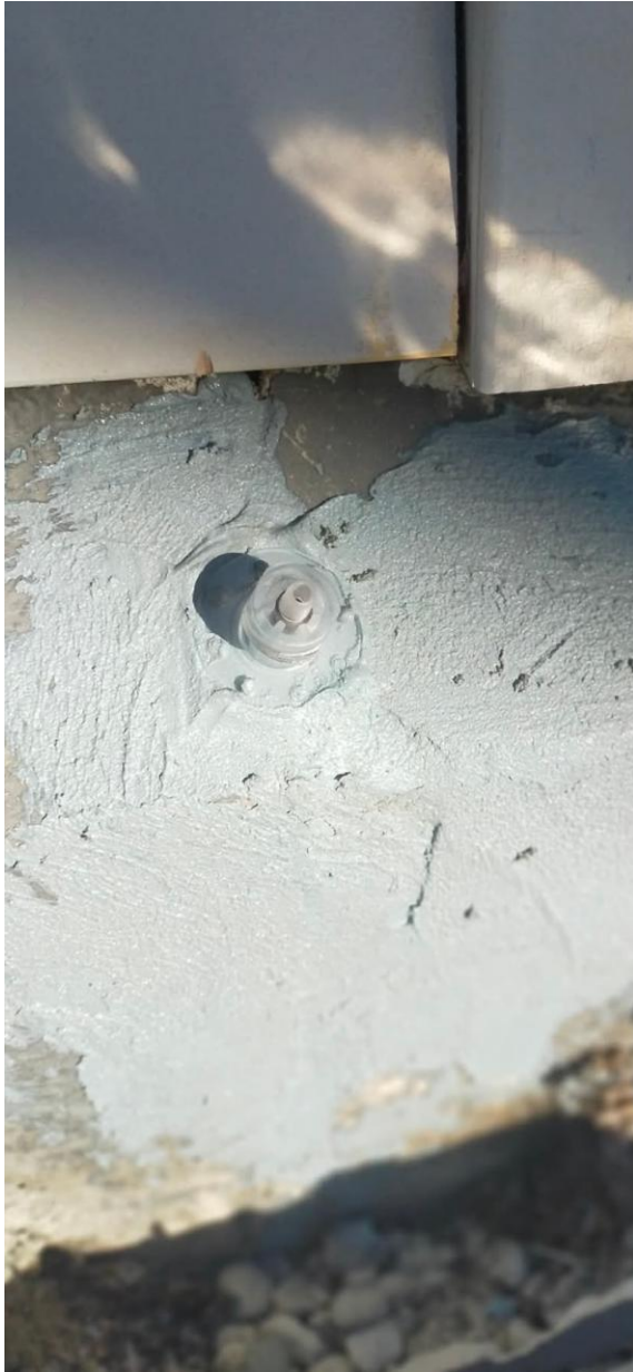
Nipple for epoxy injection (cracks to ring beam)
