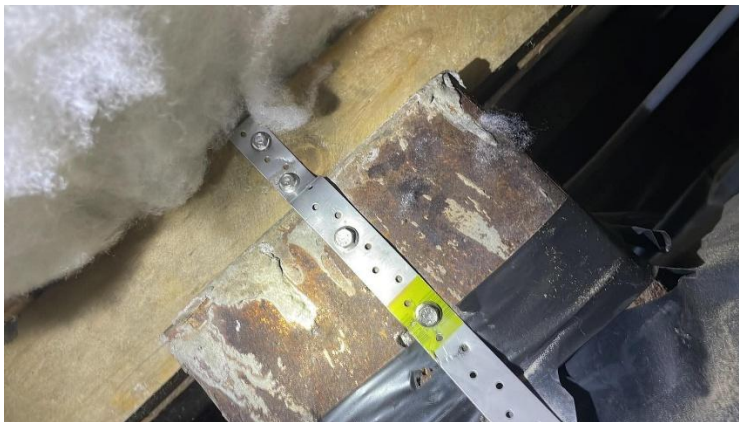
Stainless steel strap to existing "kerosene tin" Pile typical of age of house
