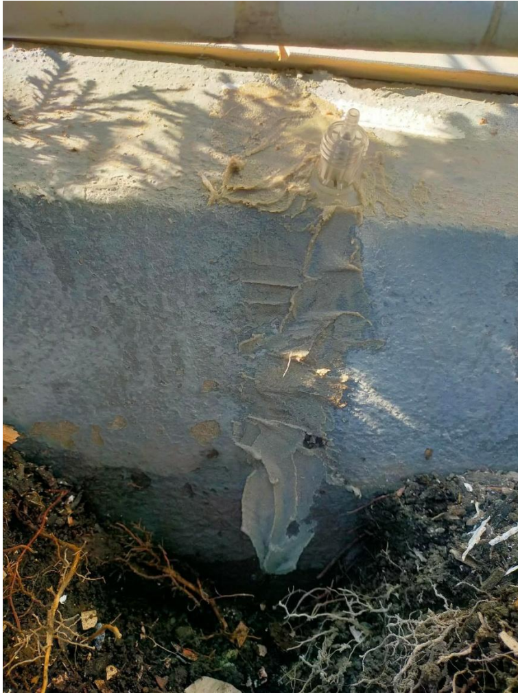
Epoxy Repair to ring beam crack
