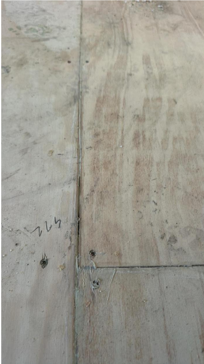
Sealed floor – minor gaps in floor sheet sealed.
