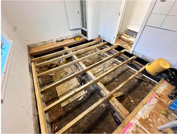
Typical under floor
