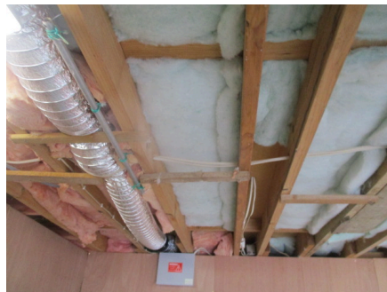
insulation noted to garage ceilings
