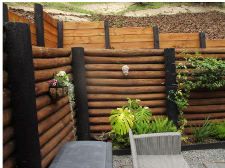
various timber retaining walls
