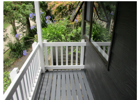
verandah at front
