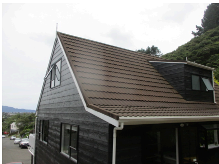
exterior painting completed
