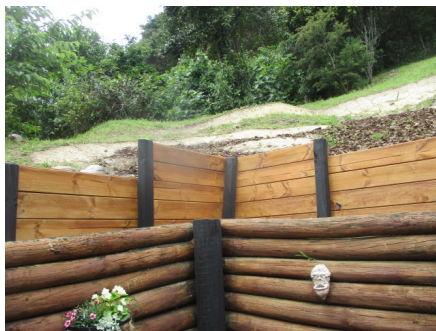
extensive retaining walls done at rear to a good standard
