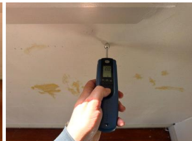
Dry reading around joinery
