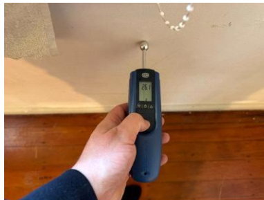
Dry reading around joinery
