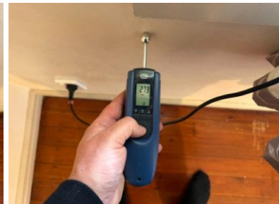
Dry reading around joinery
