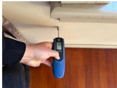
Dry reading around joinery
