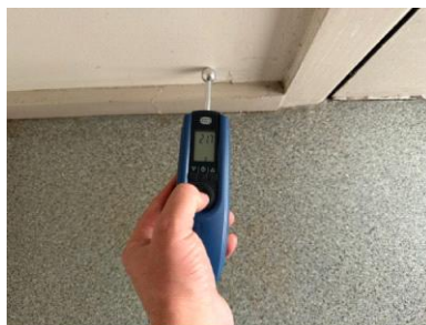
Dry reading around joinery
