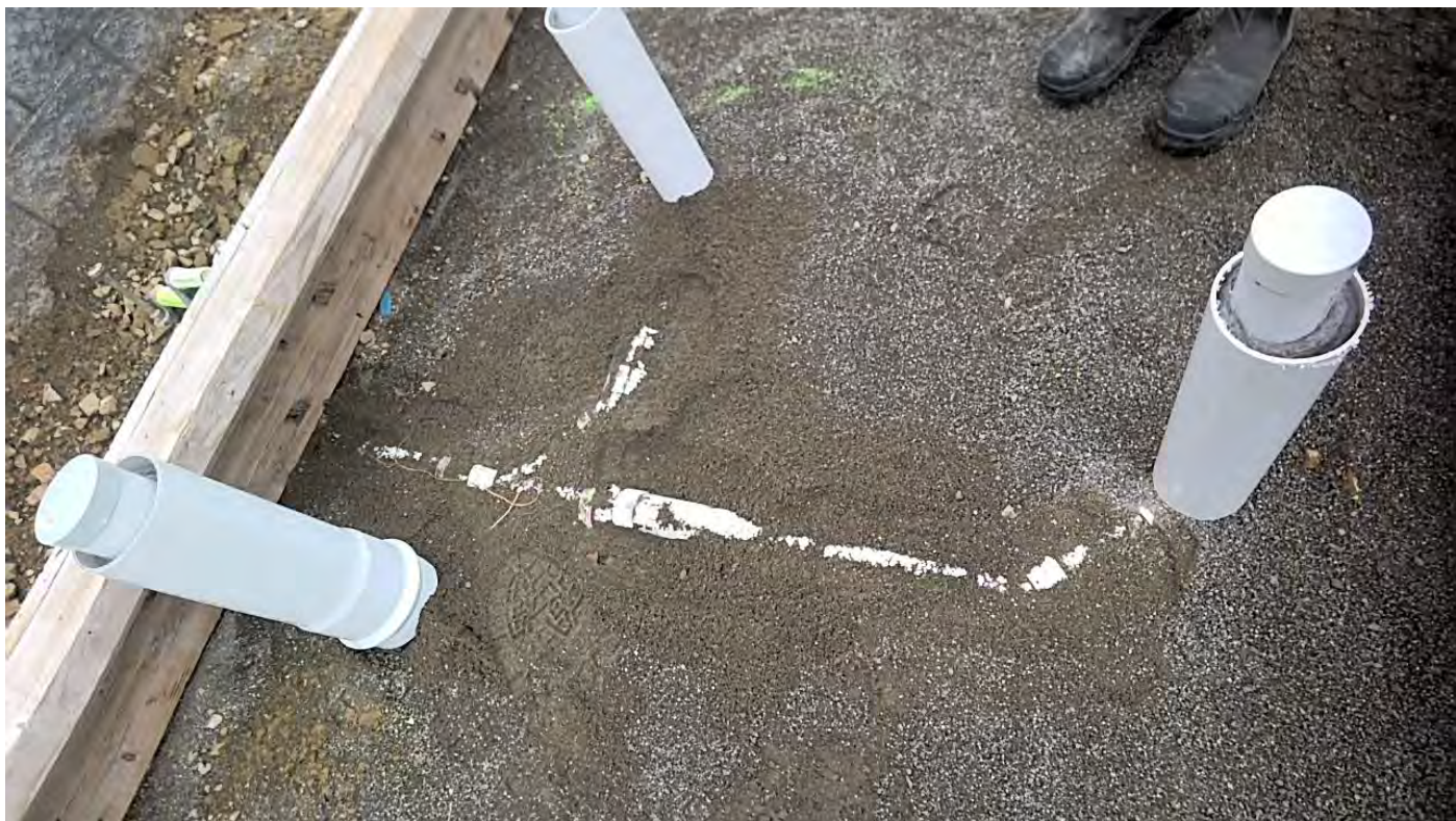
65DN services reduced to 100DN before wc, soffits maintained Taken at 12:18 PM on Wednesday 29/11/2023
