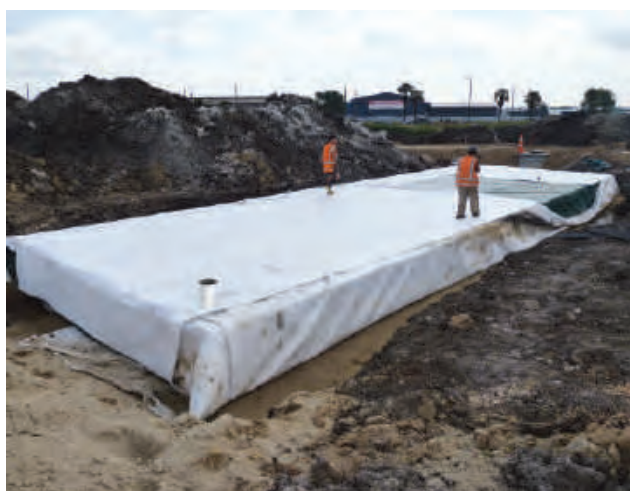
Fig. 16 Installed maintenance port
