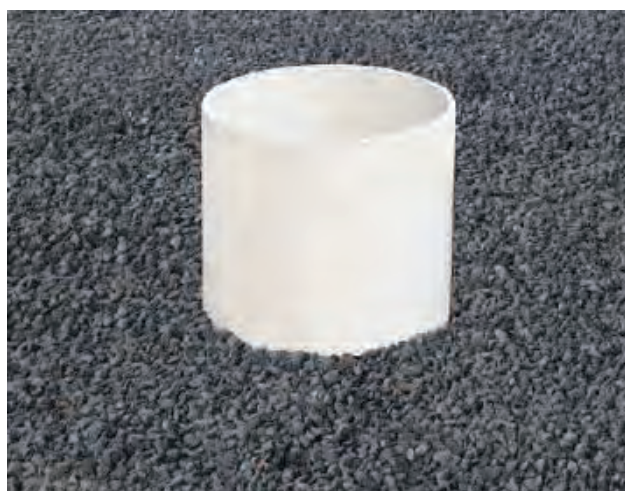
Fig. 17 Install port into RainSmart System
