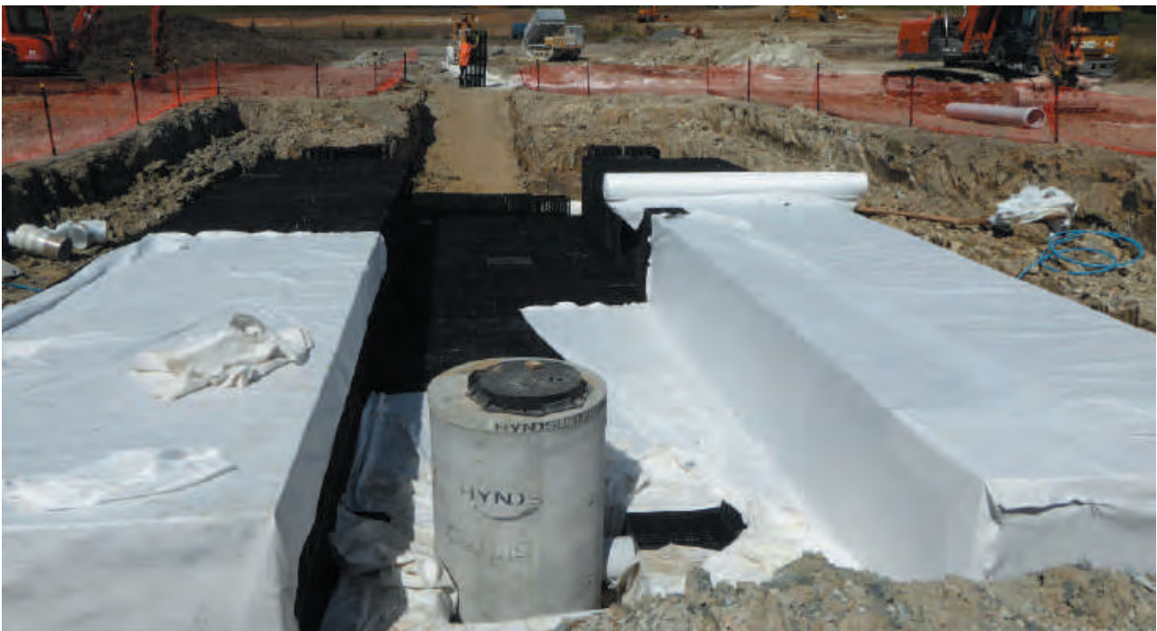
Fig. 18 Encapsulate RainSmart system with geotextile
