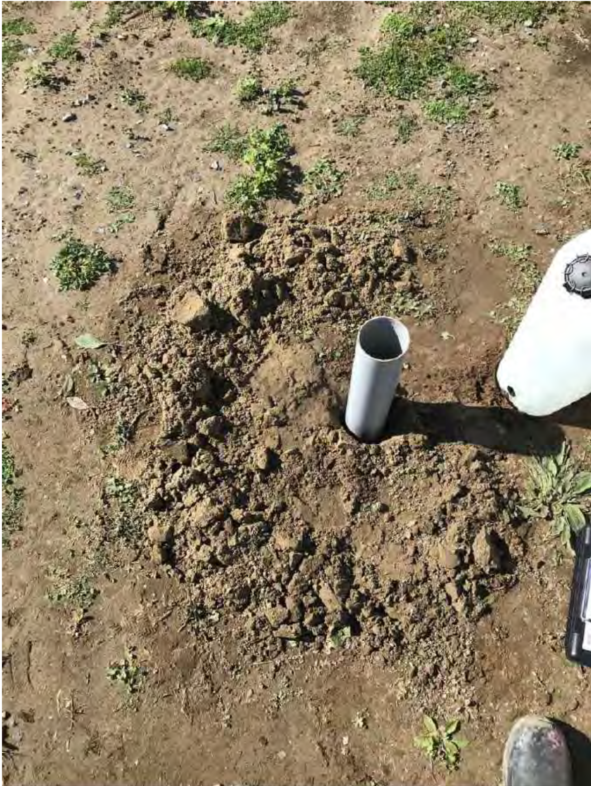
Above: 14 April 2023 – Augered hole at test location – well compacted sand material encountered.
