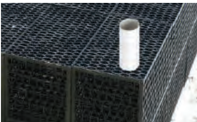
Fig. 11 Installed inspection port.
