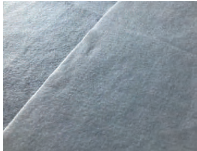
Fig. 7 Overlap geotextile by a minimum of 300mm
