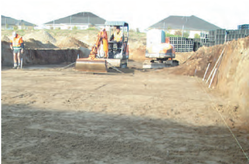
Fig. 5 Base must be smooth to ensure modules fit together without gaps.
