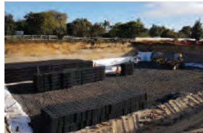
Fig. 4 Preassembled modules can be placed in the excavation or installation can be sped up by assembling the modules in the excavation.
