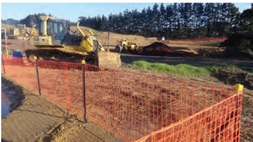
Fig. 25 Secure RainSmart system installation using barriers.
