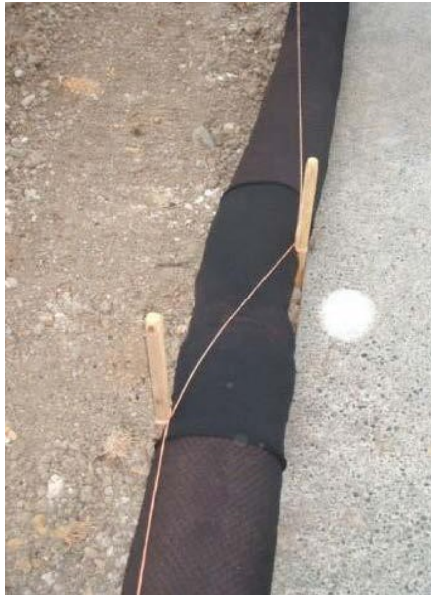
SILT SOCKS: ø225 SILT SOCK FILLED WITH SAWDUST JOINED USING A SLEEVE AND PEGGED AND SECURED USING BAILING TWINE WITH 1m OVERLAPPING JOINT BETWEEN SECTIONS (SEE BELOW)
