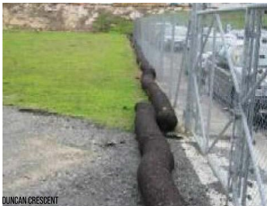
SILT SOCKS: ø225 SILT SOCK FILLED WITH SAWDUST JOINED USING A SLEEVE AND PEGGED AND SECURED USING BAILING TWINE WITH 1m OVERLAPPING JOINT BETWEEN SECTIONS (SEE BELOW)
