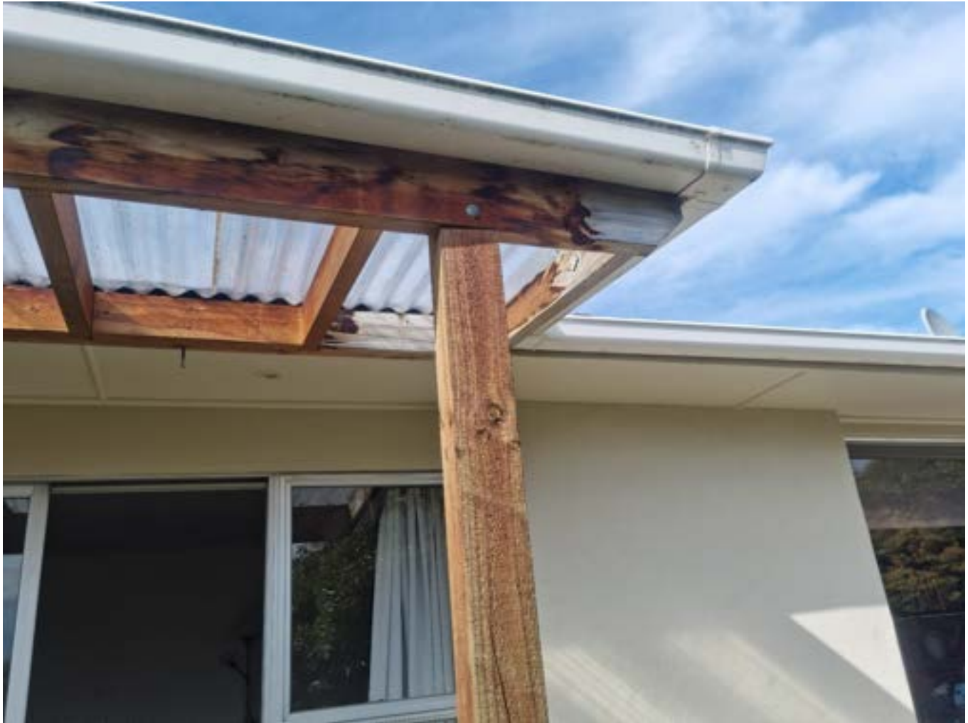
Cantilevered 200 x 50 beam from 100 x 100 post
