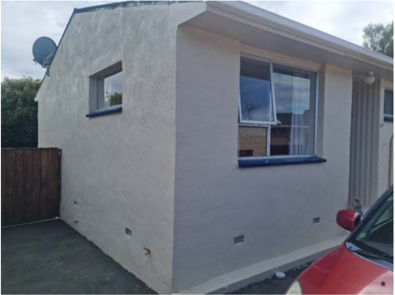
Sub-floor vents to bedroom beside entry South-West corner
