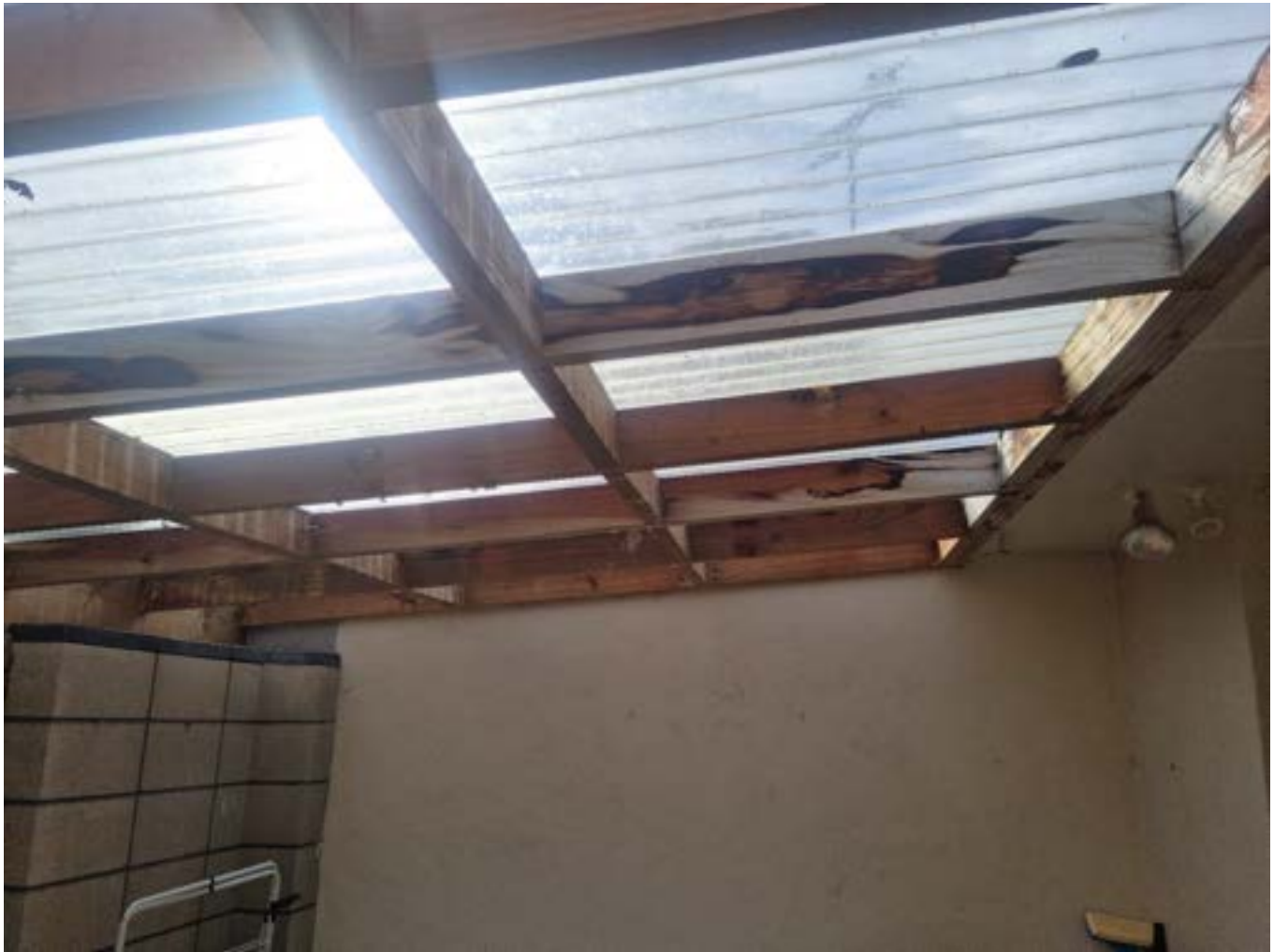
Veranda construction from original fascia over concrete deck with concrete snub wall
