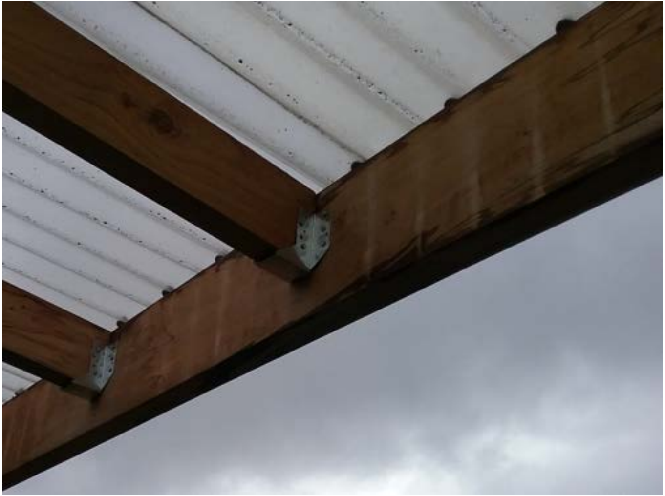
Joist hangers to rafters
