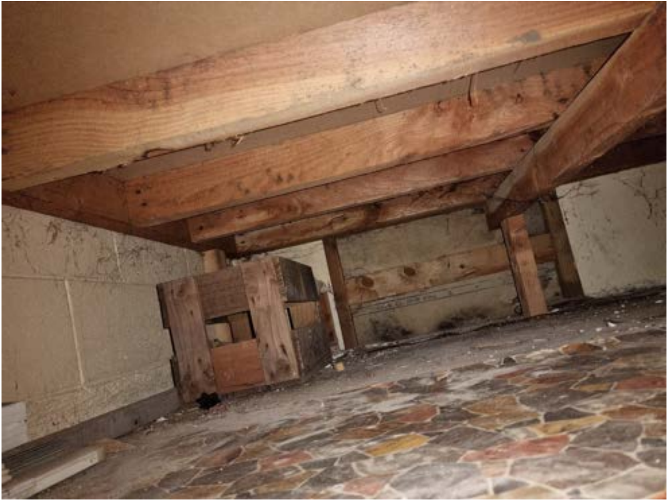
Sub-floor timber framing below laundry
