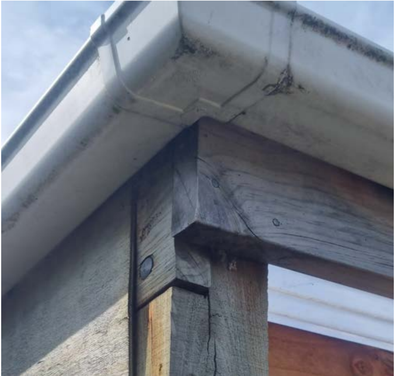
200 x 50 beam fixing to 125 x 125 post
