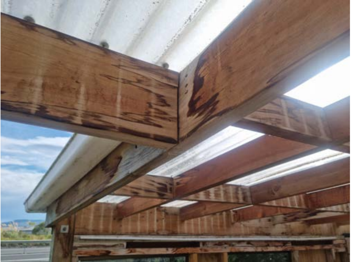
200 x 50 to 250 x 50 beam connection
