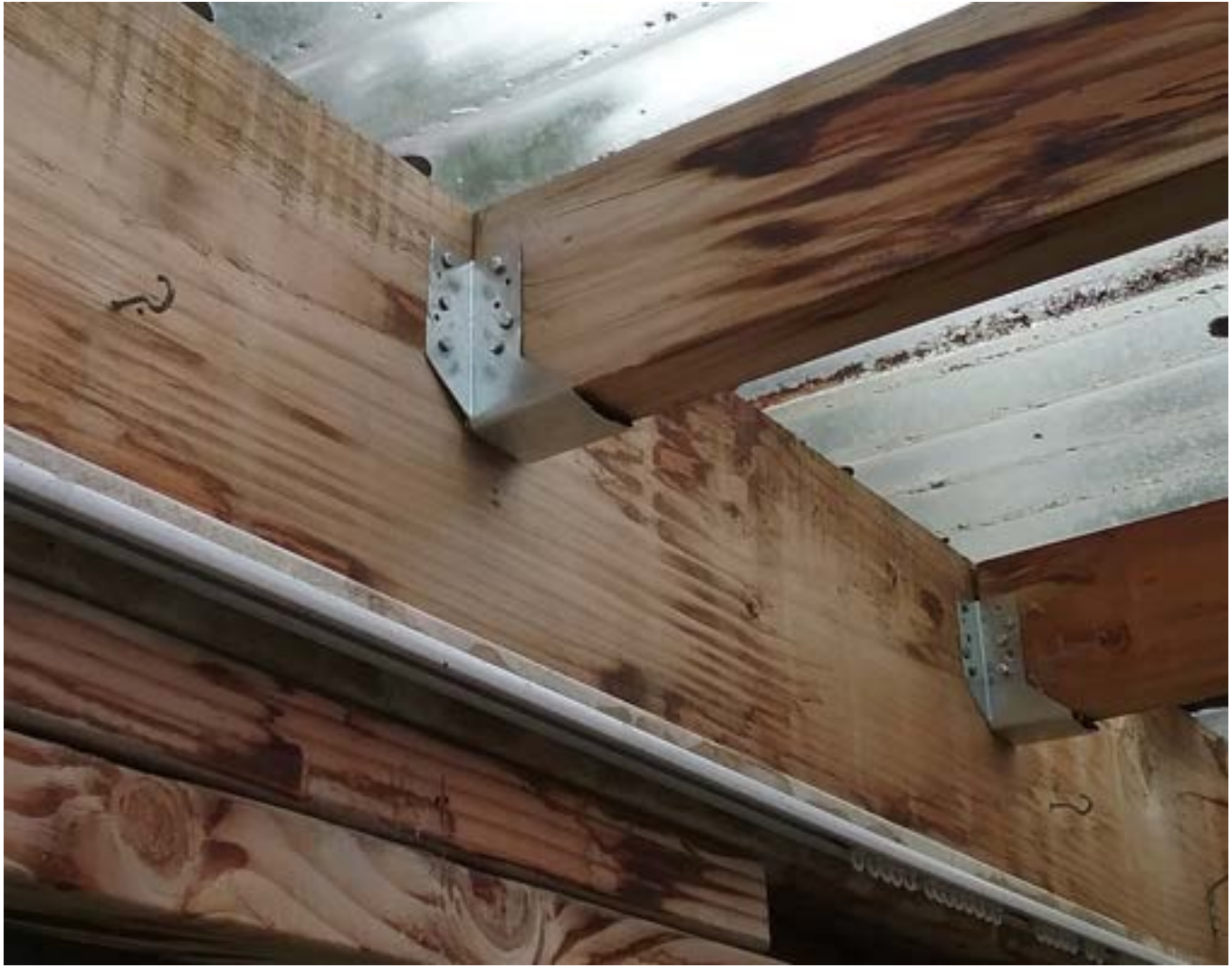
Joist hangers to rafters
