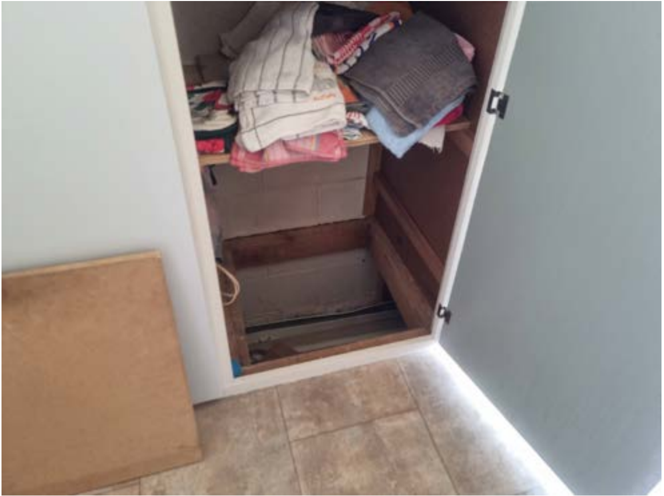
Sub-floor access in laundry cupboard
