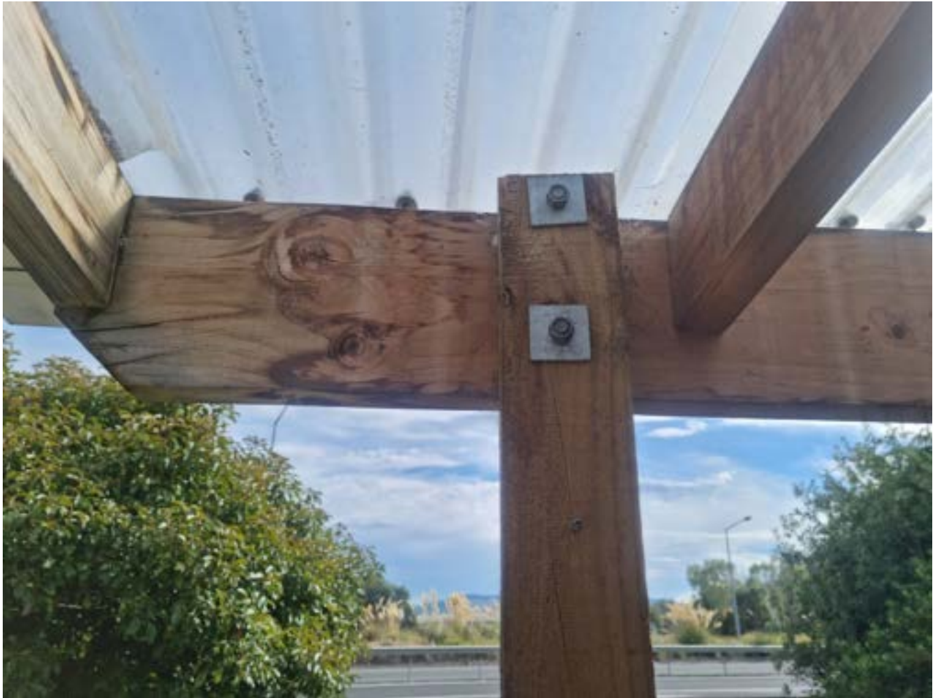
200 x 50 beam fixing to 100 x 100 post
