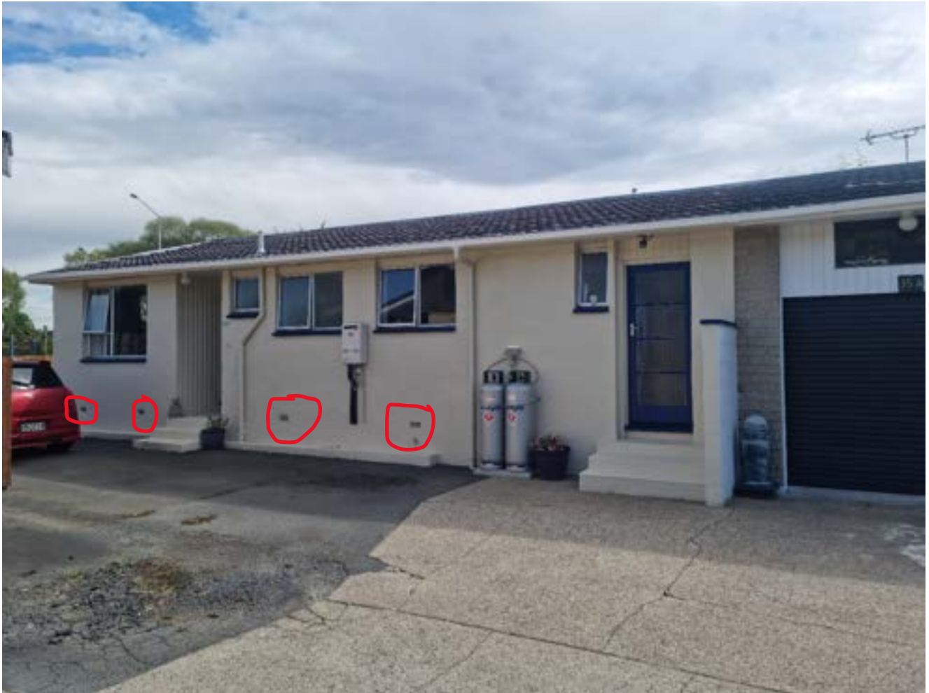
South elevation with no visible signs of alterations except to the garage area (Sub-floor vents circled)
