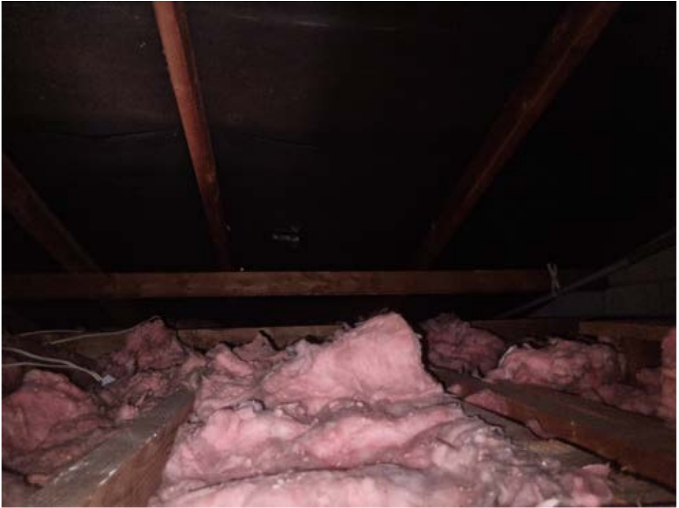
Insulation above converted bedroom
