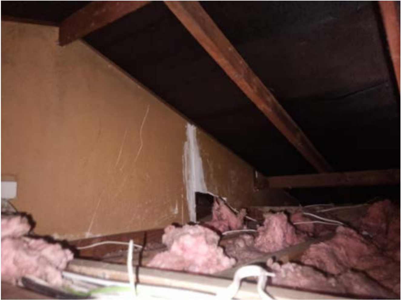
Former fire wall between original garage and lounge
