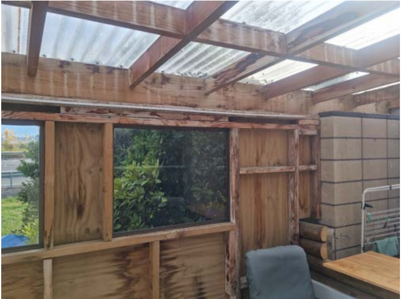
In-filled timber framing with aluminium windows
