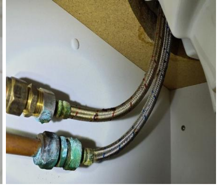
Rust to the flexible hoses under the wash basin
