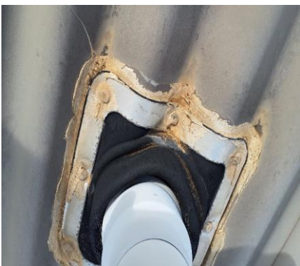
Sealant shows signs of deterioration around vent pipe boot
